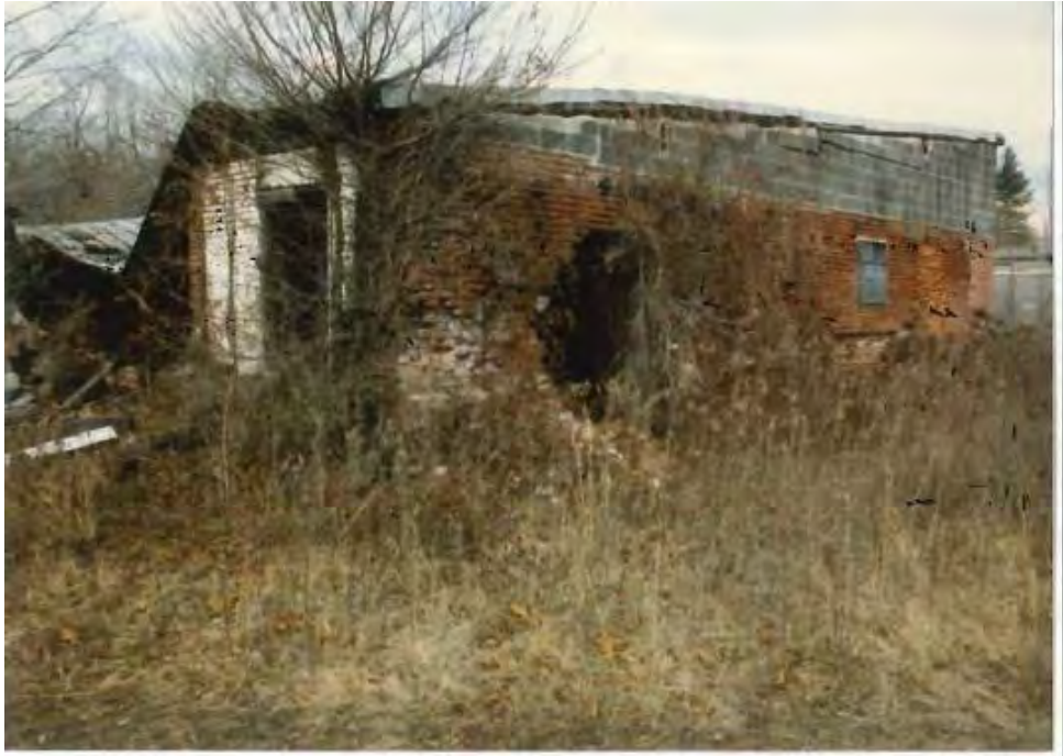
1986 photos of remains of factory buildings
