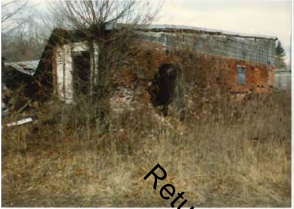
1986 photos of remains of factory buildings
