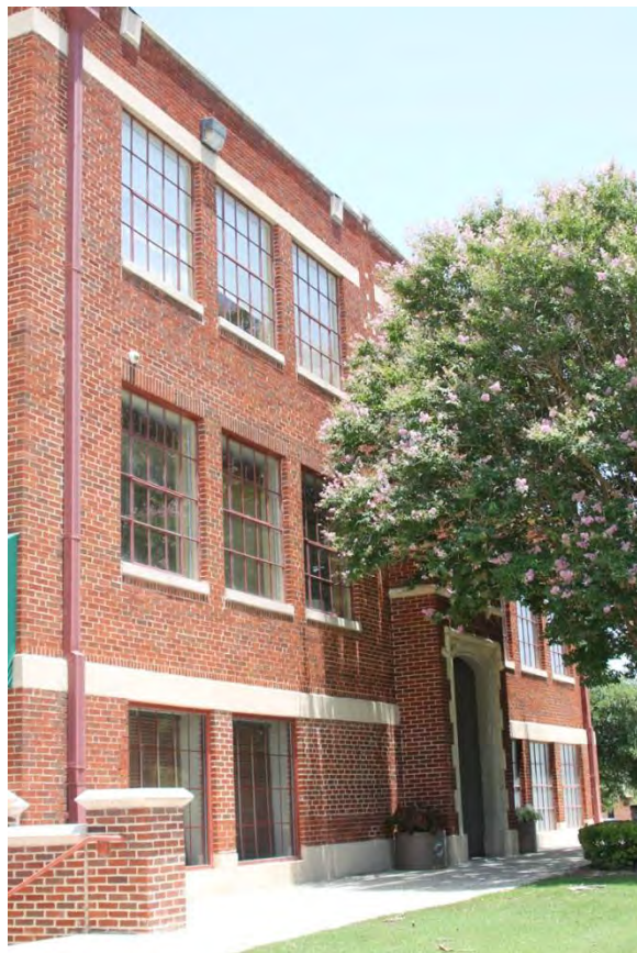
Photo 10 (TX_Bell County_Killeen High School_0010) West elevation, south end Camera facing north
