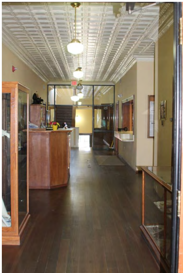
Photo 18 (TX_Bell County_Killeen High School_0018) Interior, second floor corridor Camera facing north
