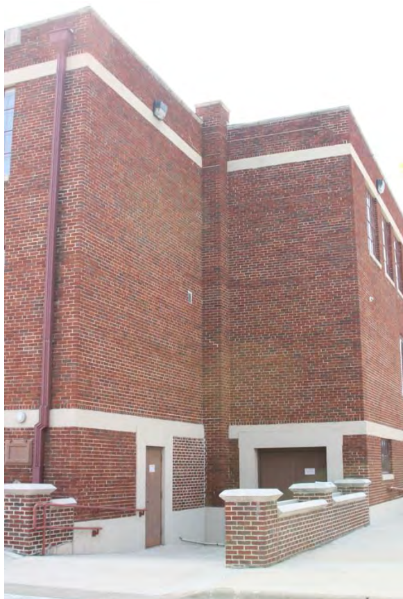
Photo 6 (TX_Bell County_Killeen High School_0006) West elevation, north end Camera facing south
