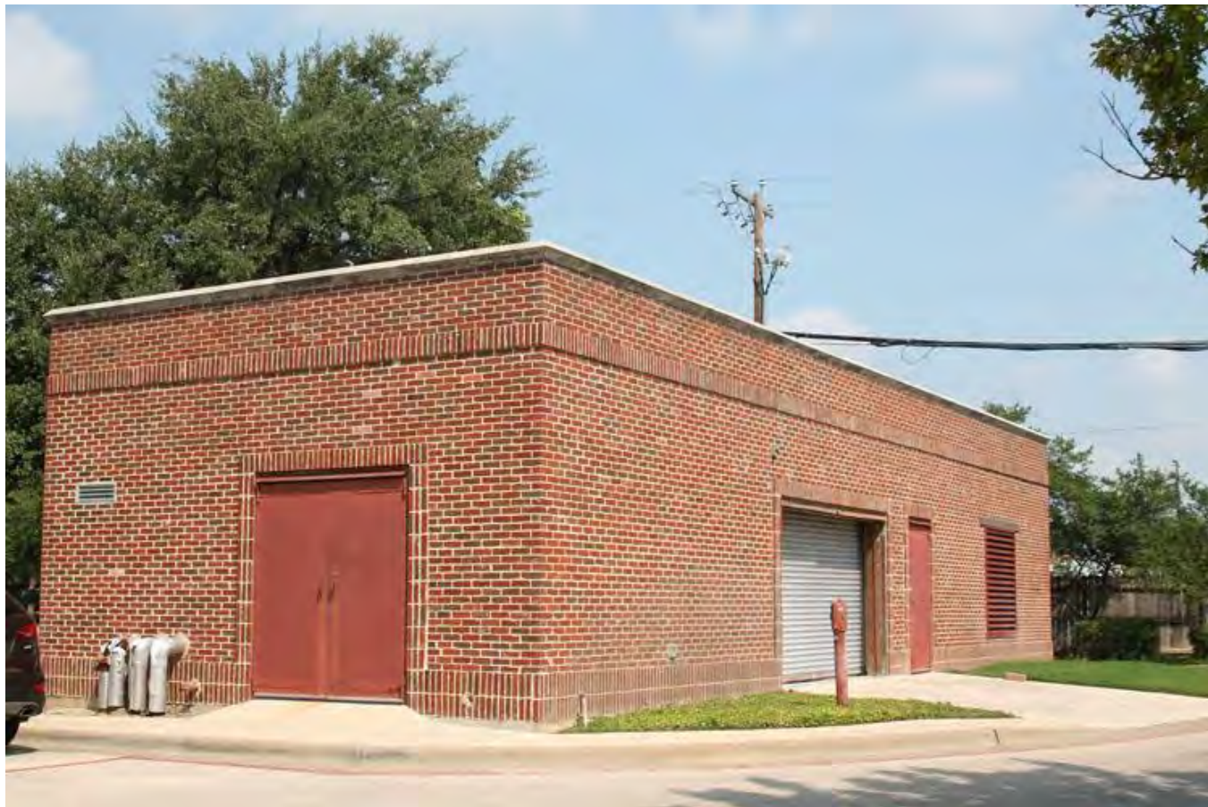
Photo 22 (TX_Bell County_Killeen High School_0022) MEP building (noncontributing) Southeast oblique Camera facing northwest
