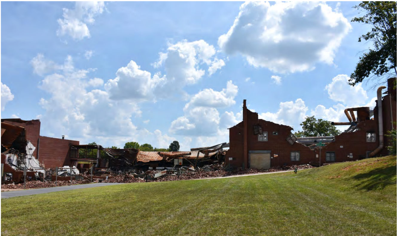
12. Dixie Furniture Company - Lexington Furniture Industries, Ruins of Building Nos. 25-14 to 25-16, South Railroad Street, looking south, September 7, 2018 Demolition commenced in November 2018
