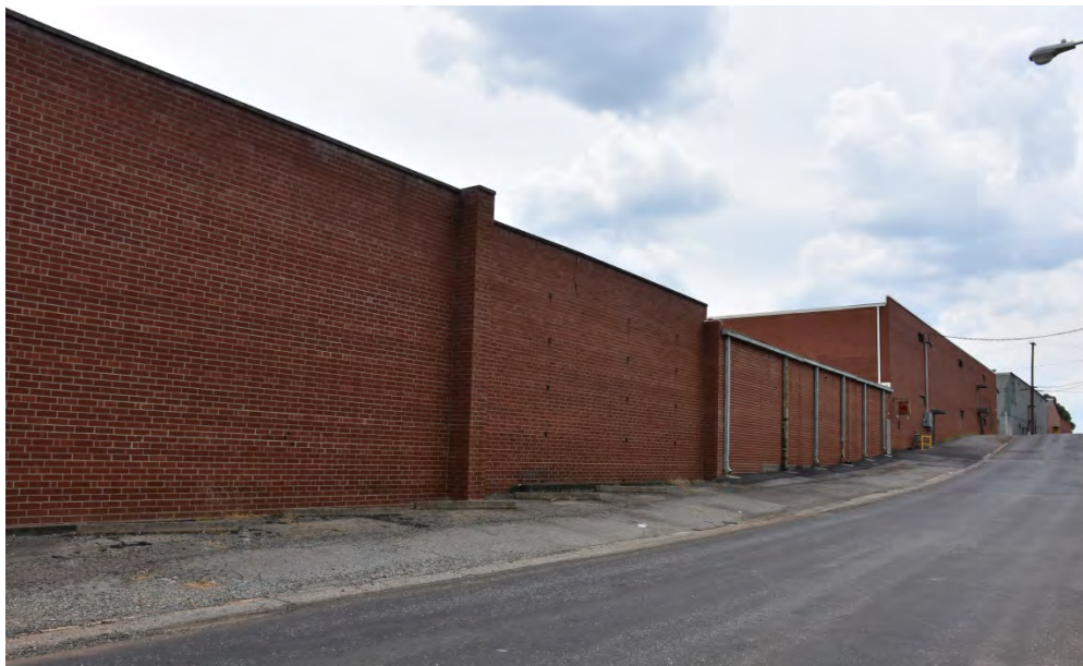
11. Dixie Furniture Company - Lexington Furniture Industries, Building Nos. 25-10 to 25-6, looking southwest (below)
