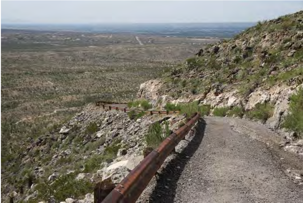
48 of 56. South route (Observatory Road), mid-ascent, photographer facing south. (Not in National Register boundary.)
