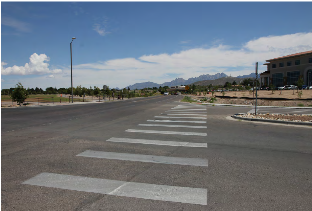
31 of 56. Wells Street, photographer facing northeast. (Not in National Register boundary.)
