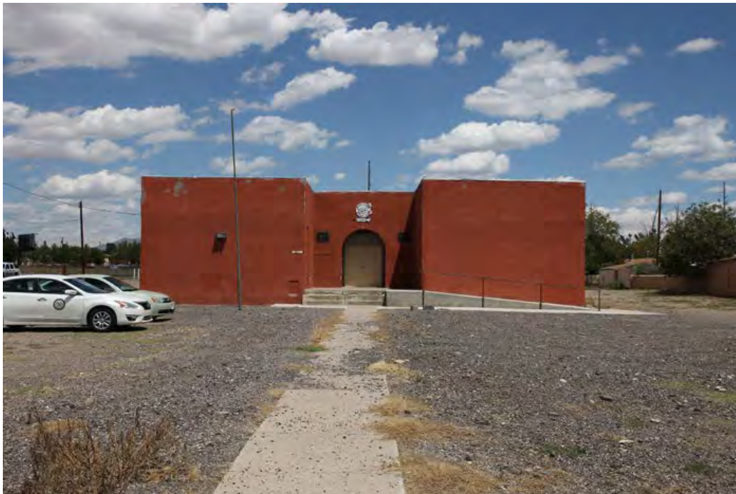
16 of 56. La Escuelita, photographer facing northeast.
