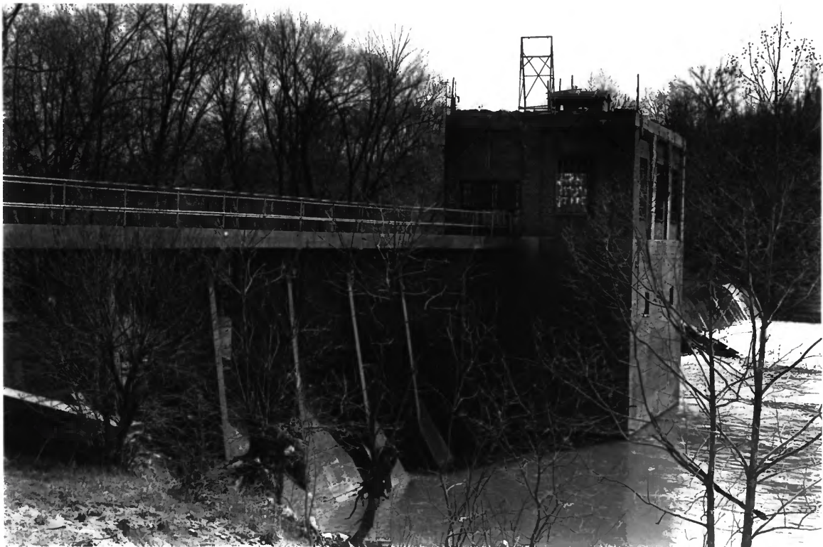
Columbia Hydroelectric Station Columbia, Maury County, TN
