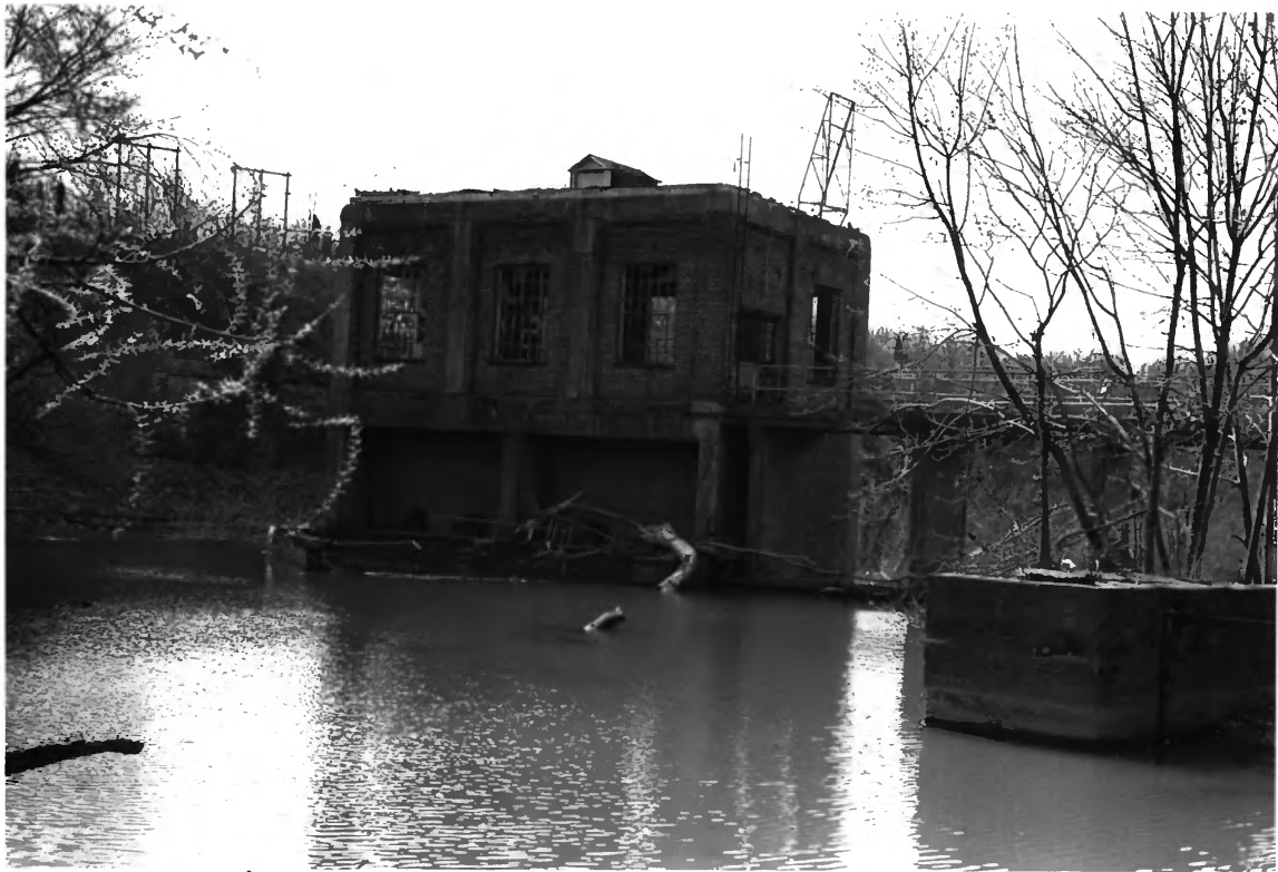
Columbia Hydroelectric Station Columbia, Maury County, TN
