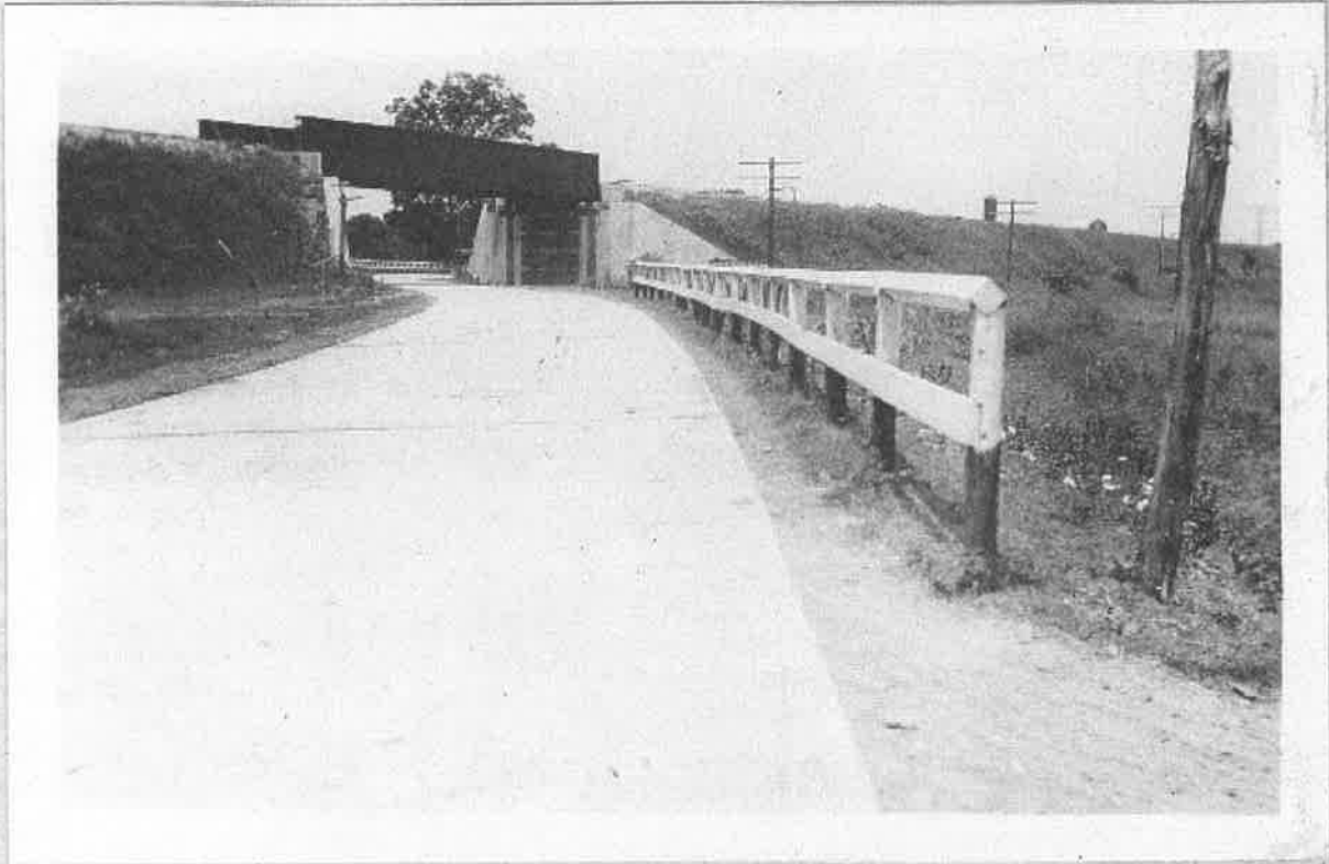
State Highway No. 3, (Southern National) Colorado County. Underpass and concrete roadway east of Columbus, on portion of State Aid section. June 7, 1921.
