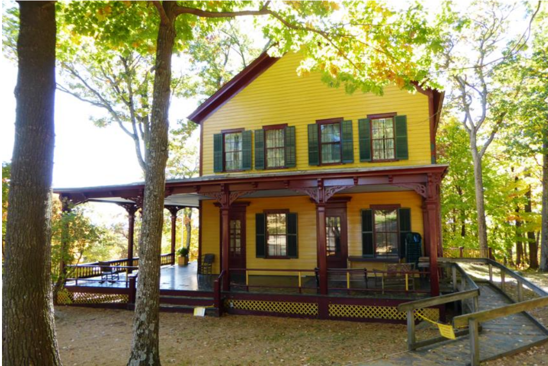
Photo 2: North elevation, view toward southwest.
