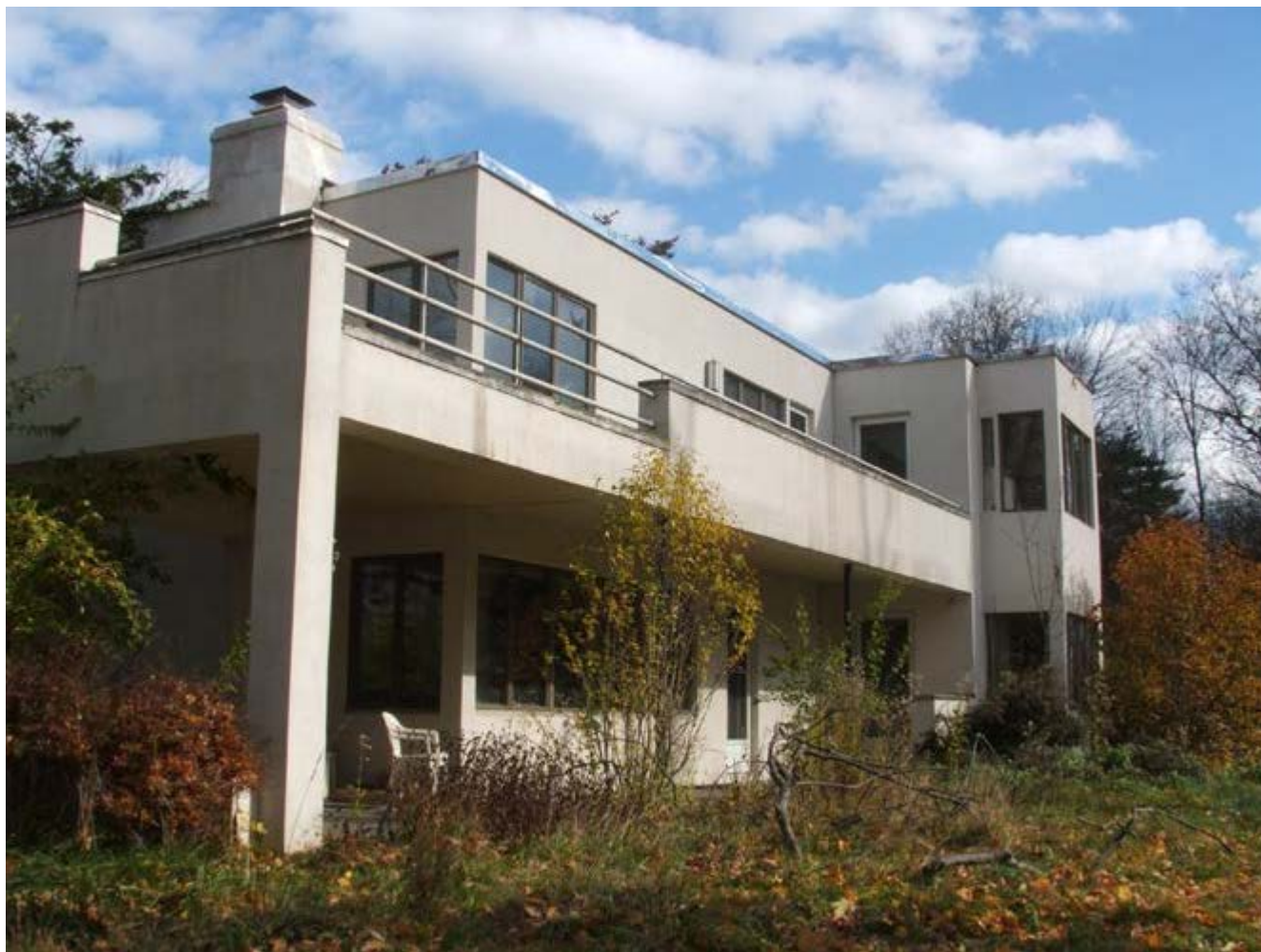
Figure 9: Rauh House rear facade before restoration (2005).
