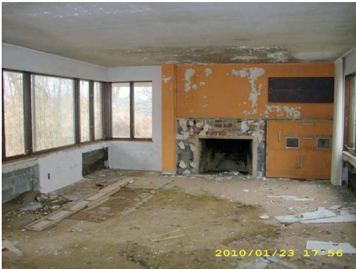
Figure 10: Rauh House living room before Figure restoration (2010).
