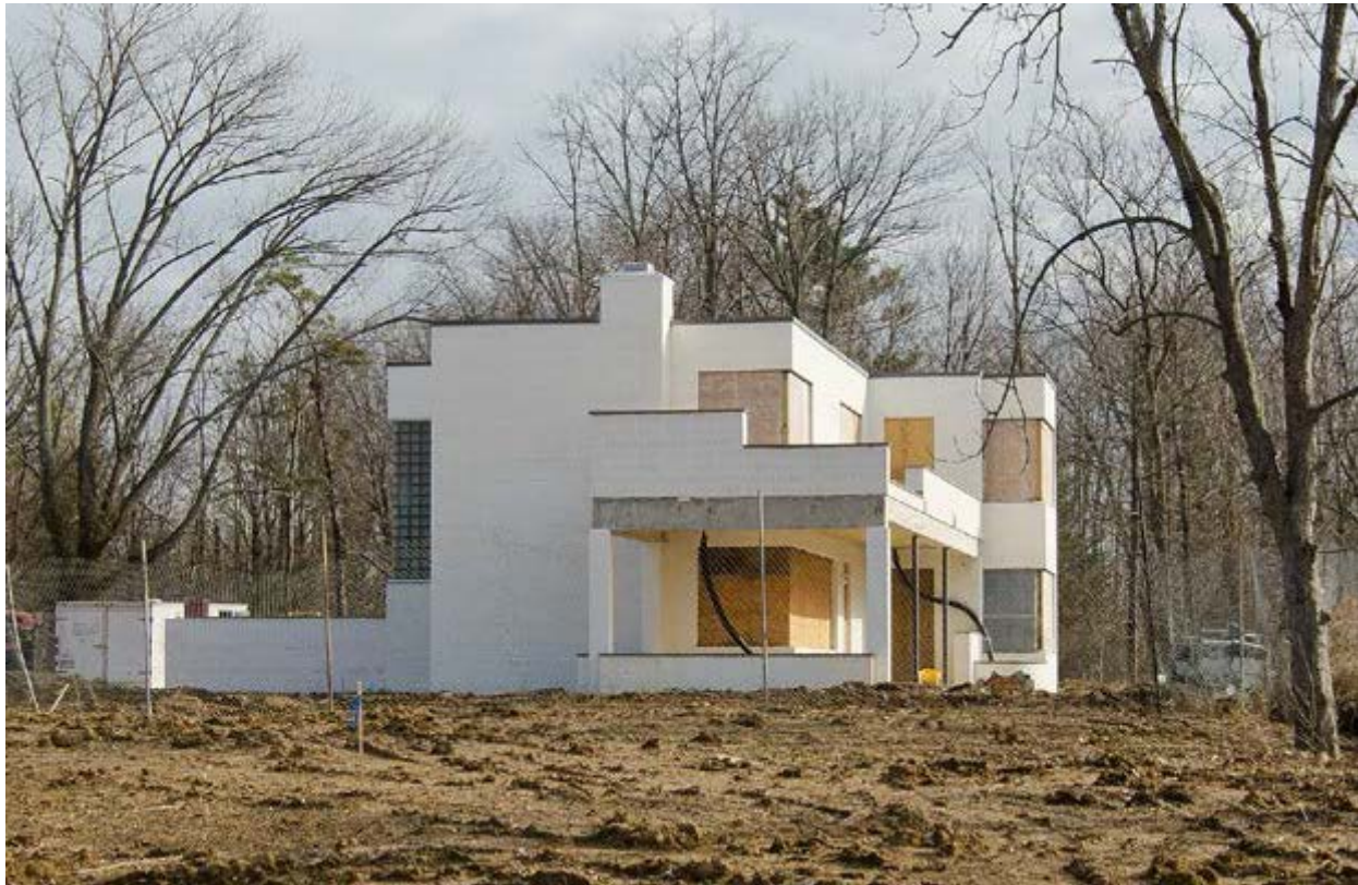
Figure 11: Rauh House west facade during restoration (2012).
