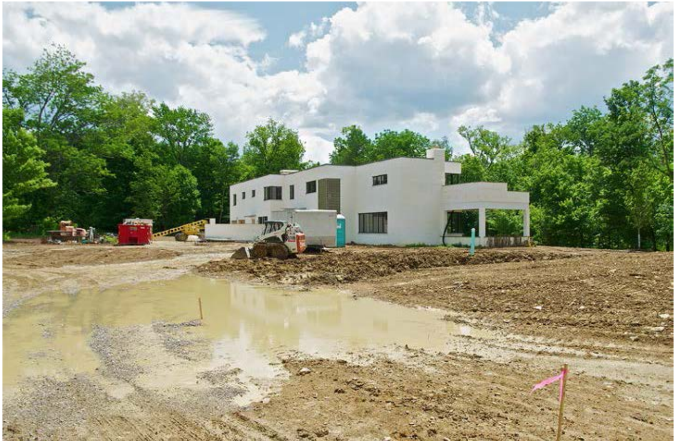
Figure 12: Rauh House during driveway reconstruction (2012).
