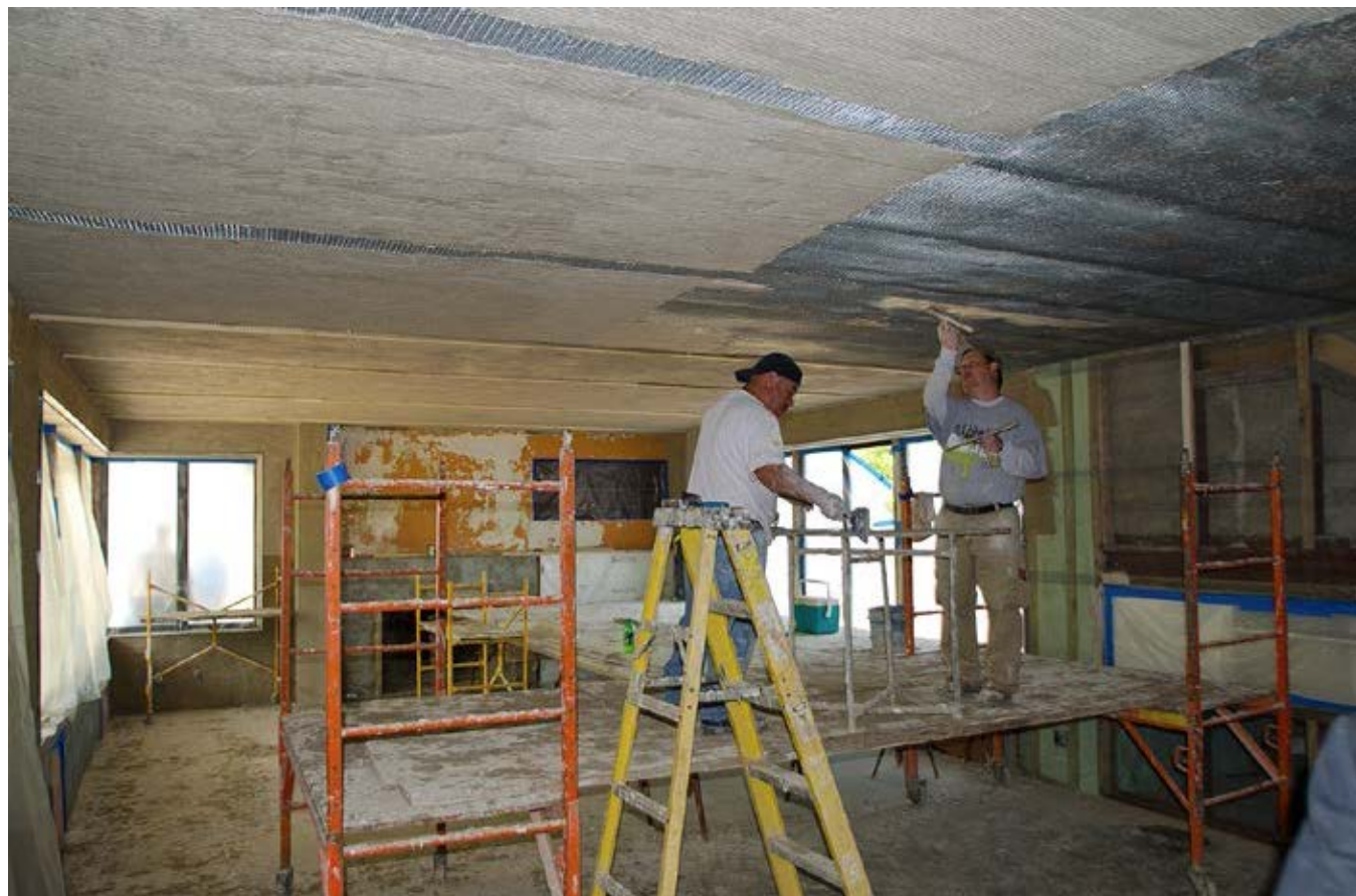
Figure 13: Replastering underway in the Rauh House living room (2012).
