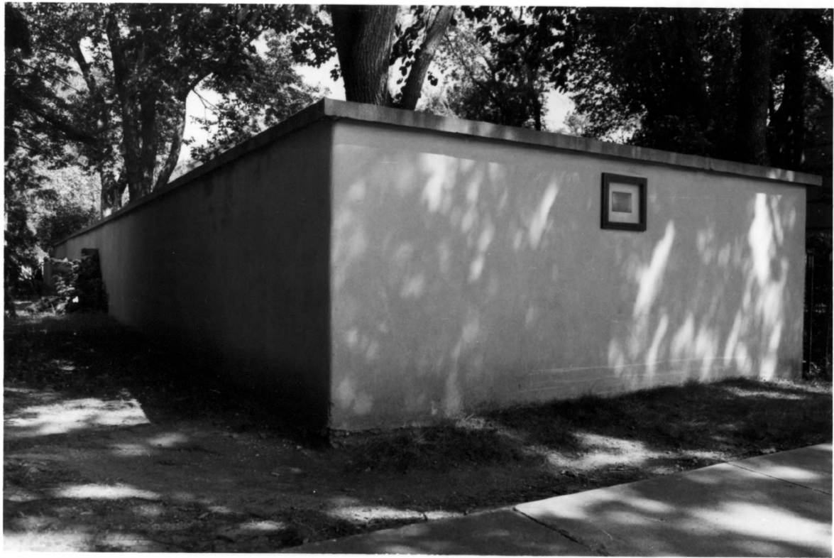
Woodbine Cottage Experimental Rammed Earth Wall, Brookings Co., S. D., No. 1
