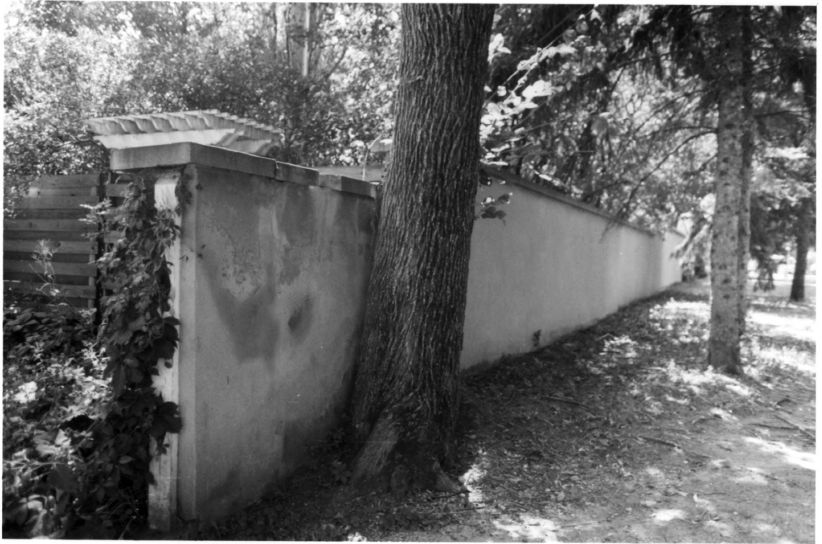
Woodbine Cottage Experimental Rammed Earth Wall, Brookings Co., S. D., No. 2
