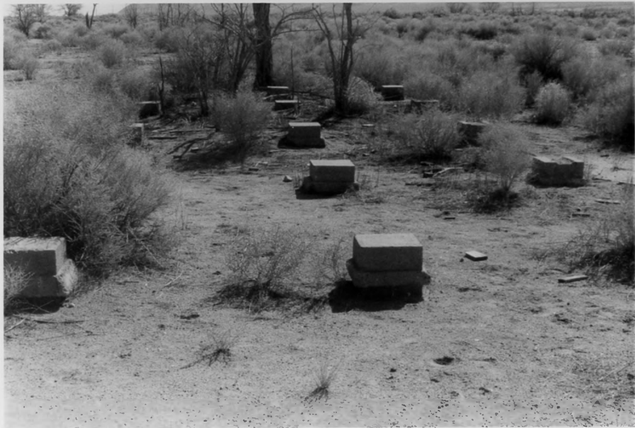
9. Concrete foundation posts slowly weather away in the desert at Manzanar.
