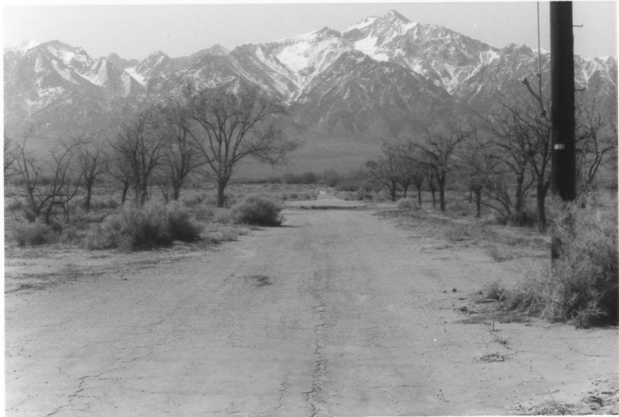
3. Manzanar street separating blocks of barracks. Sierra Nevada in the background.
