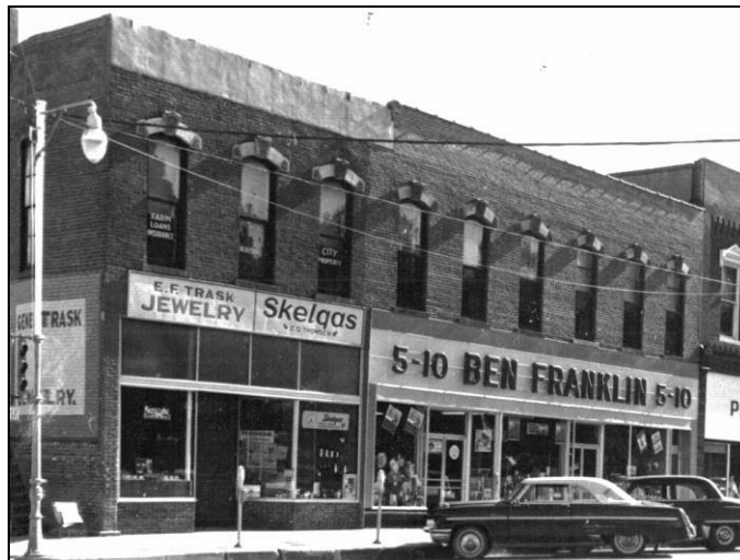
Circa 1950s photograph showing cornice removed and storefronts remodeled. Courtesy: Madison County Historical Society, Winterset
