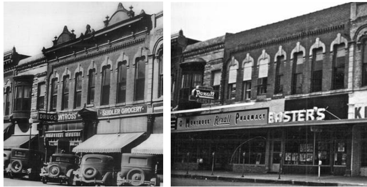
Circa 1948 (left) prior to removal of cornices and circa 1980s (right) showing cornice gone and the storefronts remodeled. Photographs Courtesy: Seidler Family Private Collection (left) and Allen Family Private Collection (right).
