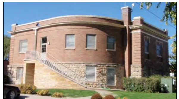
Current view of rear of building showing curved wall.
