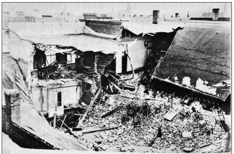
Figure 7. 1896 photograph of the collapsed walls of 68 Court Avenue E and those adjoining caused when the excavation for a basement destabilized the building's stone foundation under T.F. Mardis' supervision, one of several building collapses that occurred under his supervision. Courtesy Allen Family Private Photograph Collection.
