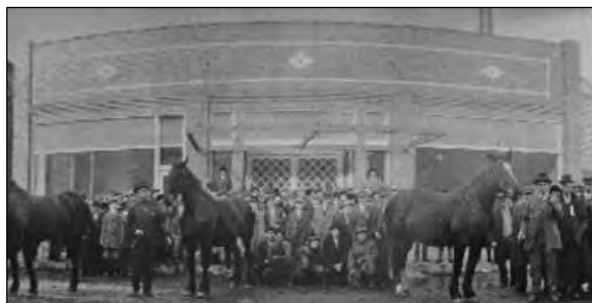
Circa 1926 photograph when building was the Armory. Courtesy: Madison County Historical Society, Winterset.
