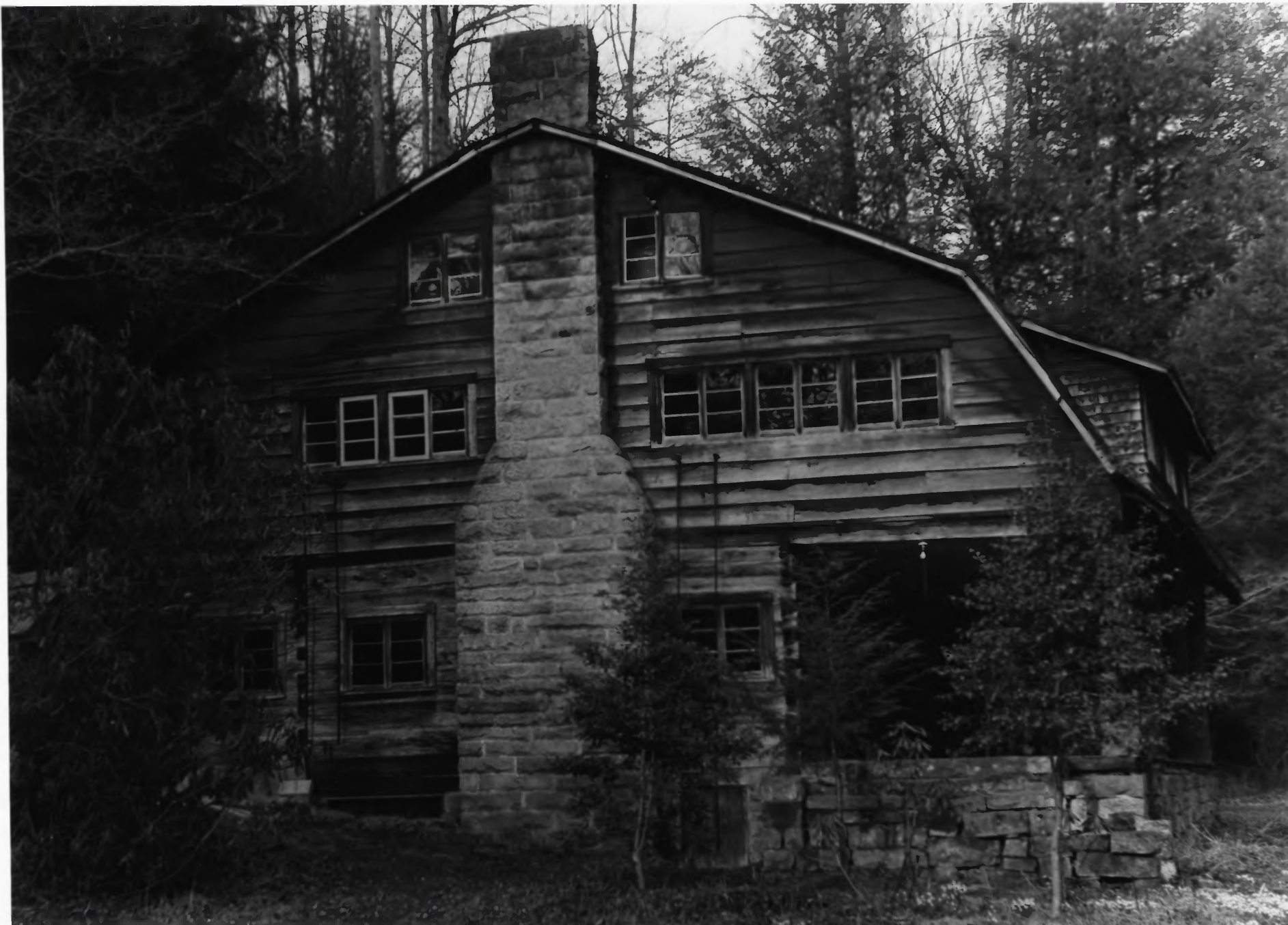
BIG LOG HOUSE, PINE MOUNTAIN SETTLEMENT SCHOOL Harlan County, Kentucky West facade Photo by Chris Jones, February 1990
