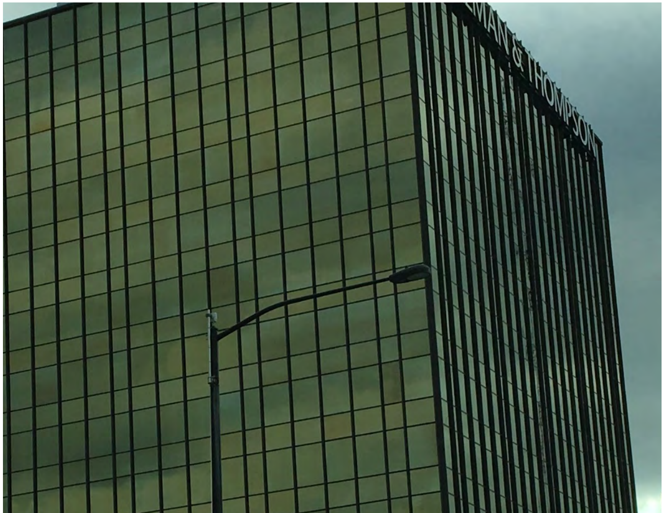
Figure 15. Penntower 3100 Broadway Blvd. Kansas City. Detail of glass curtain wall showing spandrels and profile of vertical mullions. Photo Sophie Roark.
