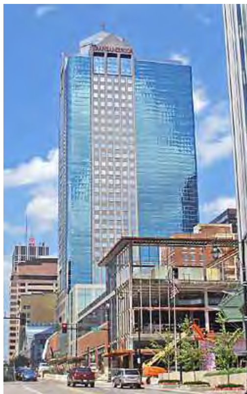
Figure 20. Town Pavilion Tower at 1111 Main Street elevation and plan view Source: Google Map, 2016.
