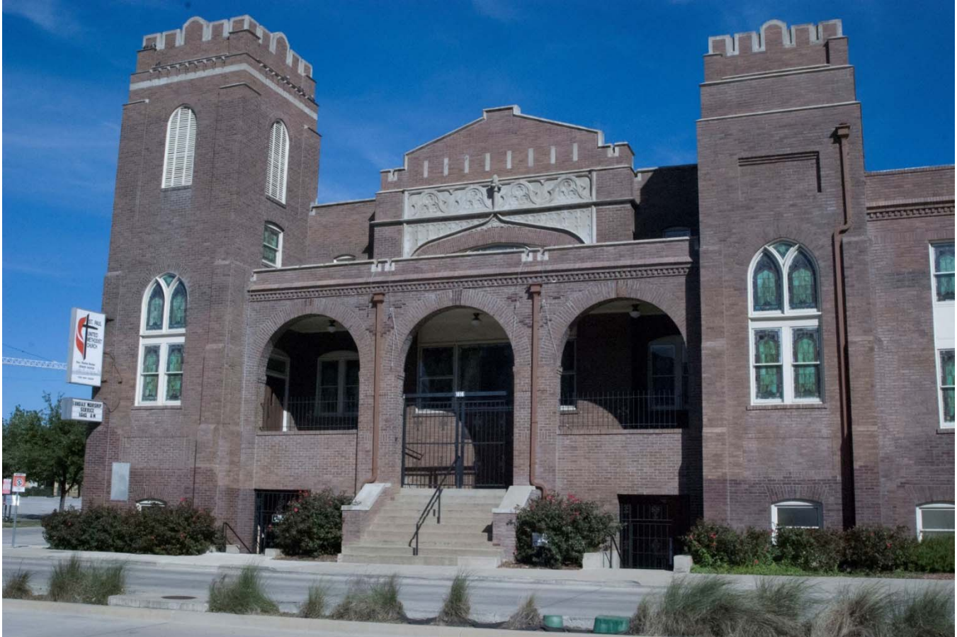
Photo 8: Front (Southwest) Elevation, Detail, Entry Portico, camera facing north.
