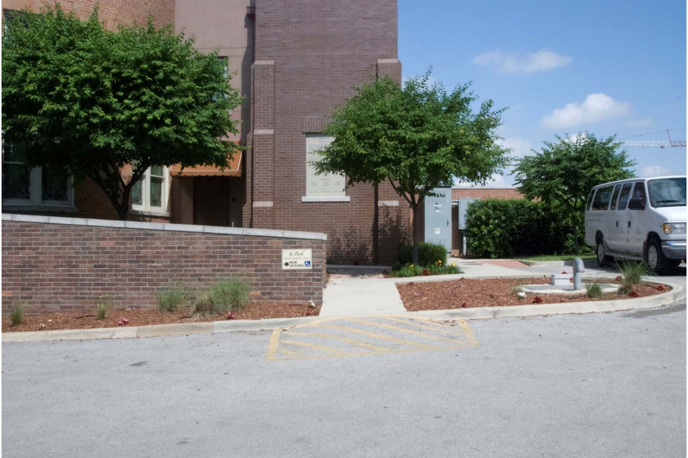
Photo 15: Side (Southeast View, Secondary Entry (Elevator)), camera facing northwest.
