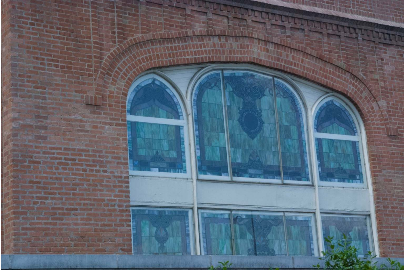
Photo 6: Rear (Northeast) Elevation, Detail, Hood Mold, camera facing northwest.
