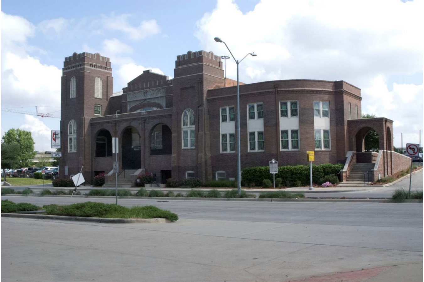
Photo 1: Front (Southwest) and Side (Southeast) Elevations, Oblique, camera facing north.
