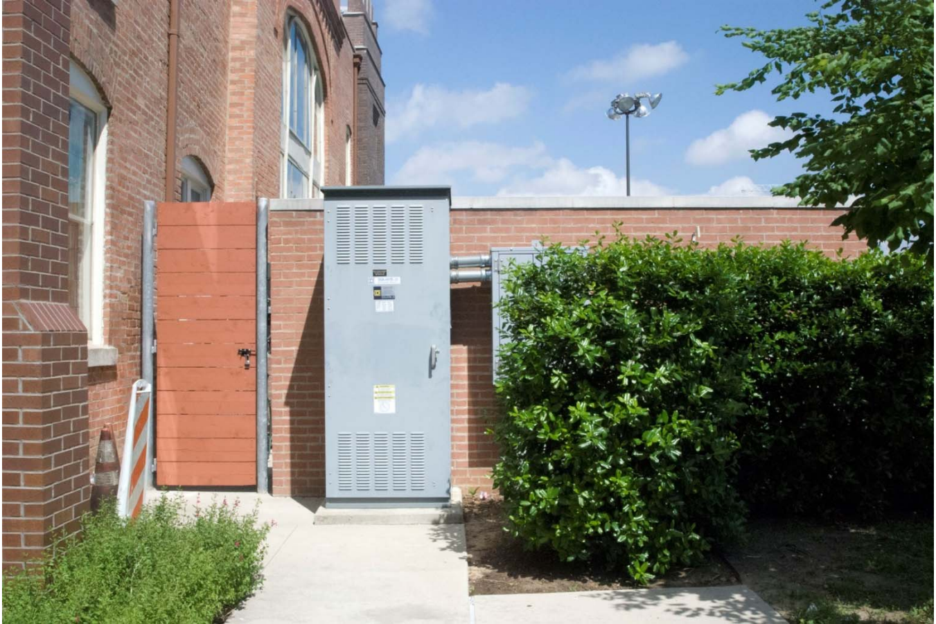
Photo 22: Rear (Northeast) Elevation, Detail, Mechanical Area Entry, camera facing northwest.
