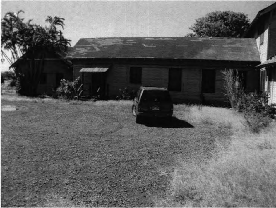
FBMH-006-003. Fred Baldwin Memorial Home, Building 006, Looking Northwest.
