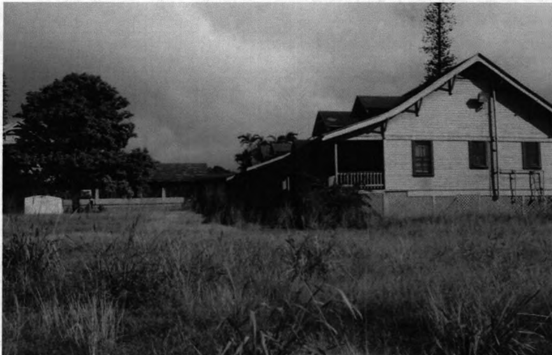
FBMH-S008. Fred Baldwin Memorial Home Site, (left-right) Buildings 005, 006, 007, and 008, Looking East.
