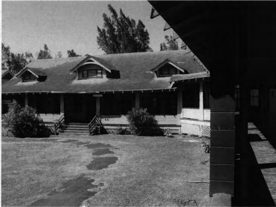
FBMH-002-003. Fred Baldwin Memorial Home, Building 002, Looking Northwest.
