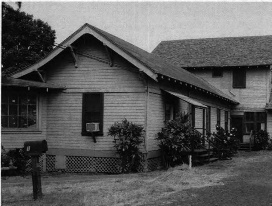
FBMH-006-004. Fred Baldwin Memorial Home, Building 006, Looking Northwest.
