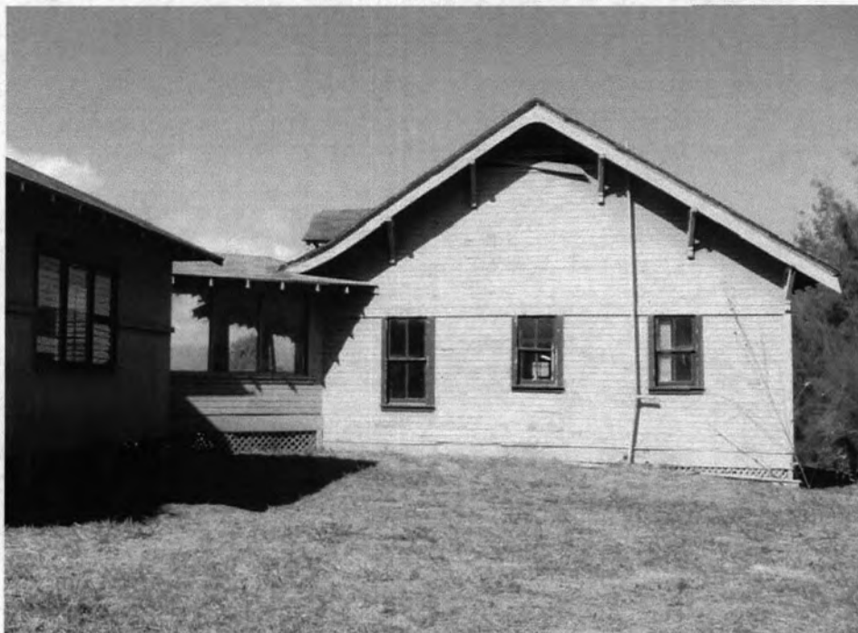
FBMH-002-004. Fred Baldwin Memorial Home, Building 002, Looking Northwest.
