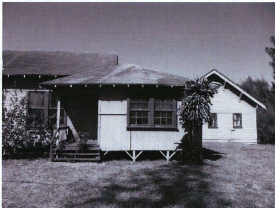
FBMH-004-001. Fred Baldwin Memorial Home, Building 004, Looking Northwest.
