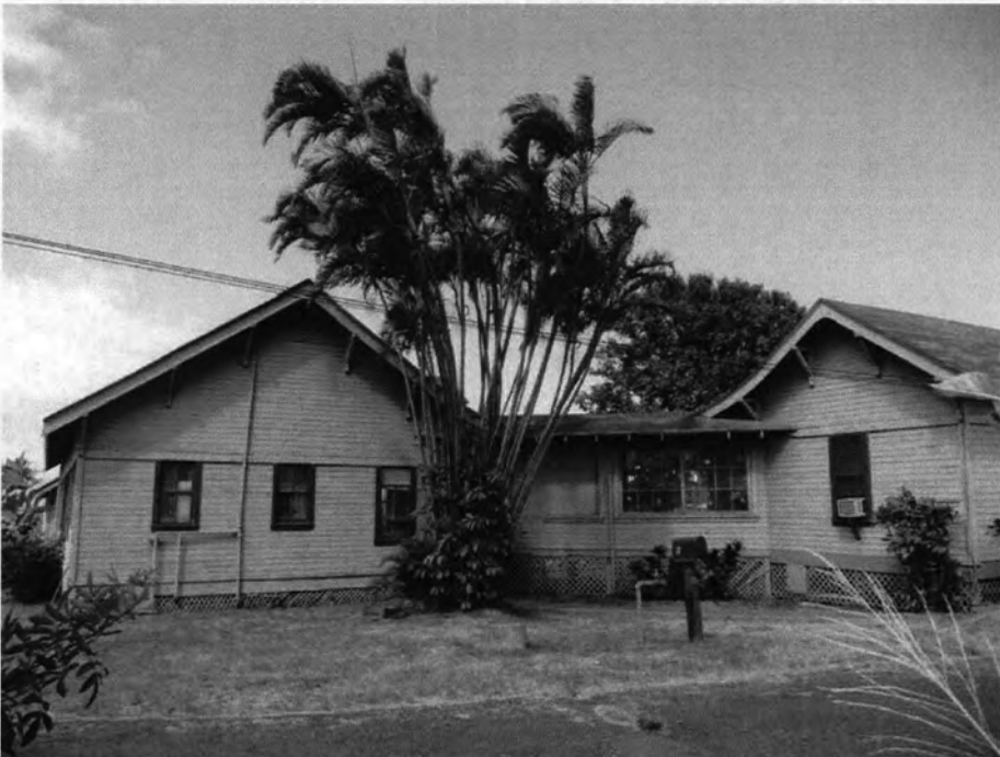
FBMH-007-003. Fred Baldwin Memorial Home, Building 007, Looking Northwest.
