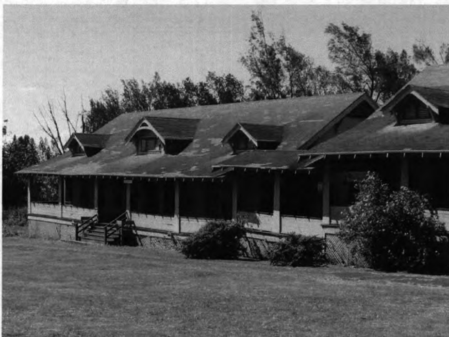
FBMH-001-004. Fred Baldwin Memorial Home, Building 001, Looking Northwest.
