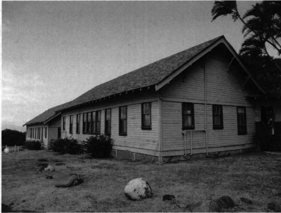
FBMH-007-004. Fred Baldwin Memorial Home, Building 007, Looking Northwest.
