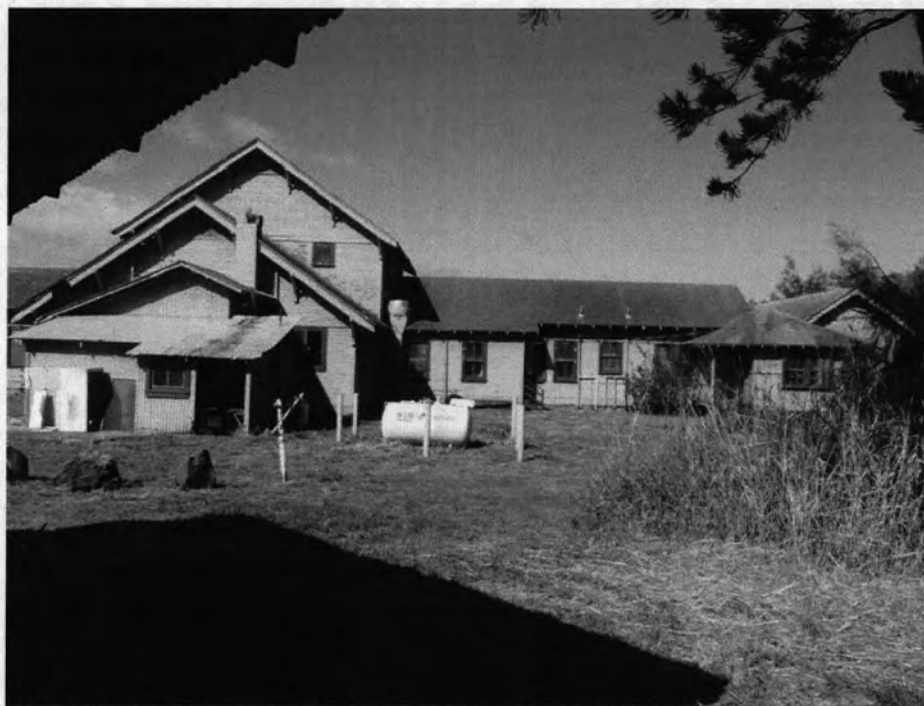
FBMH-S005. Fred Baldwin Memorial Home Site, (left-right) Buildings 005, 003, 004, and 002, Looking Northwest.
