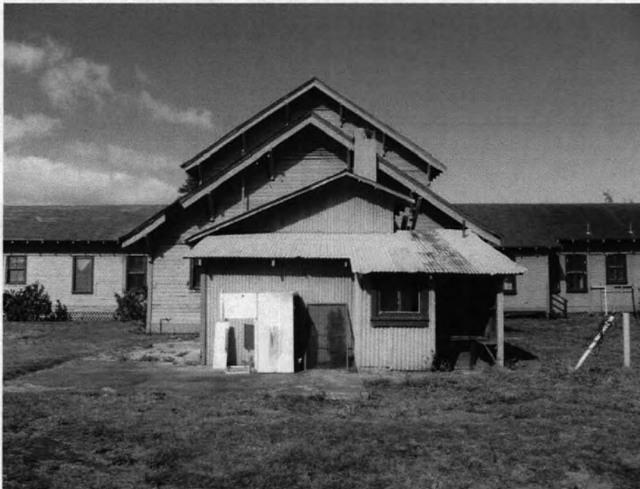
FBMH-005-003. Fred Baldwin Memorial Home, Building 005, Looking Northwest.
