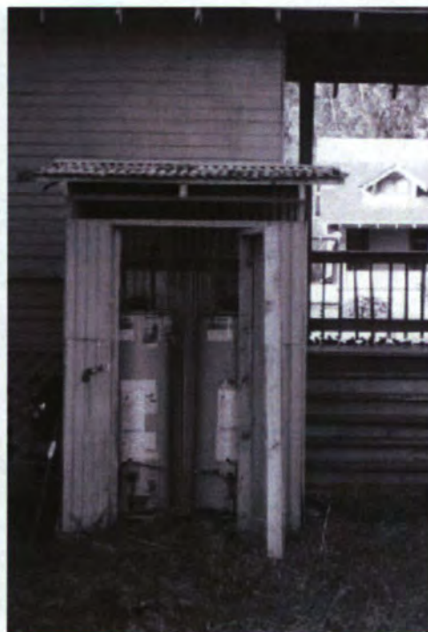
FBMH-008-002. Corrugated metal shed, Looking Northeast.
