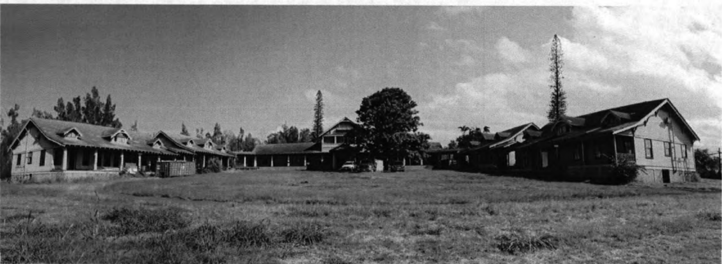
FBMH-S009. Fred Baldwin Memorial Home Site, (left-right) Buildings 001, 002, 003, 005, 006, 007, and 008, Looking Southeast.
