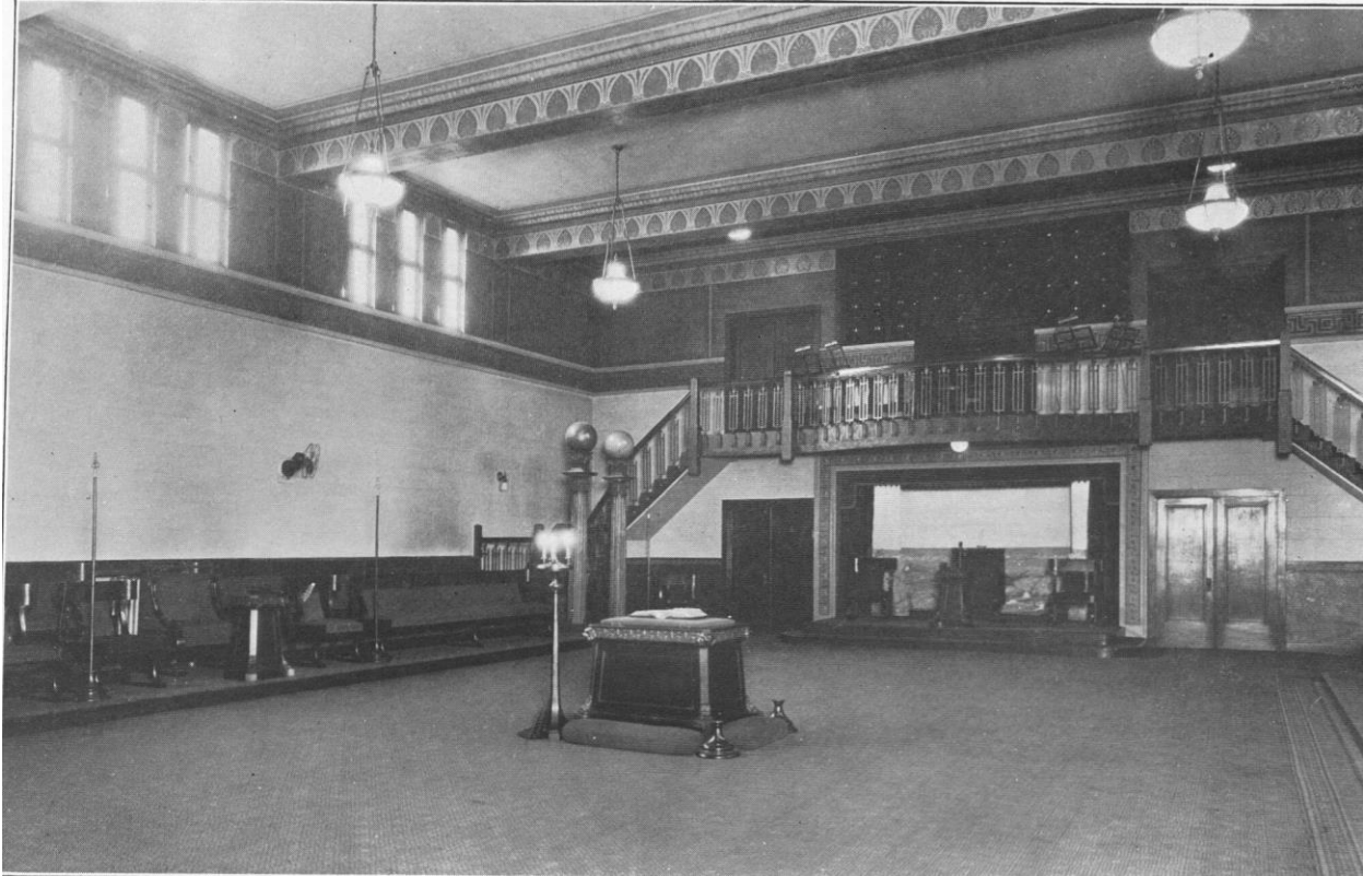
Historical Photograph 10--c. 1925 photograph of south and west walls of lodge room from northeast corner, from Historical Sketch of Oriental Lodge No. 500, F. & A. M., 1875-1925 , p. 60.
