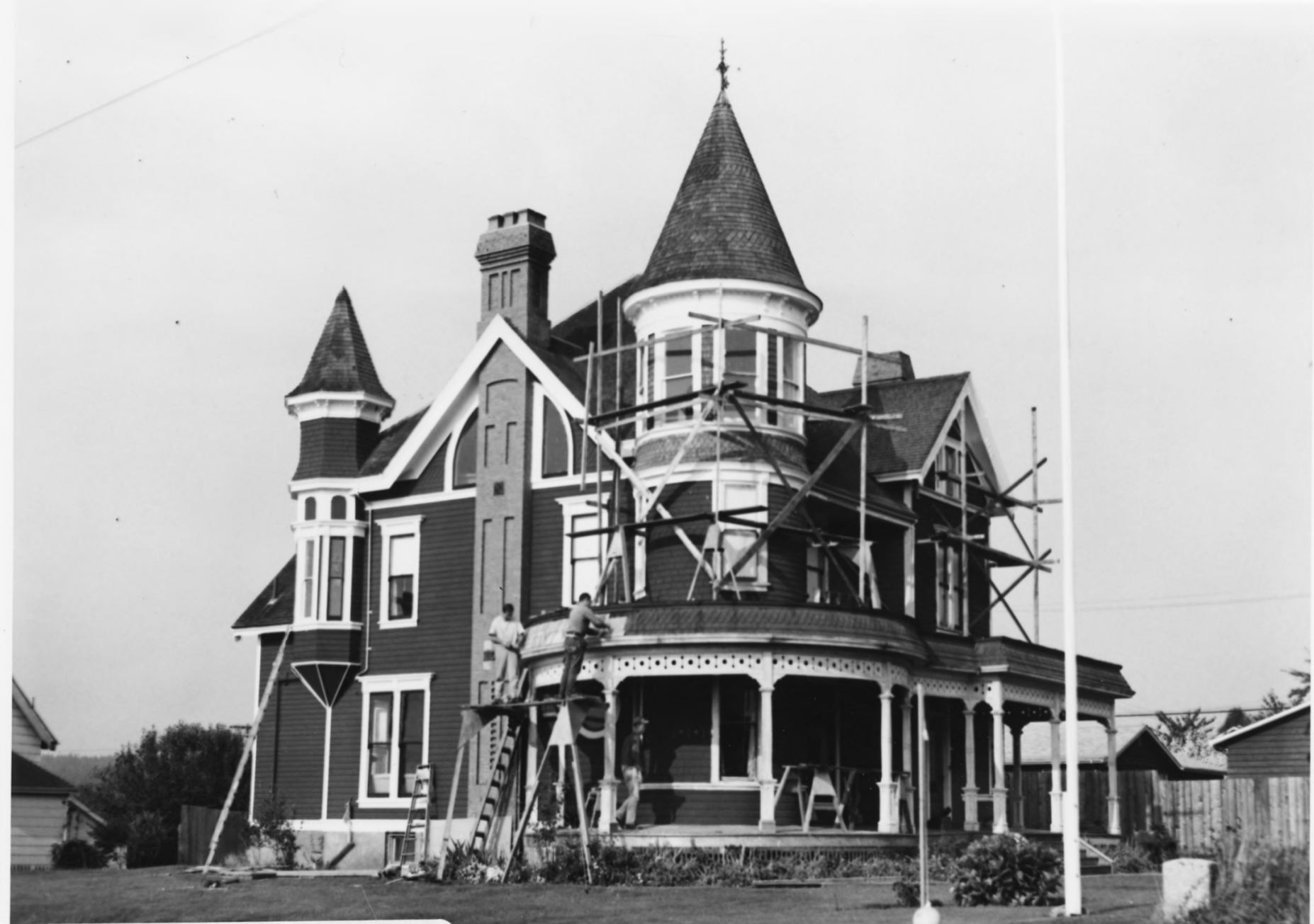
F. W. Hastings Residence, 1890
