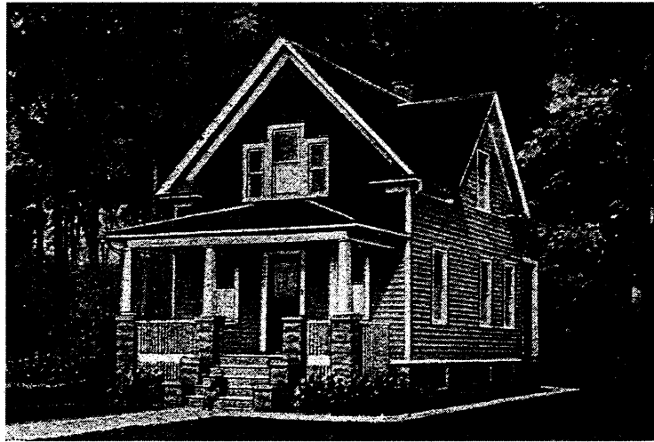
Figure 10: "The Yale," A kit home sold by the Aladdin Company in its 1917 Catalog.
