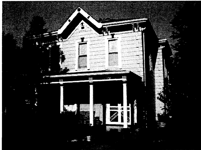
Figure 7 (below): The exterior material on the Congdon House, another Italianate home, is wood blocks.
