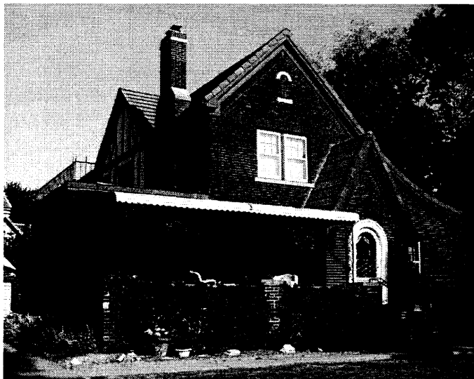
Figure 14: Property #99, a high-style example of Tudor Revival with asymmetrical design, arched openings, half-timbering, and a broken gable roof. Figure 15 (below right): Property #71, A Colonial Revival home with symmetrical design and side-gabled roof.
