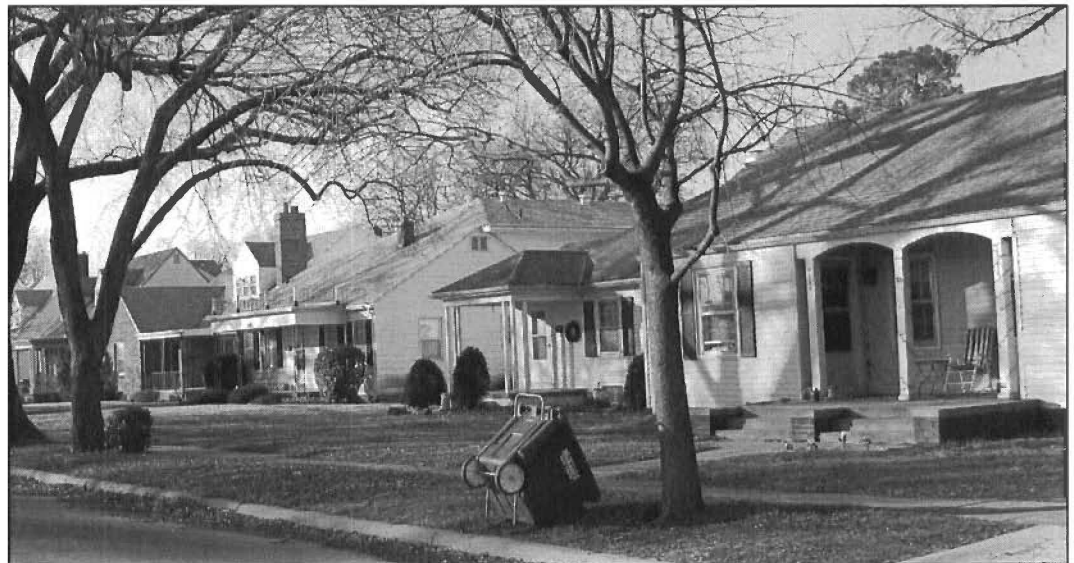
Examples of original wood porch posts built 1940s and replacement cast iron posts (no date). Left to right: 1437 (wood), 1441(iron), 1447 (iron), 1451-53 (wood), 1457-59 (wood) N Jeanette Avenue, Wichita. 85
