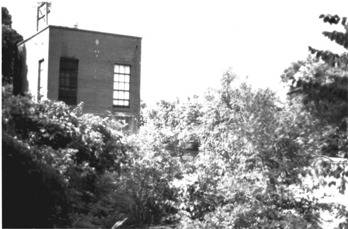
Walkermill Hydroelectric Station Sevierville vicinity, Sevier Co., TN
