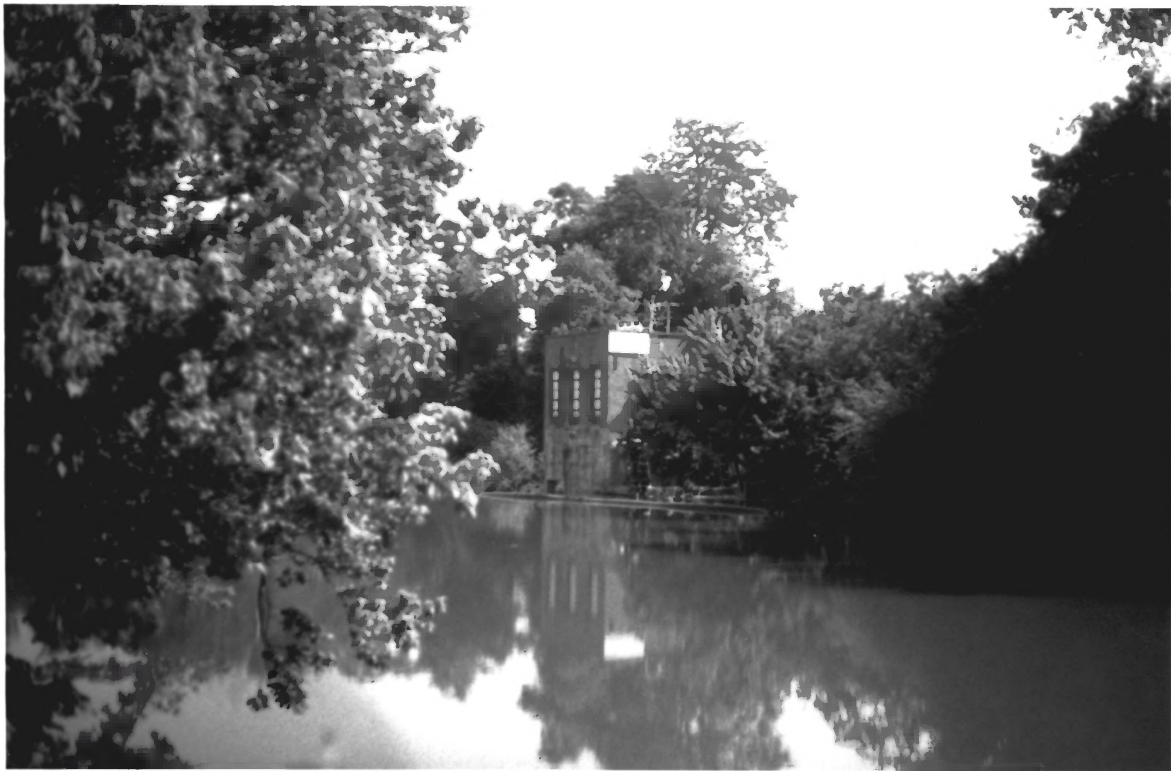
Walker Mill Hydroelectric Station Serierville vicinity, Sevier Co., TN
