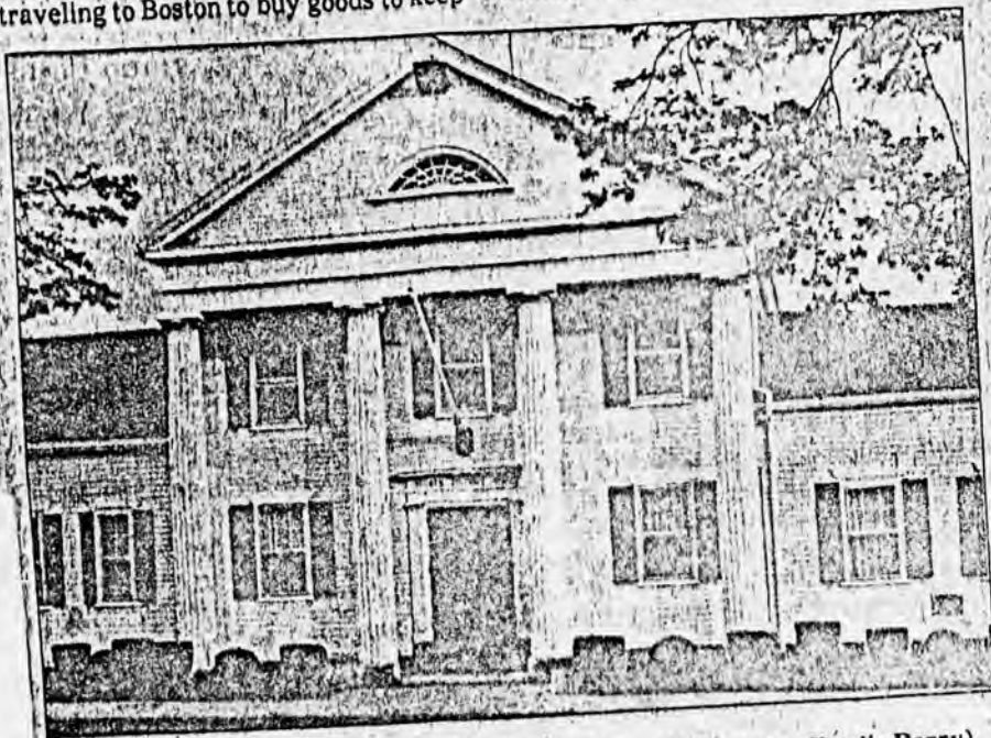
Middleboro Courthouse and Police Station. (Gazette Photo by Charlie Perry)
