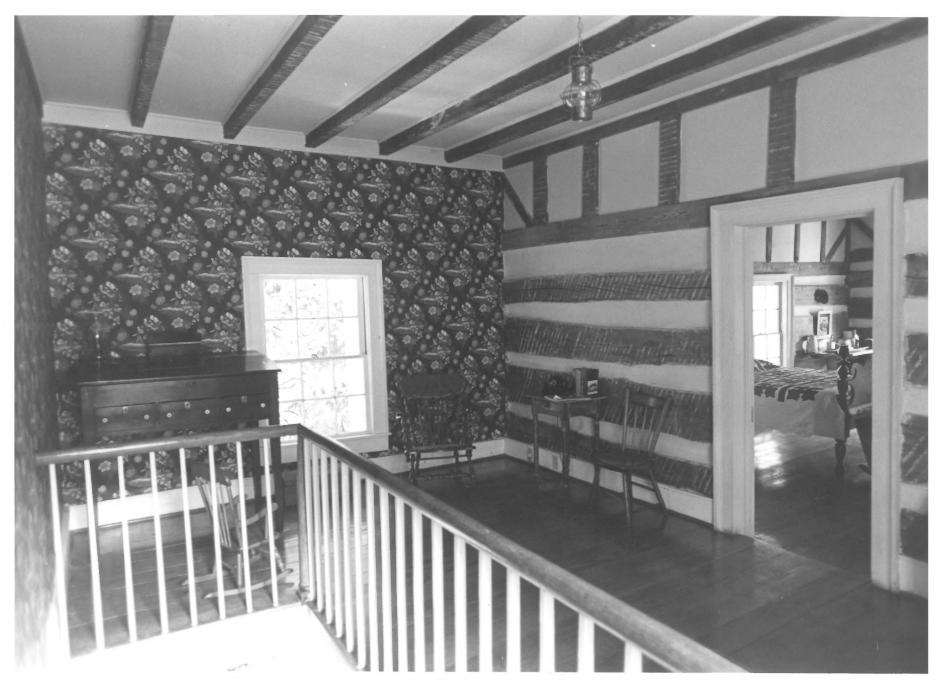
Photo No. 4 Hickory Sticks Columbus, Lowndes County, Mississippi Elizabeth P. Reynolds Mississippi Department of Archives and History Interior view: second floor hall with partial view of northwest chamber. showing log construction extended with timber framing; looking northwest
