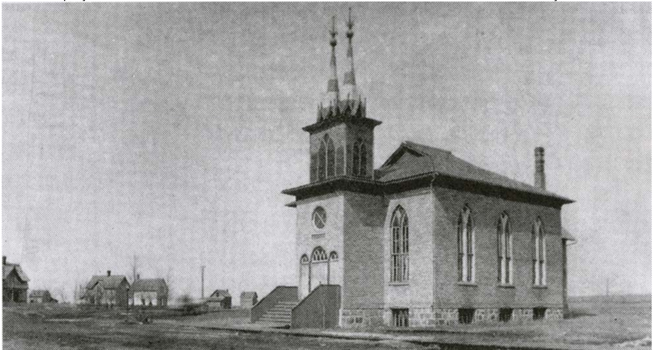
Figure 1. Trinity Lutheran Church, ca. 1901. Photo courtesy "Save the Trinity"
