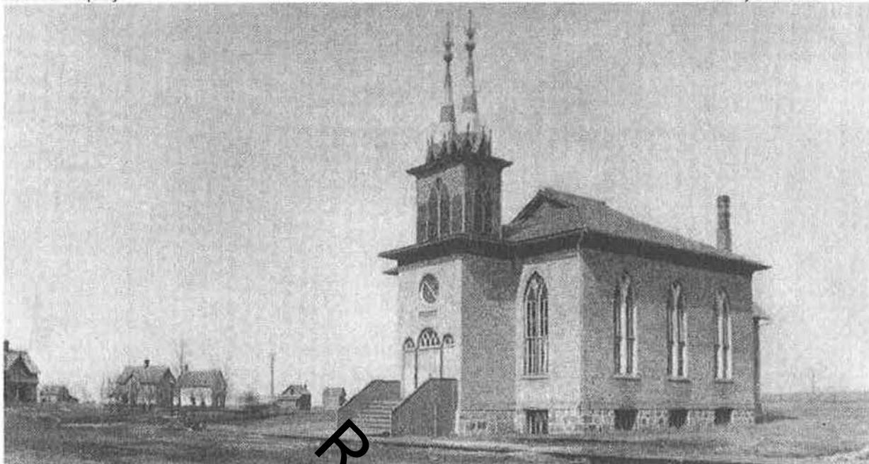
Figure 1. Trinity Lutheran Church, ca. 1901. Photo courtesy "Save the Trinity"
