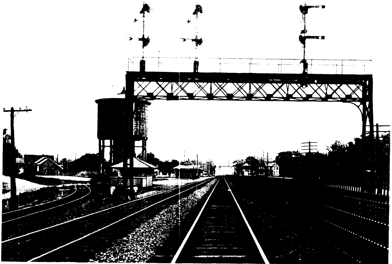
Lincoln Park looking west toward the station in 1925, the year the third and fourth tracks were added from Boonton.
