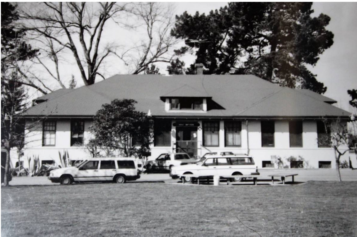
Figure 20: Men's Building, undated photo, early 1990s, on file at Napa County Building Department.
