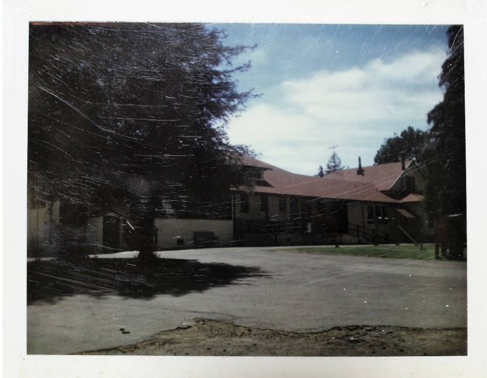
Figure 17: Main Building (rear elevation) and Hospital wing with Hospital wing right of frame, 1973, on file at Napa County Building Department.
