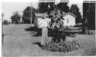
Circa 1935 Photograph of 67 East Allendale Road. Looking West. From SRHC files. Neg. file # 198351-18
