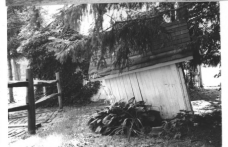
Necessary, accessory building #6. Neg. file # 190351-19
