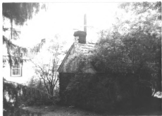
Smokehouse, Looking SE. Part of house in background. Neg. file # 3-11
