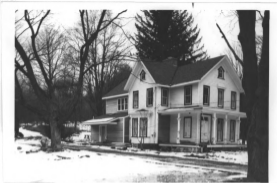
Photograph taken in 1984 showing recent alterations, especially those to the west wing. Neg. file # 19844-32.
