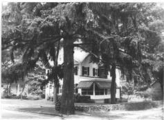
Looking NE showing front (west) and south sides Neg. file # 3-19
