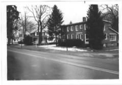
Photograph 13 View looking NE showing 148, 150, 152 and 154 W. Saddle River Road; D # 17, 19, 20, and 22. Neg. file # 19844-31.
