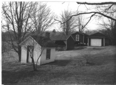
photograph of accessory buildings looking west, showing #2, 3, 4 and 5. Neg. file # 1-4 slide
