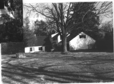
View looking SE showing sections B, A, C and the garage wing. Neg. file # 19852-3.
