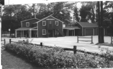
View looking east showing additions to building. Older section is the further away two-story block. Neg. file # 3-36.
