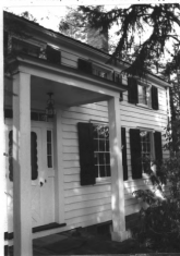
View looking NW showing section A. Neg. file # 19852-1.
