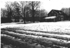
Photograph 3 The Ackerman-Pell Farm, 139 West Saddle River Road, D #13, looking SE, showing planting fields in the district. Neg. file # 19844-30.
