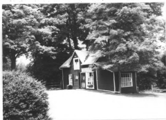
Carriage house of the Naugle-Crouter-Ackt House. Looking NE. Neg. file # 3-24,
