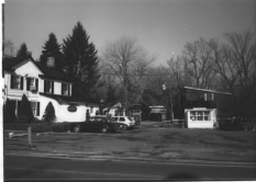
William Packer House and Accessory Buildings, 71 East Allendale Rd., Saddle River.
