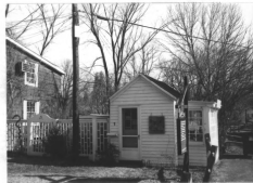
Looking east showing accessory building #1 and part of #2. Neg. file #1-16
