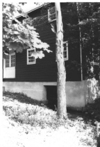
View looking NW showing rear (south) side of older part of building and part of raceway. Neg. file # 198351-23 slide
