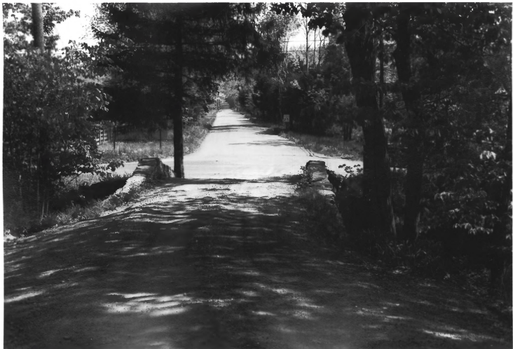
PALATINE ROAD BRIDGE, TEWKSBURY TWP., HUNTERDON CO.
