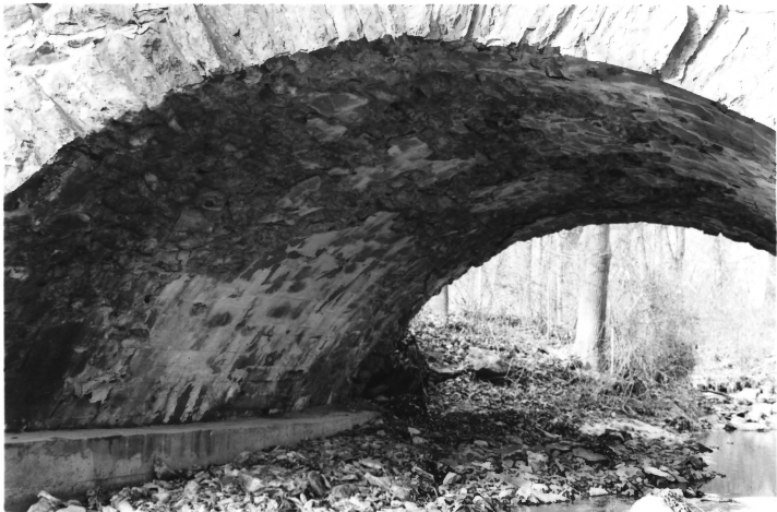
PALATINE ROAD BRIDGE, TEWKSBURY TOWNSHIP, HUNTERDON CO. PH 66
