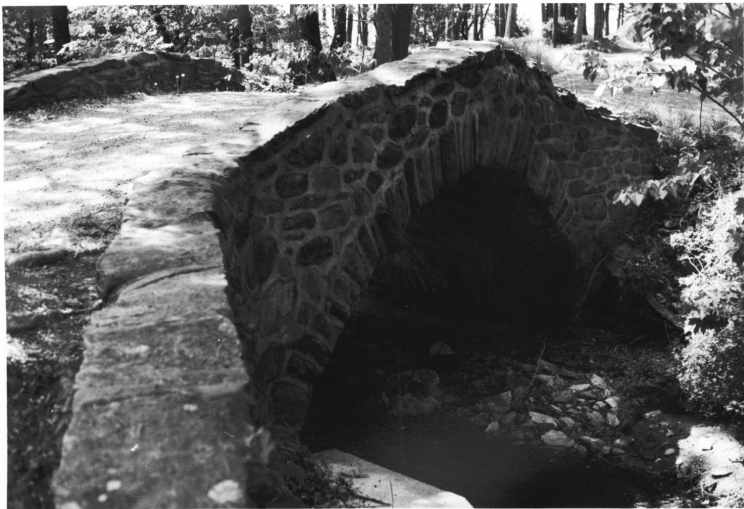
PALATINE ROAD BRIDGE, TEWKSBURY TWP., HUNTERDON CO.
