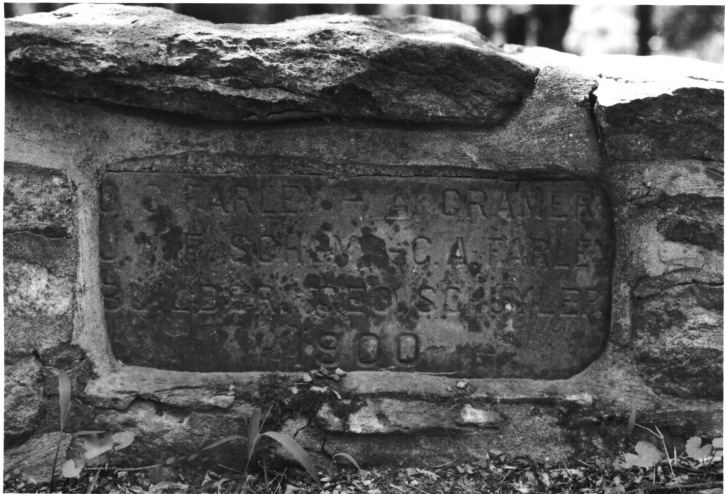
PALATINE ROAD BRIDGE, TEWKSBURY TWP., HUNTERDON CO. PHOTO 50P5
