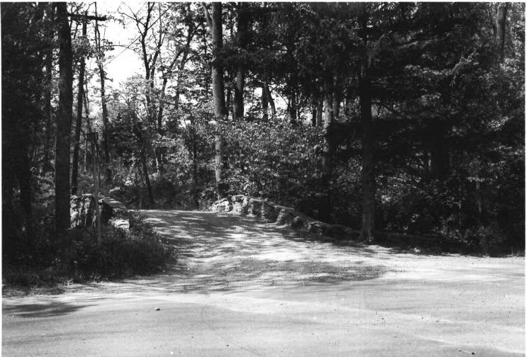
PALATINE ROAD BRIDGE, TEWKSBURY TWP., HUNTERDON CO. PHOTO 2075
