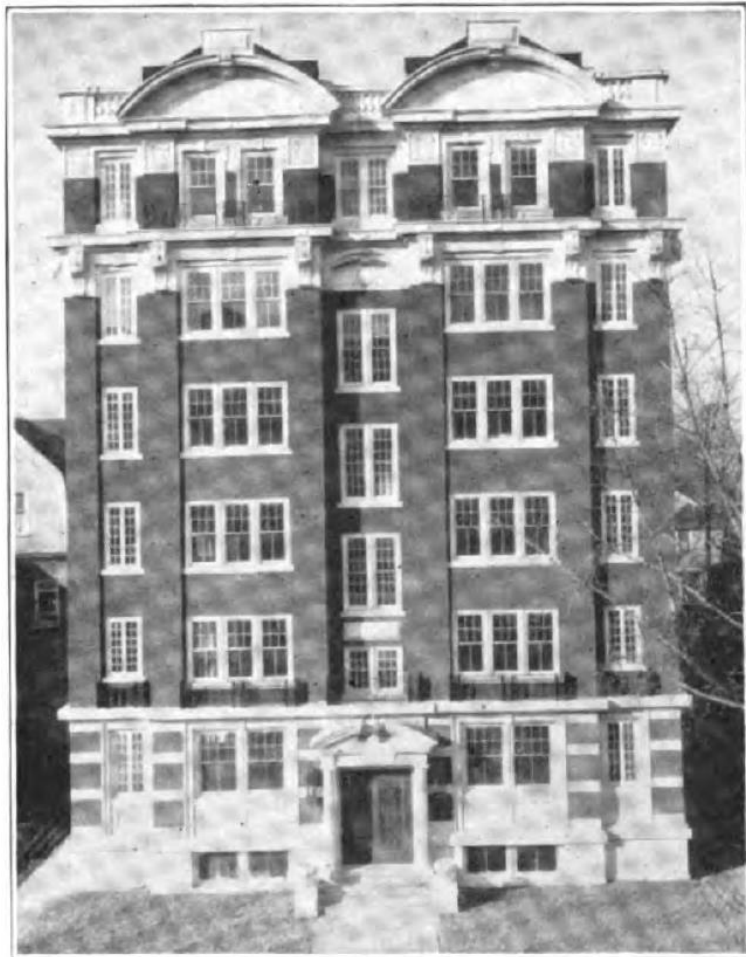
St. Rita Apartments, Detroit
