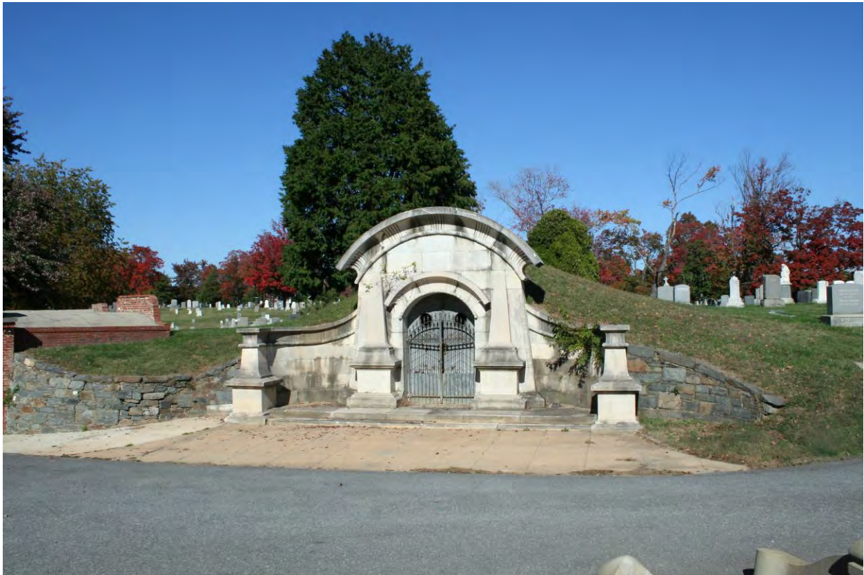
8 of 14. View looking northwest toward the entrance to the original mausoleum along Mulberry Avenue in Section G. Note papyrus entablature, obelisks, and pylon-like massing, evoking the Egyptian Revival style.
