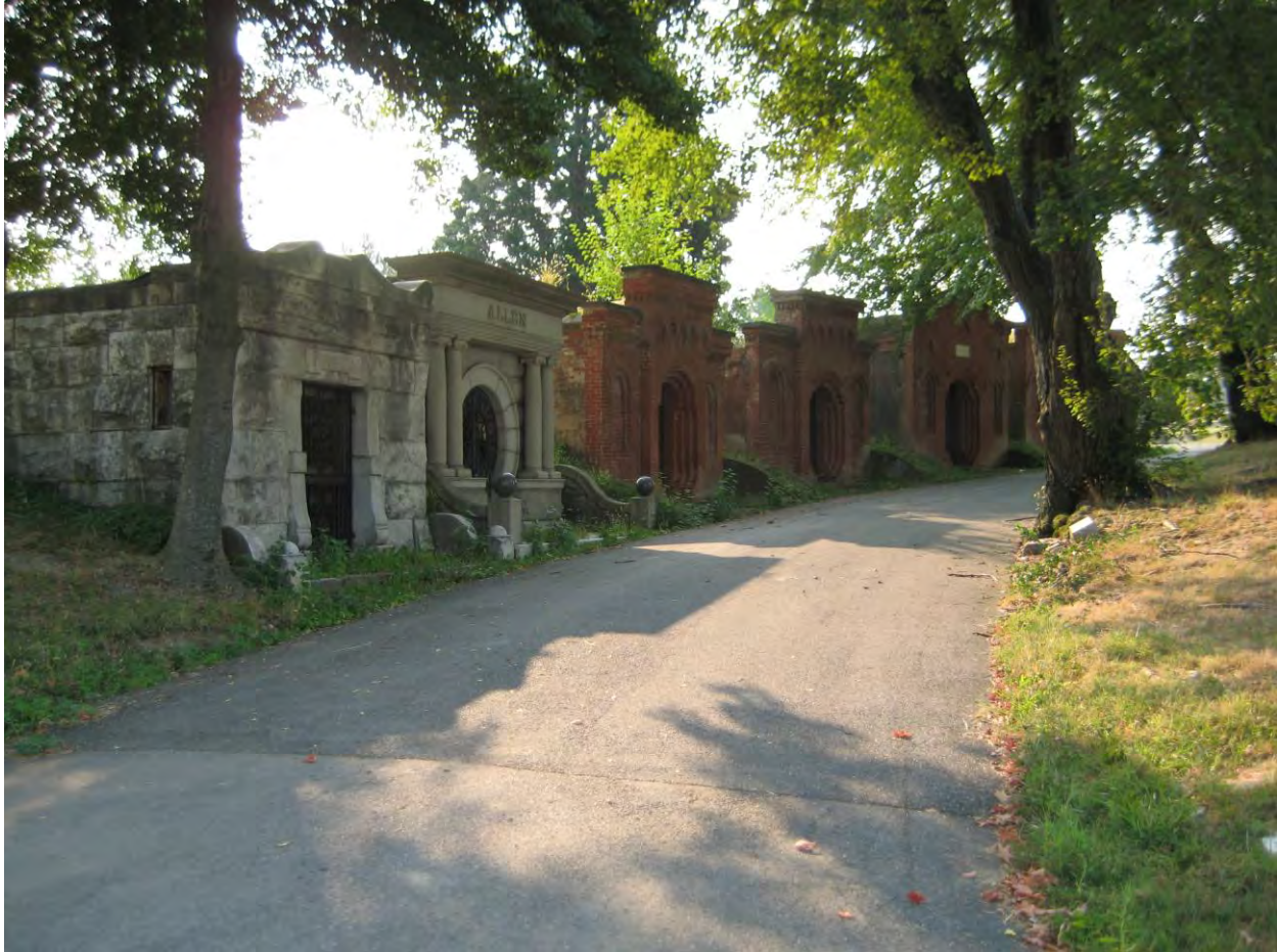
9 of 14. View looking southeast along Mulberry Avenue toward nineteenth- and early twentieth-century mausolea. Note the use of brick on nineteenth-century mausolea, compared to use of granite and limestone on early twentieth-century mausolea. In addition, note the horseshoe-arch entrance to the Allen mausoleum, second from left.
