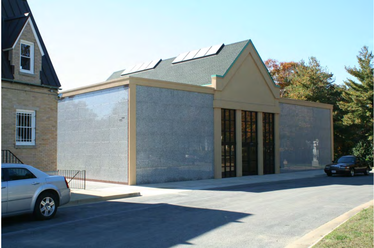
14 of 14. View looking southwest towards the north (primary) façade of the Mausoleum.
