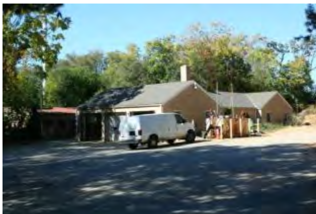
Photo 31: Maintenance Building and Shed
