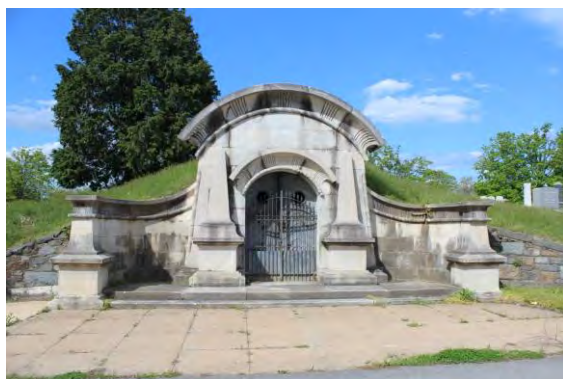
Photo 10: Public Mausoleum (Receiving Vault)
