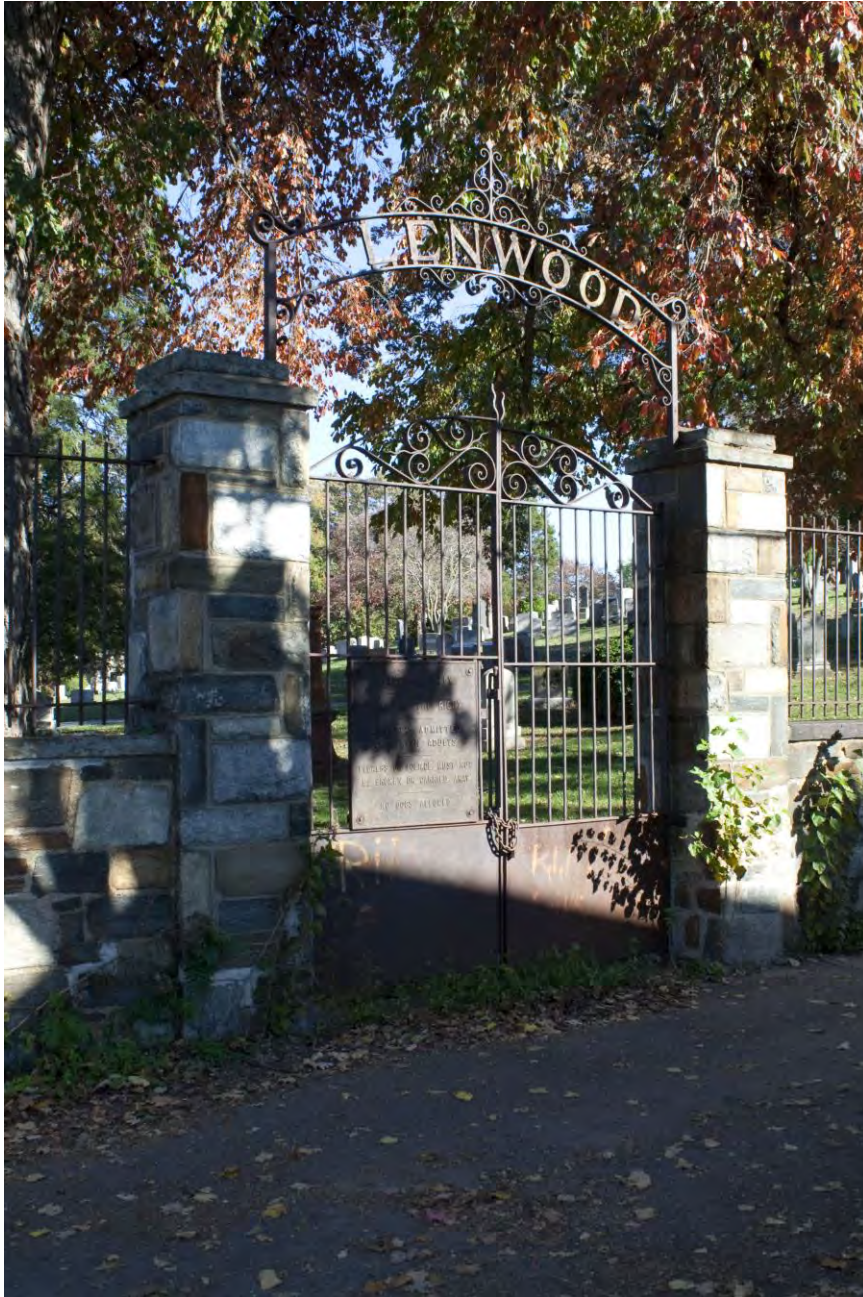
2 of 14. View looking southeast toward the pedestrian gate.
