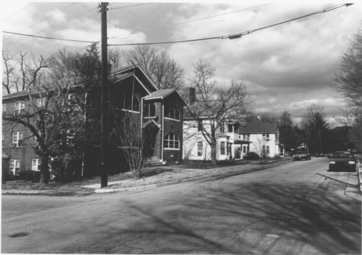
Indiana Avenue Historic District Maryville, Blount Co., TN Streetscape Stanley Ave. Photo # 306 2/2
