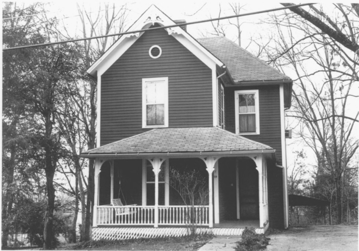
Indiana Avenue Historic District, Maryville, Blount Co., TN 119 Indiana Ave, Photo # 13 of 22
