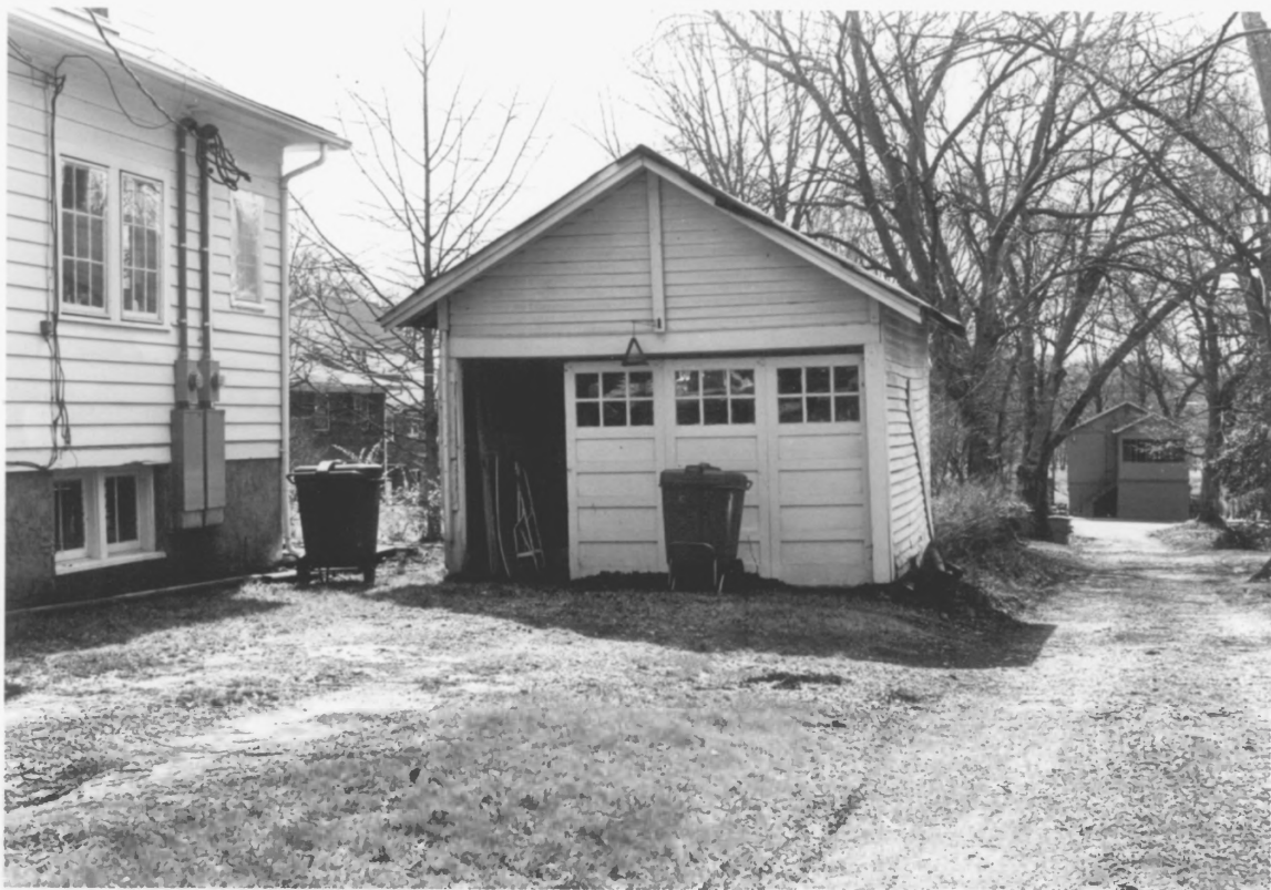
Indiana Avenue Historic District, Maryville, Blount Co., TN Garage at 319 Clark Street, Photo # 22 06 22
