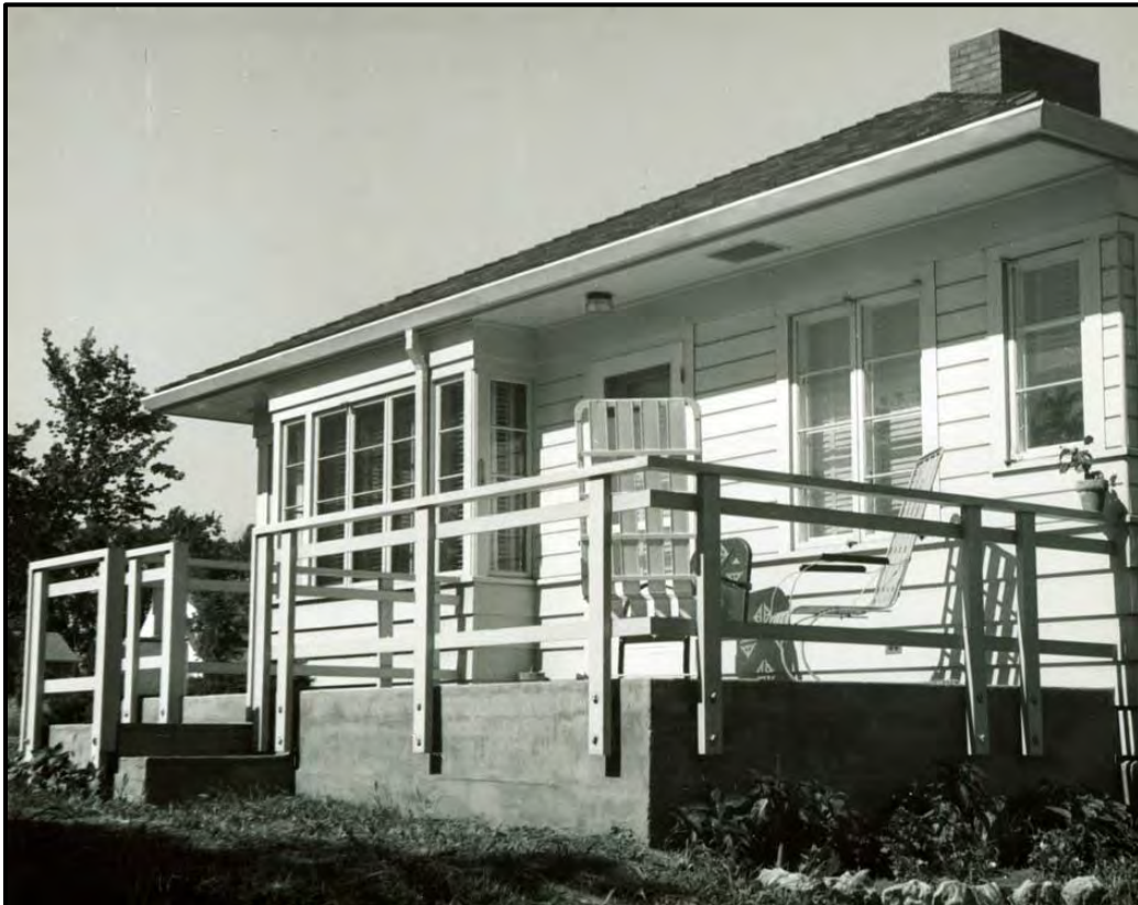
East Façade from Northeast
