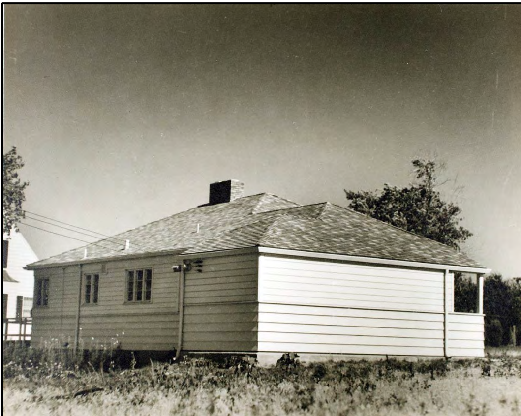
North & West Facades from Northwest
