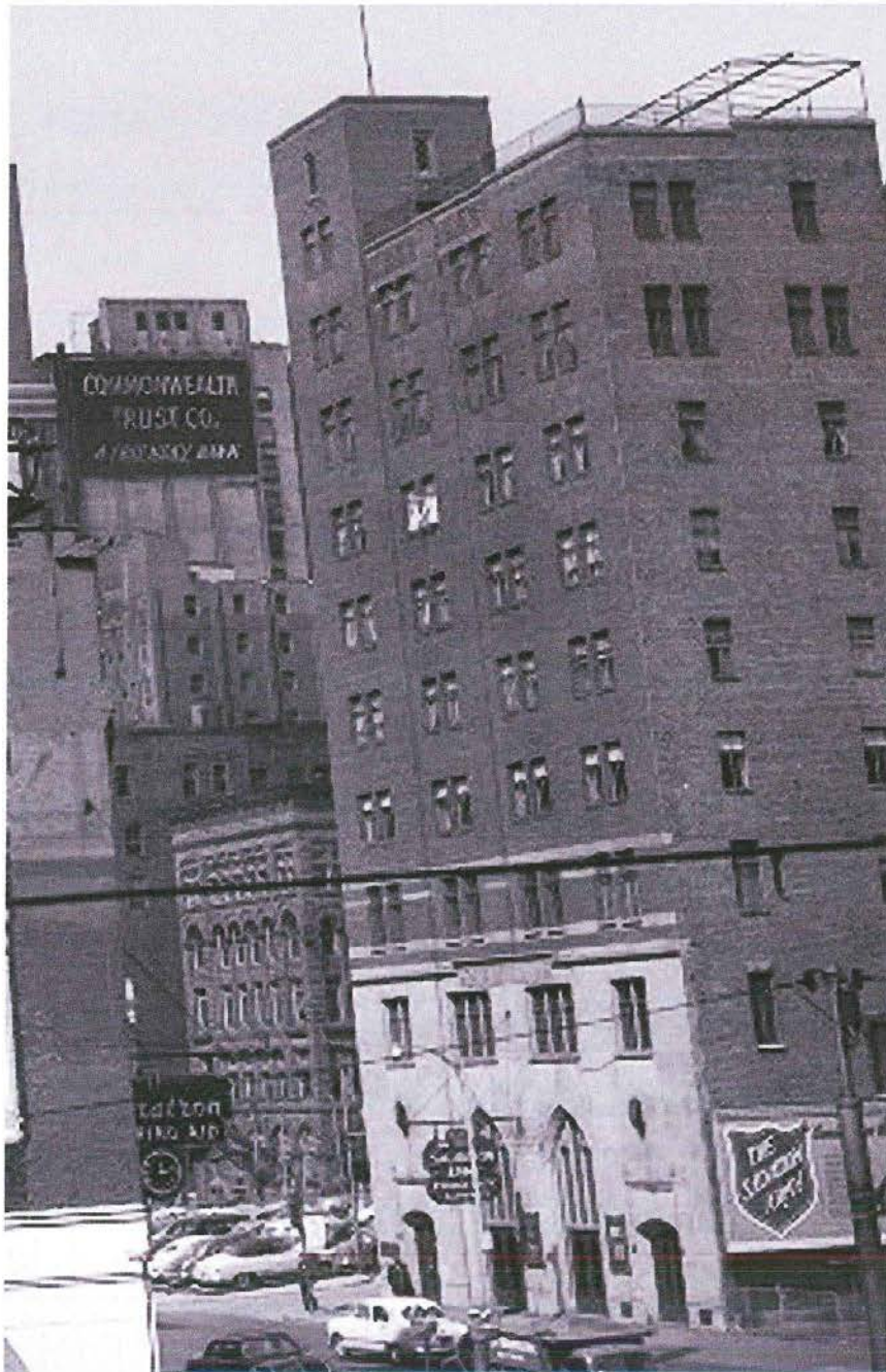
Figure 3 – The Salvation Army Building, c. 1950.
