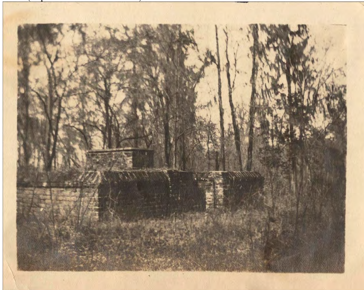
Figure 1: Smith vault and wall, St. James, Goose Creek, Cemetery, looking northwest, from William Henry Johnson Scrapbook, Volume 1, Image 342, Lowcountry Digital Library, original held at South Carolina Historical Society.
