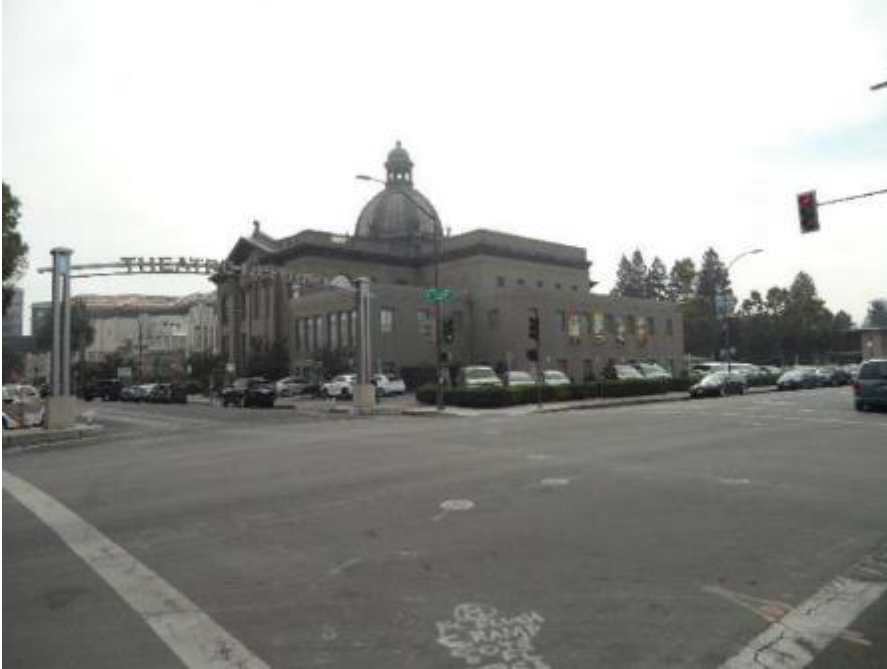
View from Marshall and Middlefield looking at rear.
