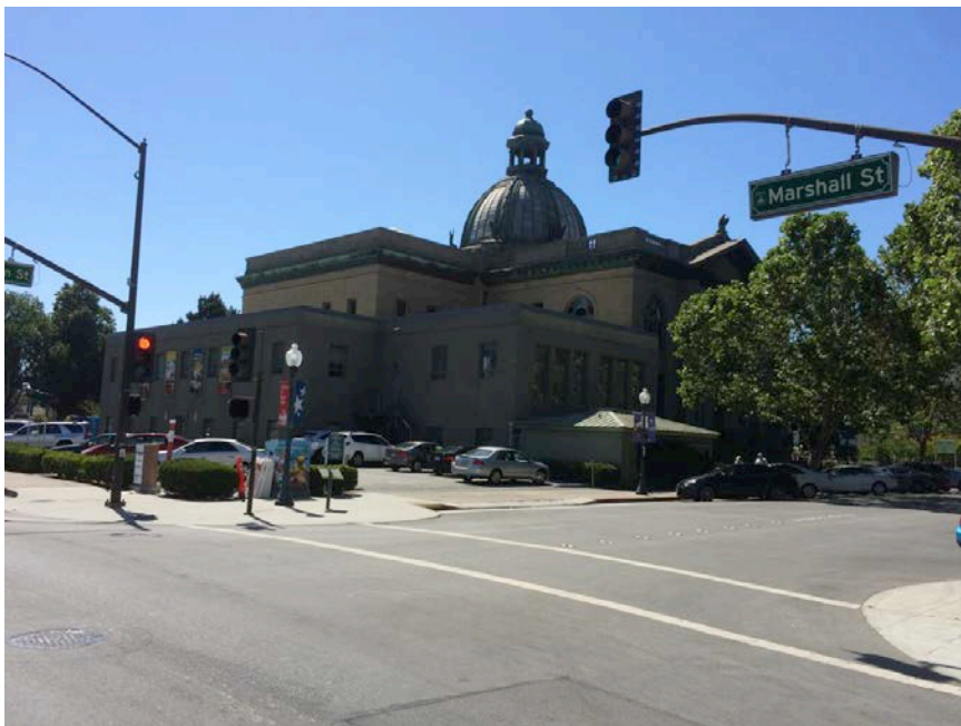
Figure 3. View of the receiver site from Marshall Street, looking southeast. (Garavaglia Architecture, Inc., 2017)
