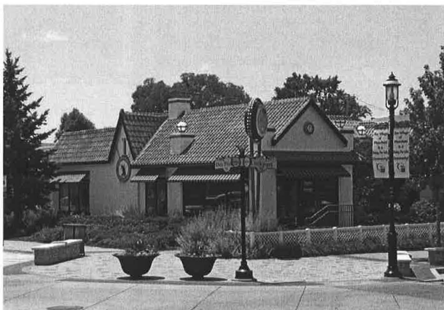
Figure 4 - View of 24103 Lockport Street showing the former Texaco Gas Station. This property is individually listed on the National Register. Source: Douglas Gilbert, AIA
