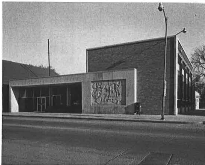
Figure 29 - Historic view of the 1960 addition to the original 1913 Plainfield National Bank Building at 24023 Lockport Street. It is an excellent example of the International Style and features a modernist stone mural by Phyllis Busse. Source: Plainfield Public Library
