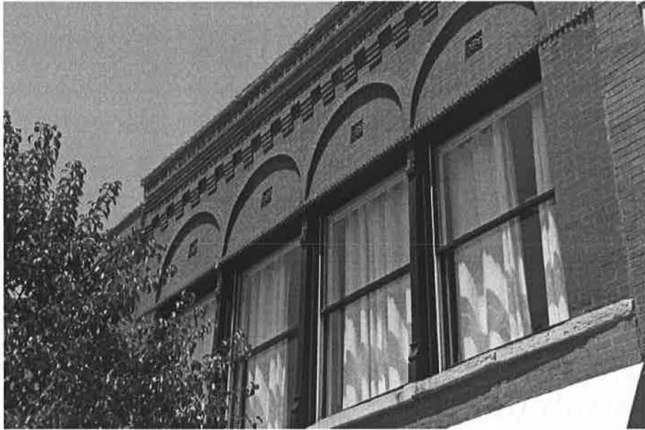
Figure 24 - View of the round arches and cornice of the Richardsonian Romanesque style building at 24038 Lockport Street. Source: Douglas Gilbert, AIA
