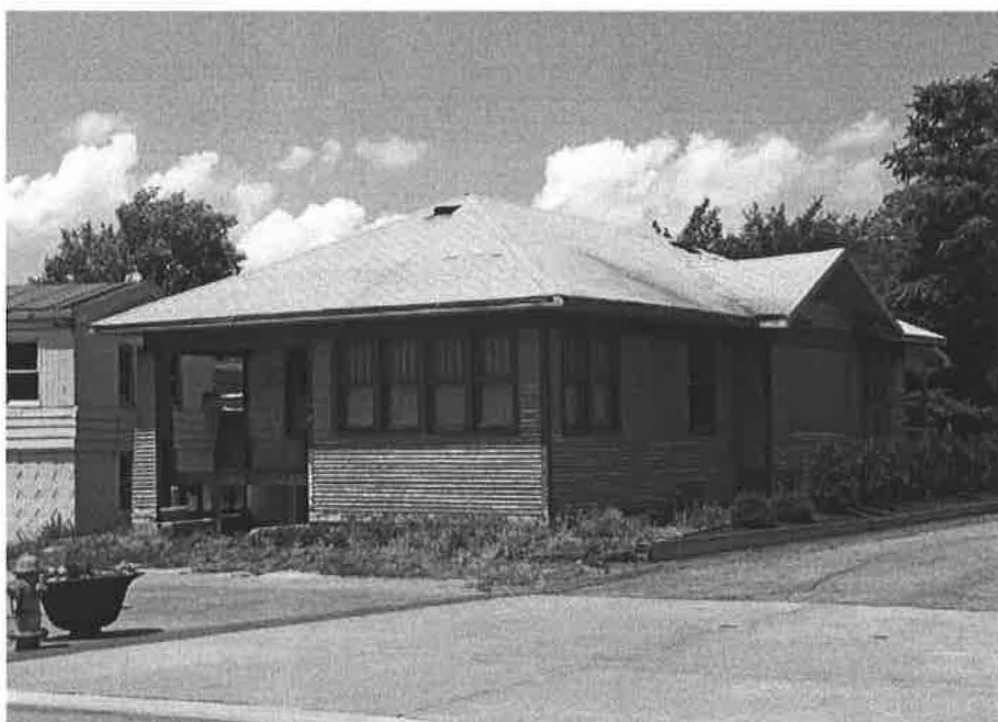
Figure 27 - View of a classic bungalow house at 24210 Lockport Street. Source: Douglas Gilbert, AIA
