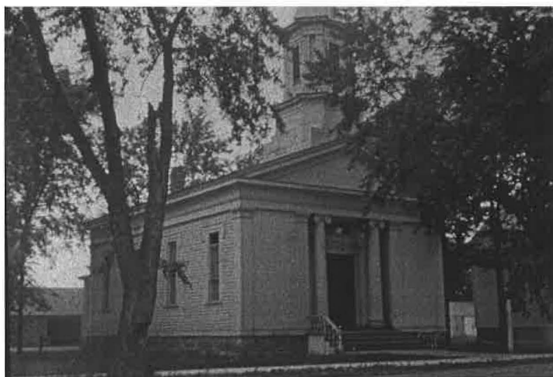
Figure 21 - Historic view of the Congregational Church at 24022 Lockport Street, prior to the west addition. Source: Plainfield Public Library
