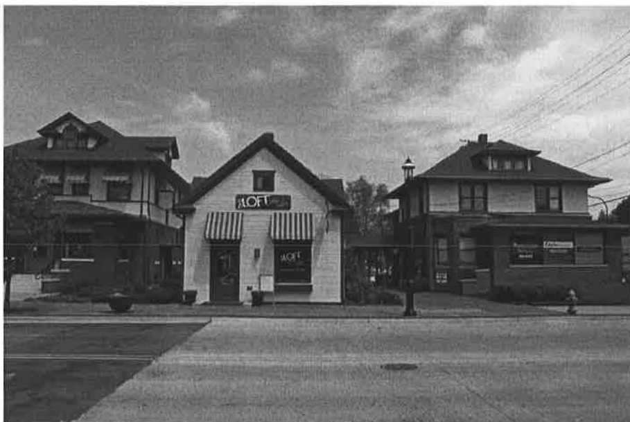
Figure 26 - View of two foursquare type homes at the east end of Lockport Street. The right building is 24004 Lockport and designed with strong Prairie Style influences. The left building is 24012 and was built as the St. Mary Immaculate Parsonage with some Prairie Style and Colonial Revival Style influences. Source: Douglas Gilbert, AIA
