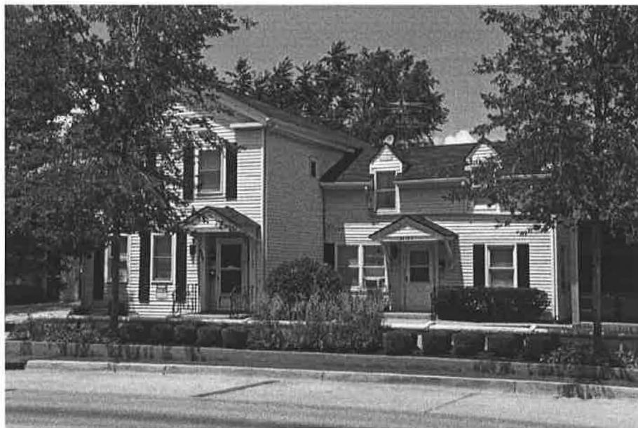
Figure 23 - View of the Ira Vanolinda House, built in 1851 by John Root Kent. It is a good example of a Greek Revival style upright and wing type house. Source: Douglas Gilbert, AIA
