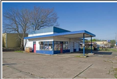
201 W. Main Street (C), with warehouse (NC) 1948, Modern
