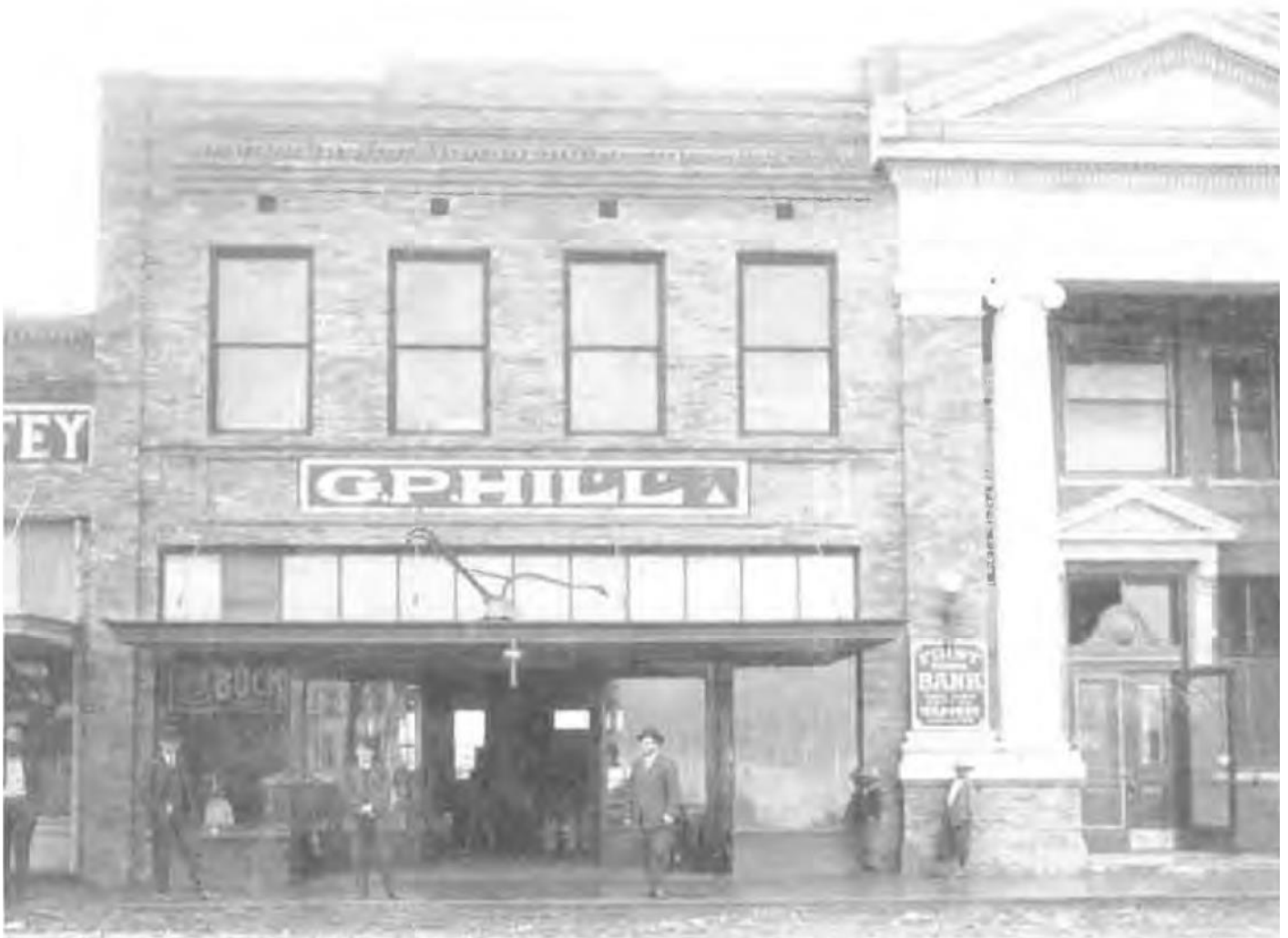
Figure 15: 1914 photo of present-day Chophouse on Bankhead (left) and Franklin County Library (right) prior to façade changes. Photo published in A Walk Through Mt. Vernon .
