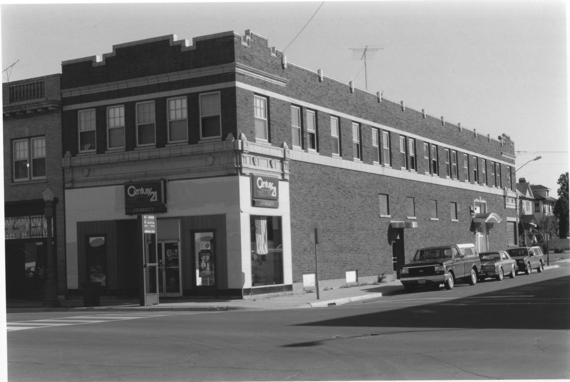
202 EAST HOWARD STREET, HIBBING HARDWARE COMPANY EAST HOWARD STREET COMMERCIAL HISTORIC DISTRICT HIBBING, ST. LOUIS COUNTY, MINNESOTA # 011021-2
