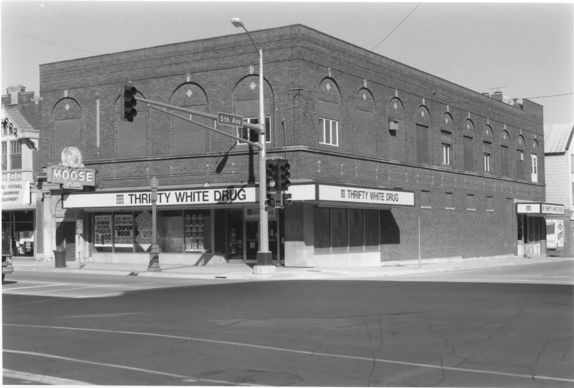
421 EAST HOWARD STREET, KELLY FURNITURE COMPANY EAST HOWARD STREET COMMERCIAL HISTORIC DISTRICT HIBBING, ST. LOUIS COUNTY, MINNESOTA #011019-13A/14
