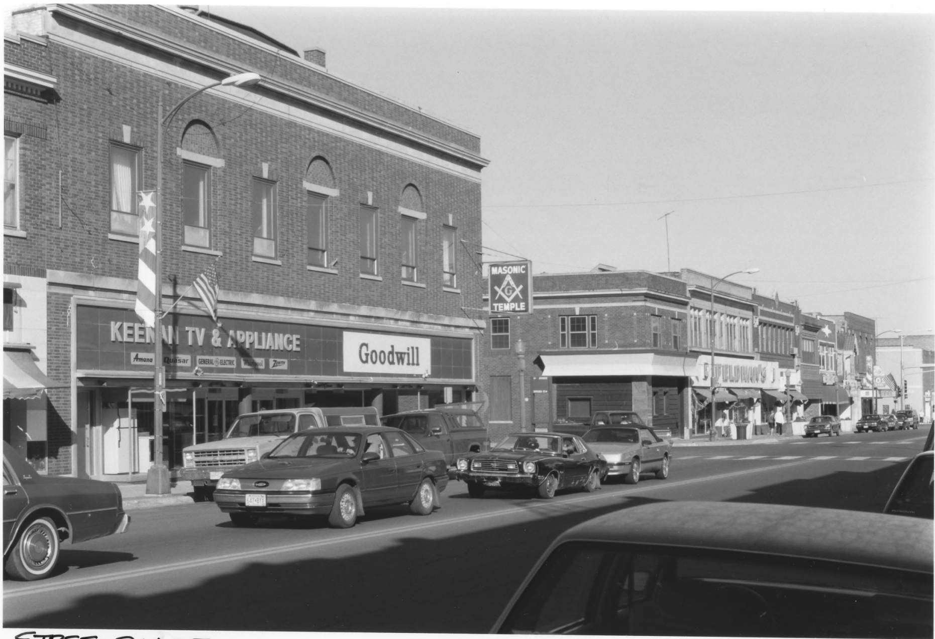
STREETSCAPE EAST HOWARD STREET COMMERCIAL HISTORIC DISTRICT HIBBING, ST. LOUIS COUNTY, MINNESOTA #011021-18
