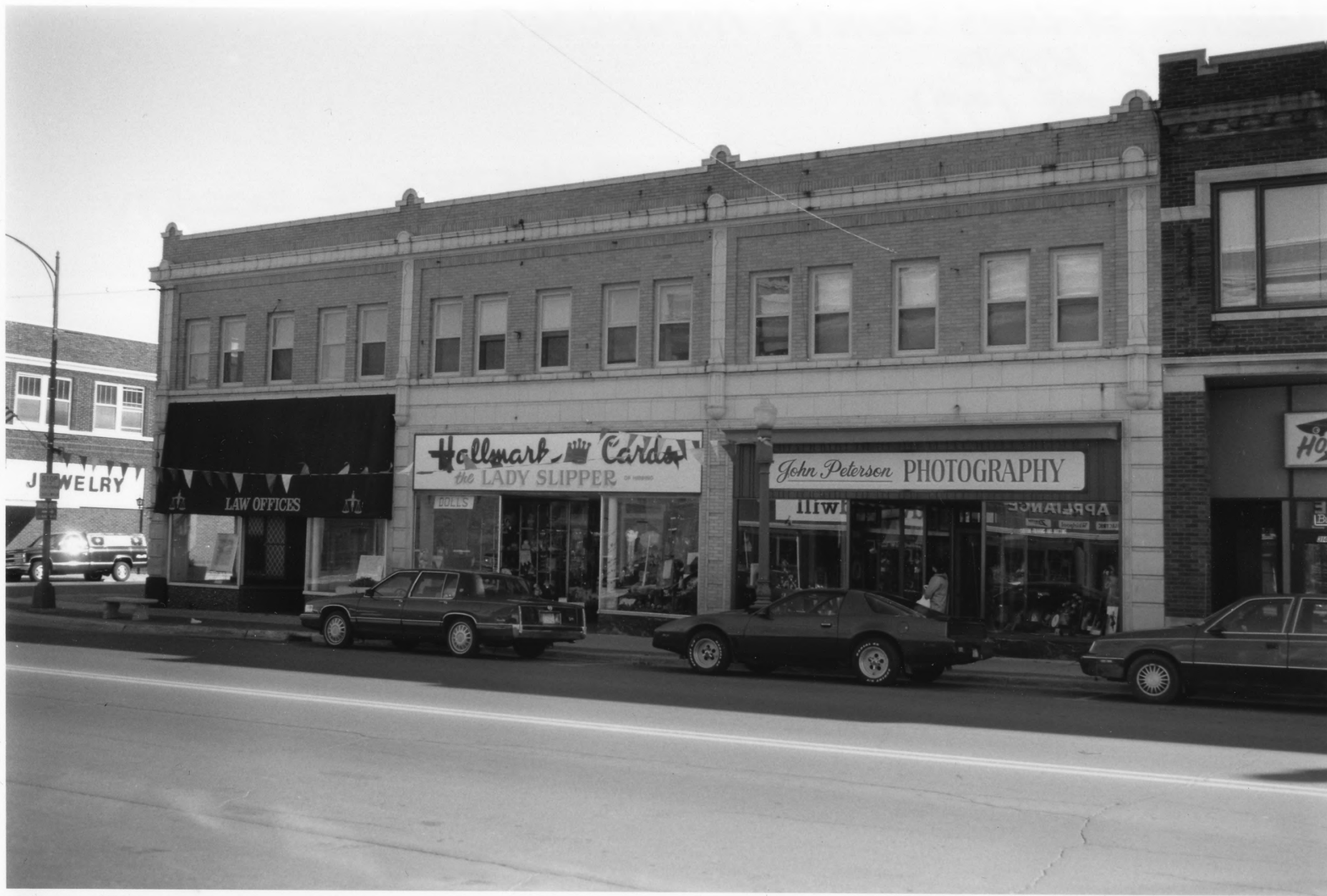
EAST HOWARD STREET COMMERCIAL HISTORIC DISTRICT - 316-320, HIBBING, ST. LOUIS COUNTY, MINNESOTA #011020-18 THOUIN-COONS BUILDING AND ANNEX
