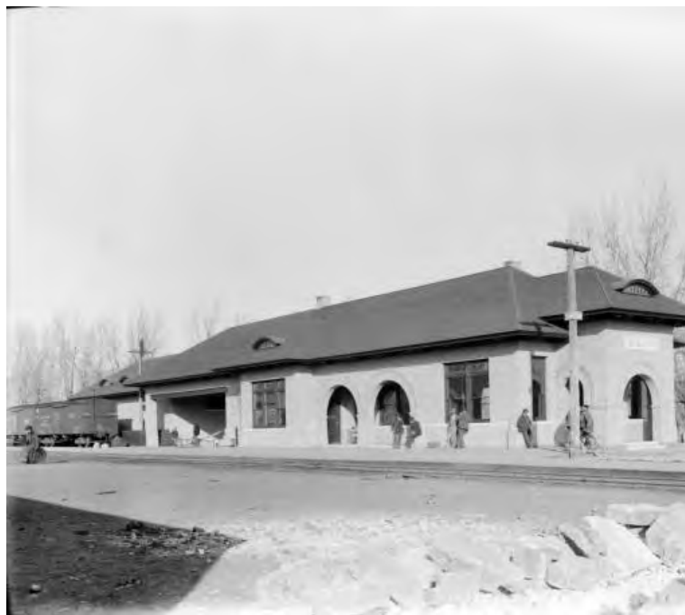
Figure 2: Colorado and Southern Railway Depot, 409-427 N. Railroad Ave. View to NE, ca. 1905. Courtesy Loveland Public Library, Loveland, Colorado.
