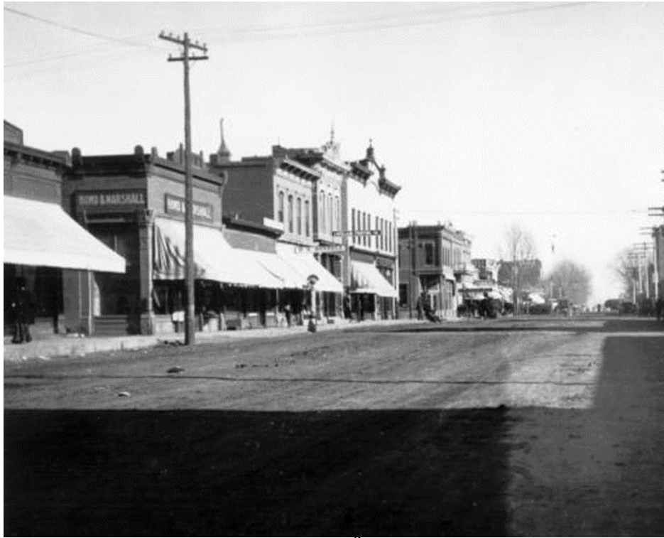
Figure 3: 100 block of E. 4 th St., view to NE, 1905. Courtesy Loveland Public Library, Loveland, Colorado.
