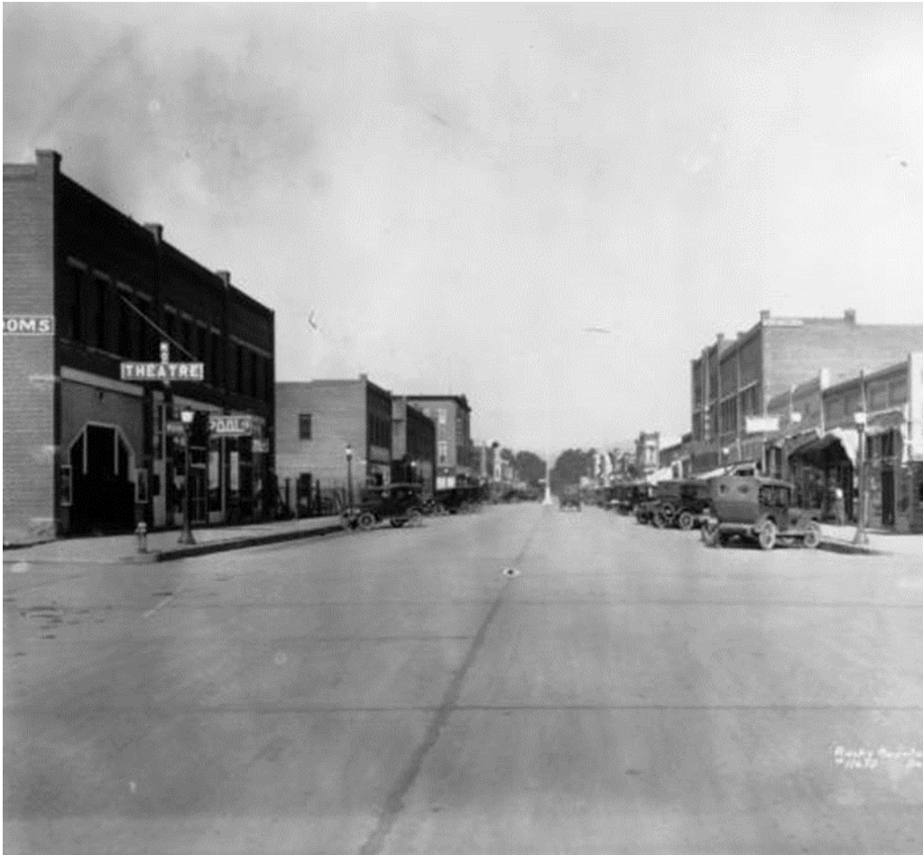
Figure 6: 300 block of E. 4 th St., view to West, 1919. Courtesy Loveland Public Library, Loveland, Colorado.
