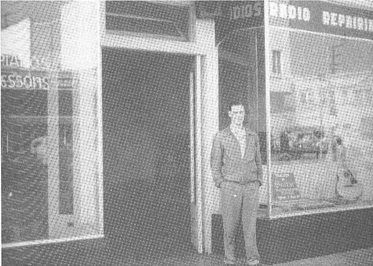
Figure 1: Front (east elevation) of building, circa 1948, Dale Hyatt pictured
