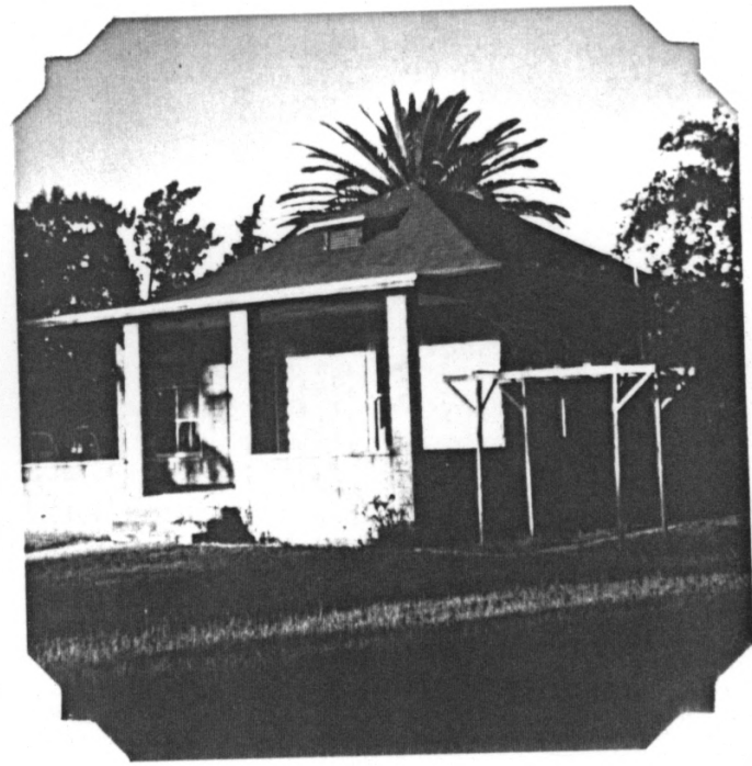
Looking Northeast, towards front of house
