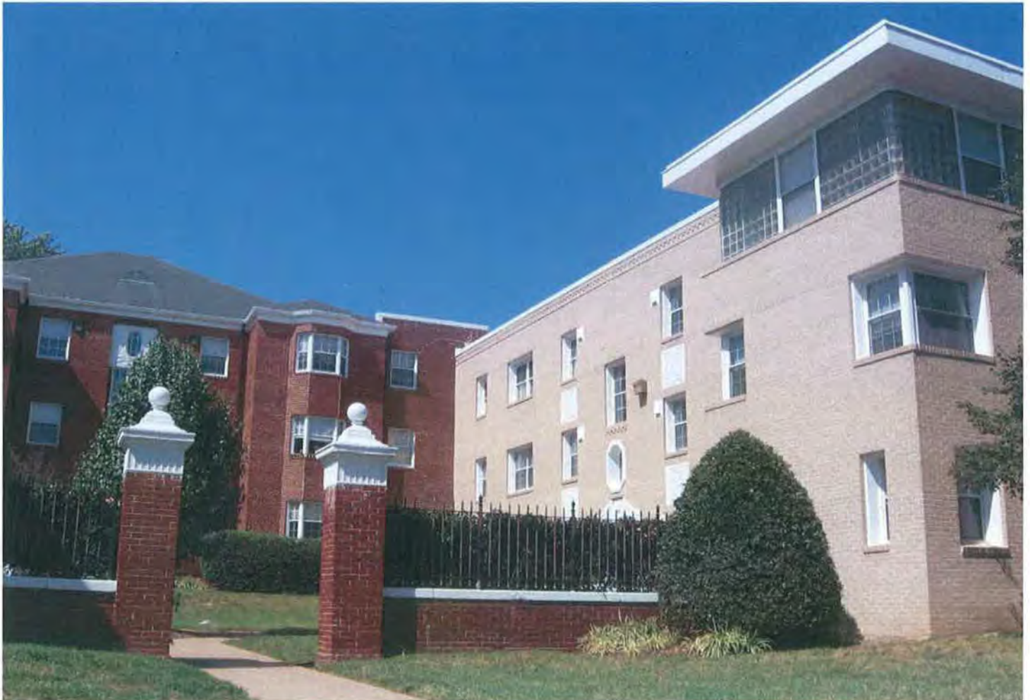
22 of 22, Buildings within the Lee Gardens South Apartments Complex (now Sheffield Court), Arlington, VA ( https://farm7.staticflickr.com )
