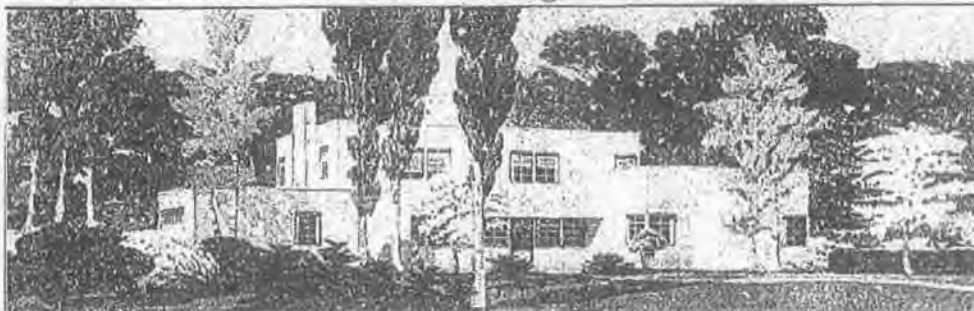
The first pre-fabricated 'motohome' to be built in the Washington area is under construction on Brookside drive, in Kenwood, Chevy Chase, Md., for Lee D. Butler, prominent Washington automobile distributor. The house is built of prefabricated steel into which are set floor-roof panels of compressed asbestos and cement, said to be indestructible. The house contains 12 rooms, 3 baths and a 2-car garage. A 'moto-unit,' a mechanism no larger than a pantry, operates the air-conditioning, heating and hot water units. The above sketch is an artist's conception of what Mr. Butler's new home will look like when completed.
