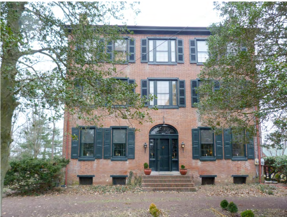
NJ_BURLINGTON_RIDGWAY, HOUSE, WILLIAM_0011 View facing north showing the south elevation.
