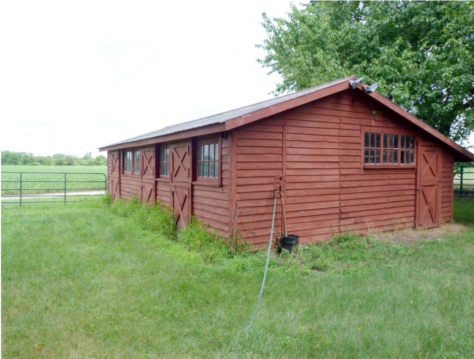
NJ_BURLINGTON_RIDGWAY, HOUSE, WILLIAM_0054
