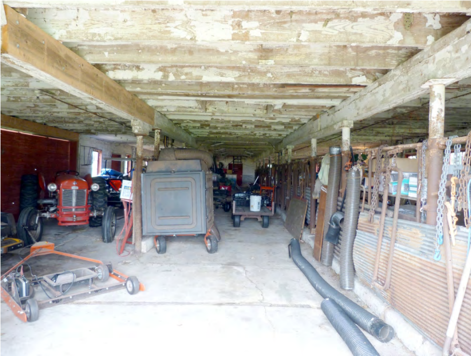
NJ_BURLINGTON_RIDGWAY, HOUSE, WILLIAM_0050 View facing north in the middle of the first floor of the barn.
