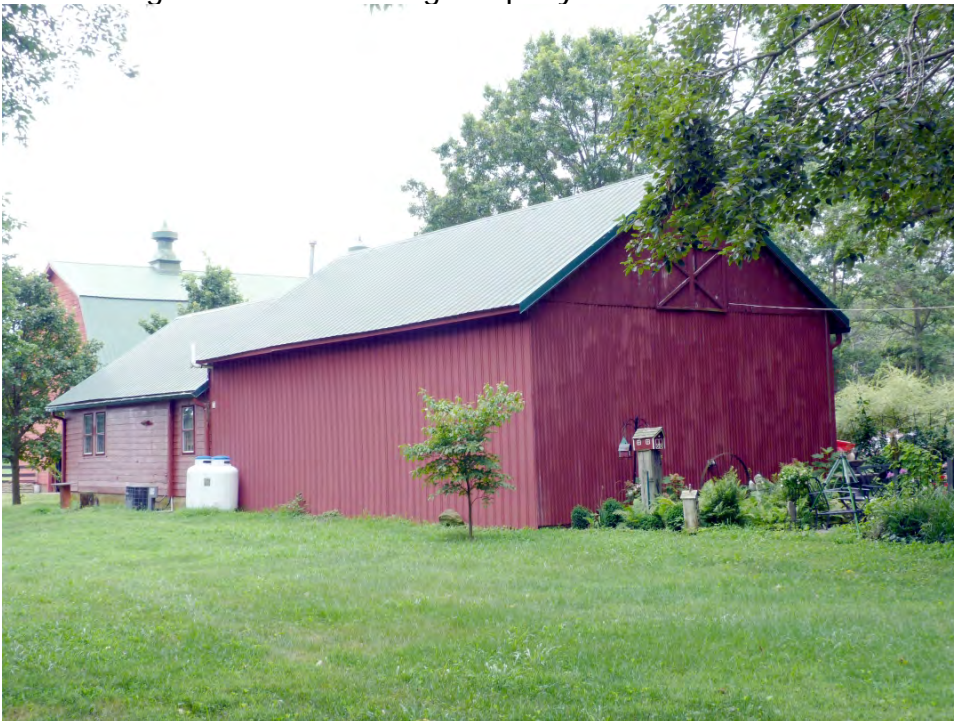
NJ_BURLINGTON_RIDGWAY, HOUSE, WILLIAM_0057 View facing SE showing the north and west elevations of the corn crib/schoolhouse.
