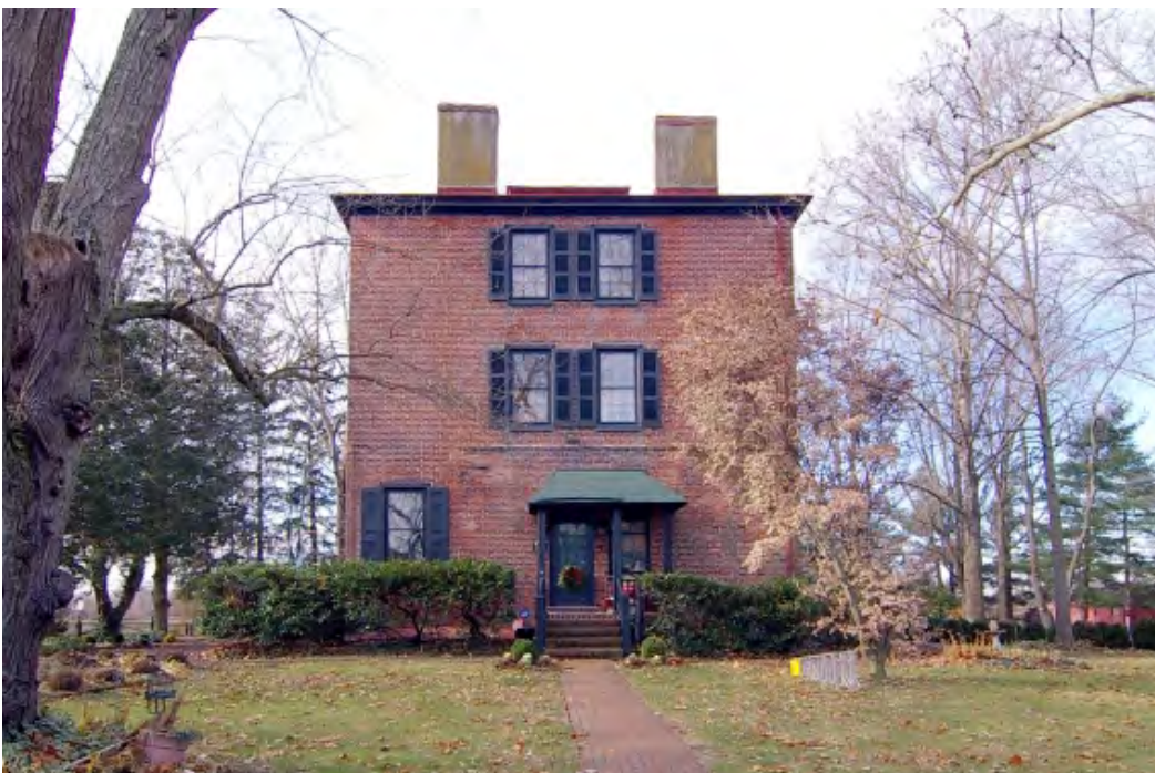
NJ_BURLINGTON_RIDGWAY, HOUSE, WILLIAM_0017 View facing west showing the east elevation and surrounding landscaping.
