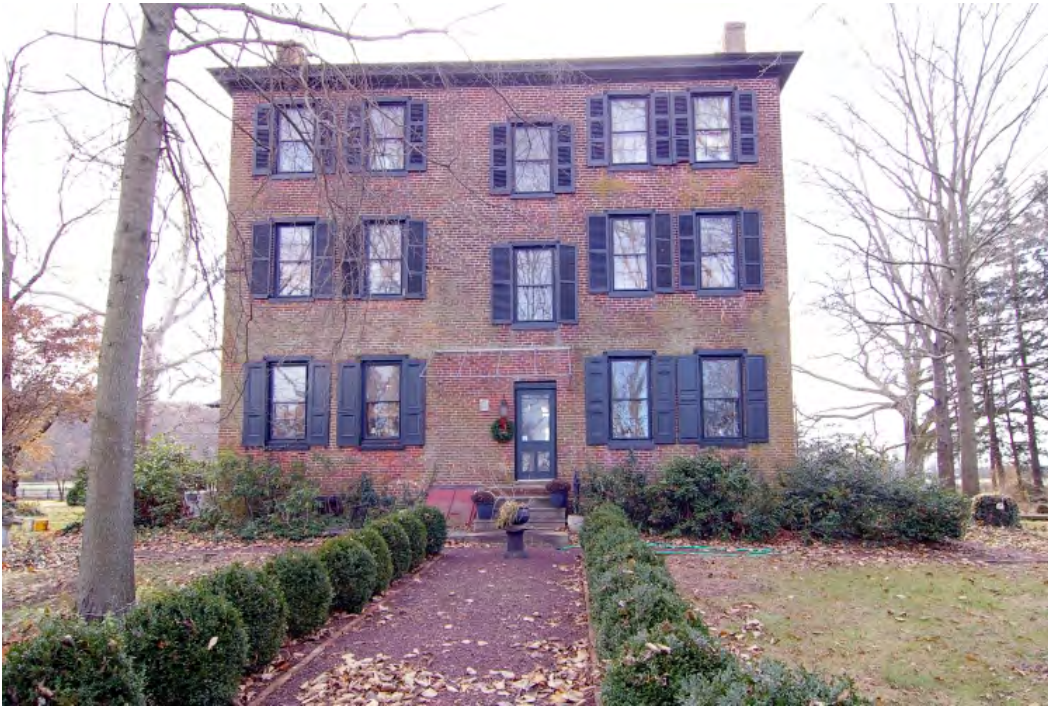
NJ_BURLINGTON_RIDGWAY, HOUSE, WILLIAM_0016 View facing south showing the north elevation.
