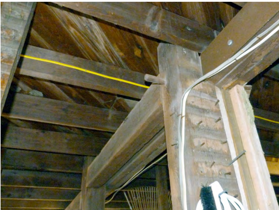
NJ_BURLINGTON_RIDGWAY, HOUSE, WILLIAM_0059 Detail facing northwest showing framing inside the corn crib.
