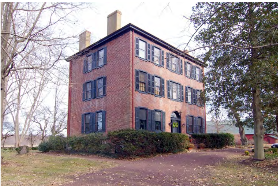
NJ_BURLINGTON_RIDGWAY, HOUSE, WILLIAM_0015 View facing northeast showing the west and south elevations with the paired interior end chimneys.
