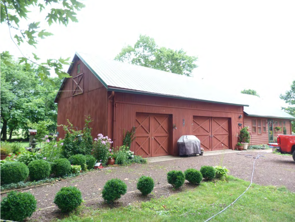
NJ_BURLINGTON_RIDGWAY, HOUSE, WILLIAM_0008
