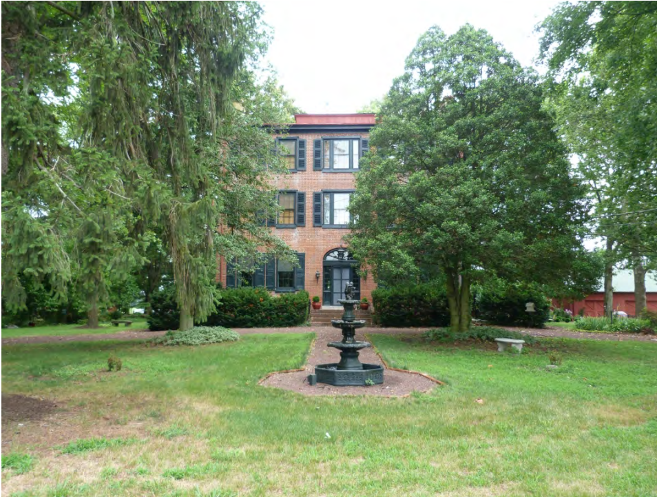
NJ_BURLINGTON_RIDGWAY, HOUSE, WILLIAM_0006
