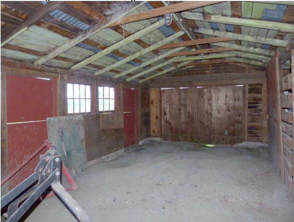
NJ_BURLINGTON_RIDGWAY, HOUSE, WILLIAM_0055
