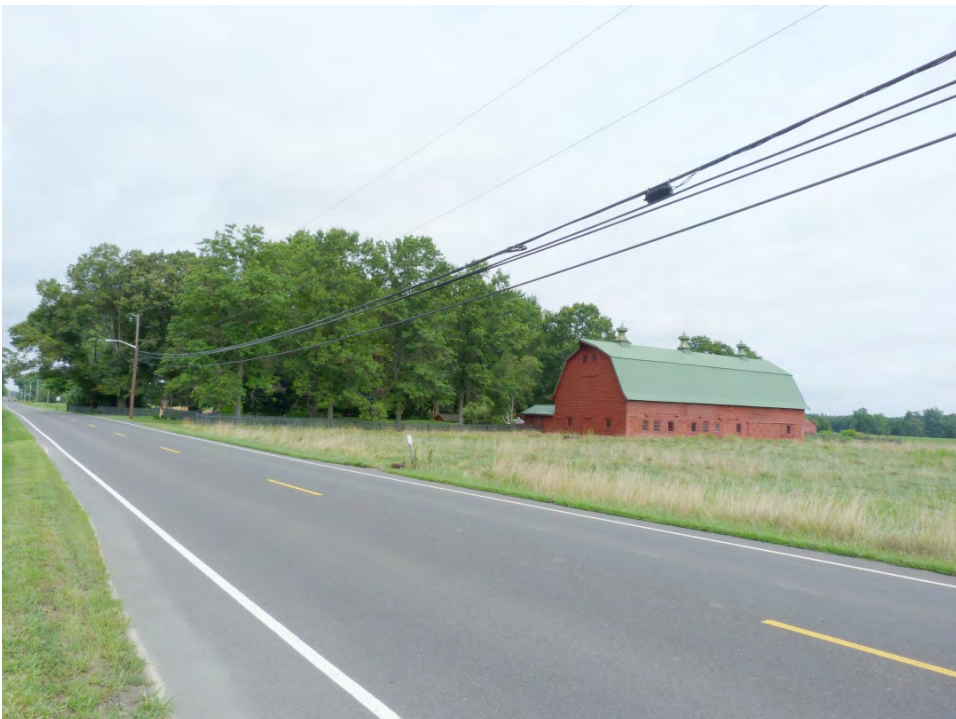
NJ_BURLINGTON_RIDGWAY, HOUSE, WILLIAM_0003
