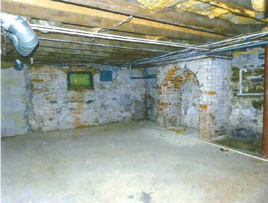
NJ_BURLINGTON_RIDGWAY, HOUSE, WILLIAM_0046
