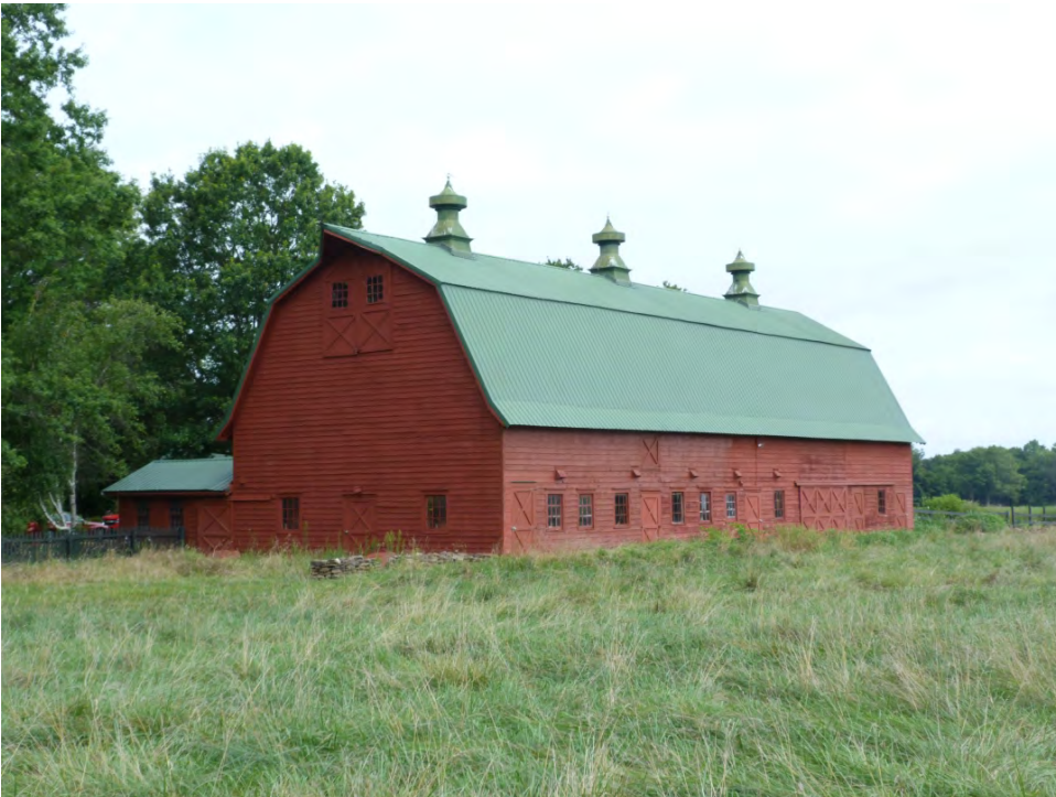
NJ_BURLINGTON_RIDGWAY, HOUSE, WILLIAM_0009
