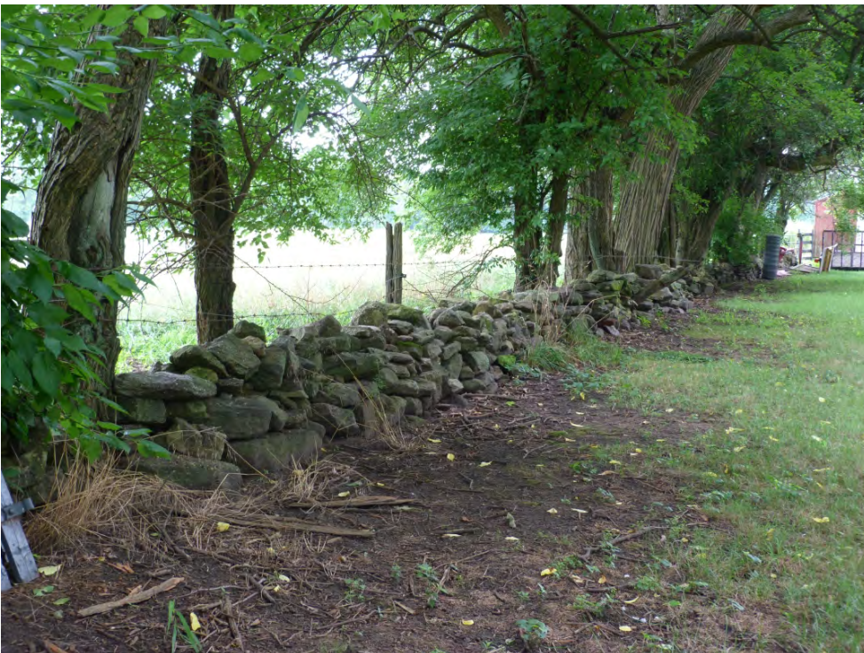
NJ_BURLINGTON_RIDGWAY, HOUSE, WILLIAM_0005
