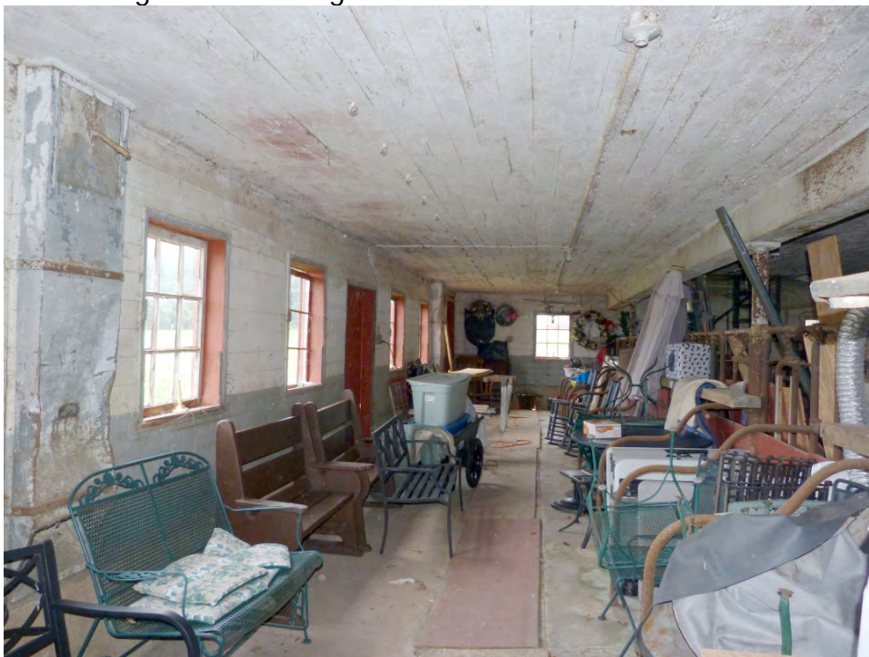
NJ_BURLINGTON_RIDGWAY, HOUSE, WILLIAM_0049 View facing north in the first floor of the barn on the east side.
