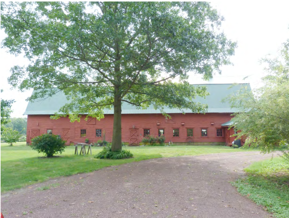
NJ_BURLINGTON_RIDGWAY, HOUSE, WILLIAM_0047
