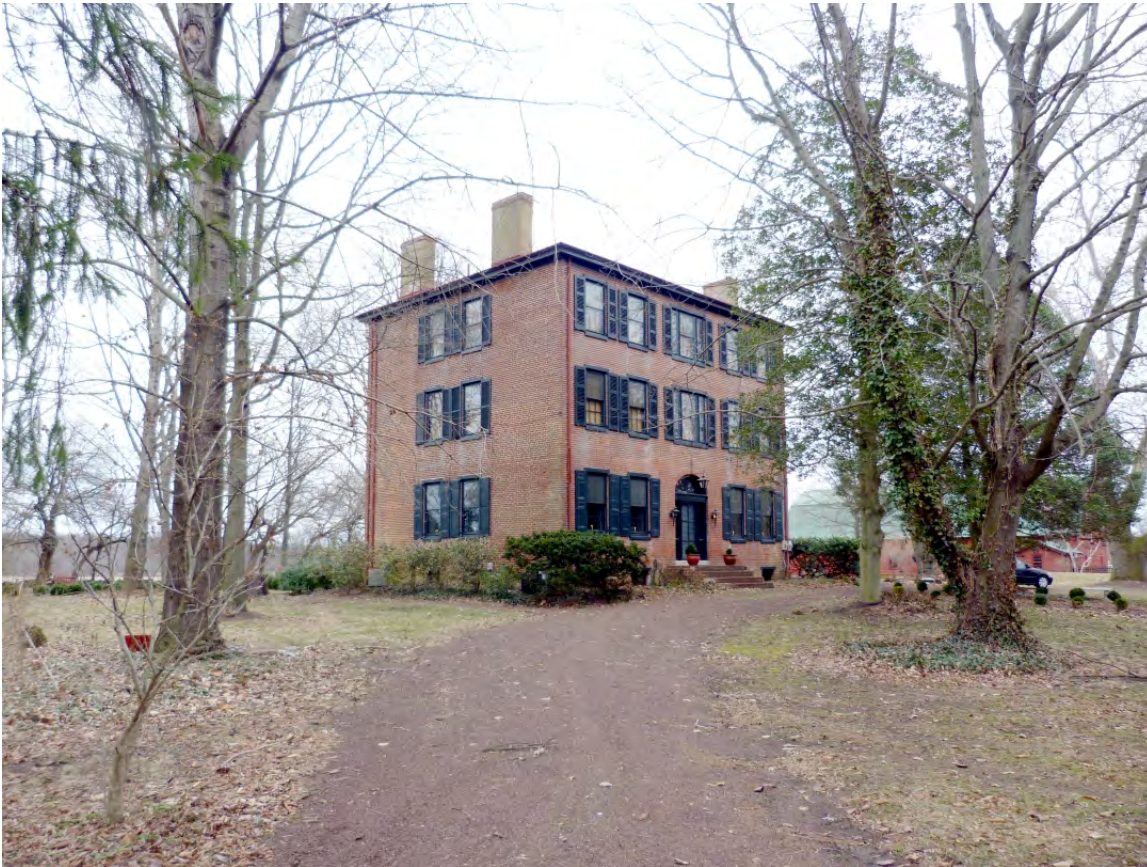
NJ_BURLINGTON_RIDGWAY, HOUSE, WILLIAM_0001
