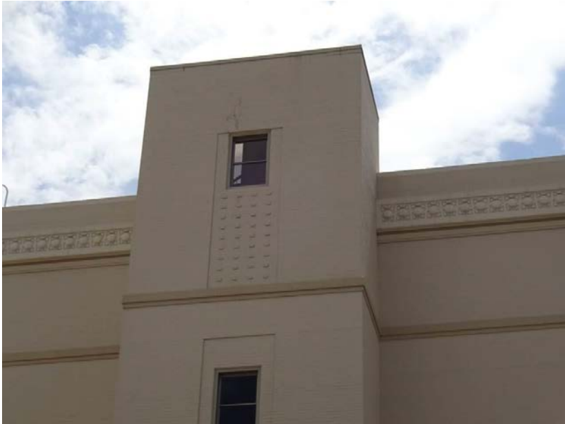
Photo 18 West elevation, fifth floor detail
