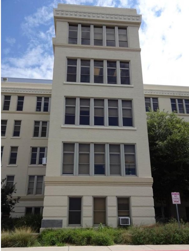
Photo 5 Central portion, south elevation west wing looking
