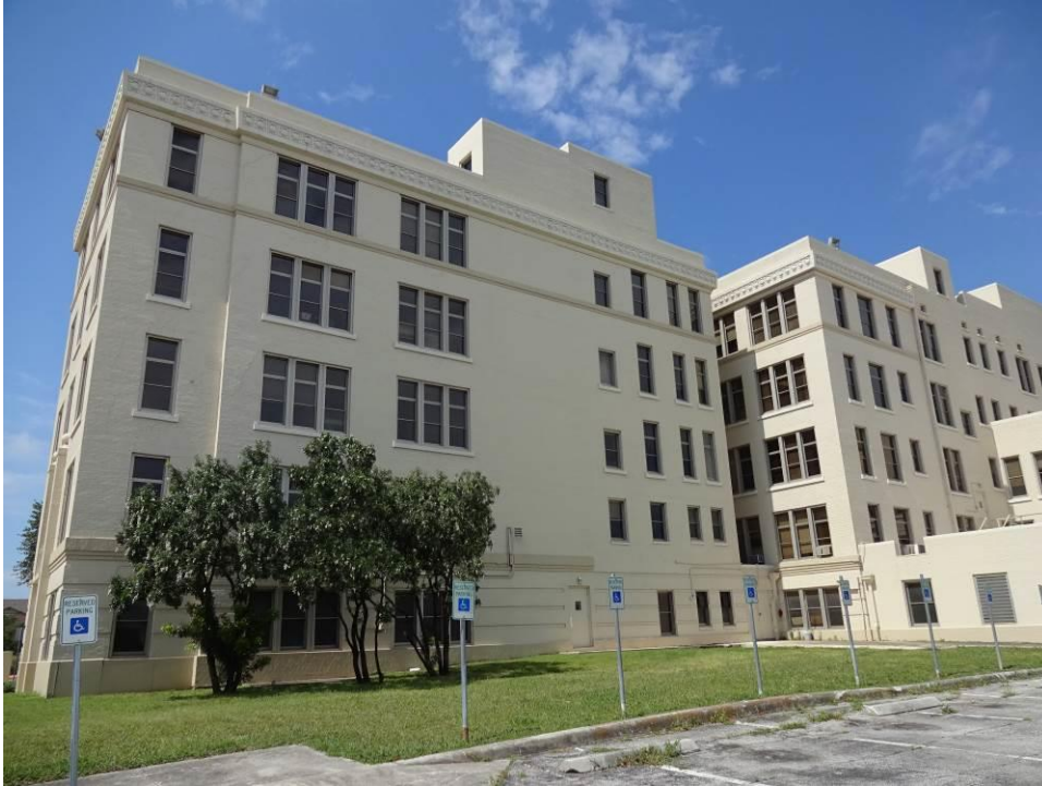
Photo 11 East annex, north elevation looking south
