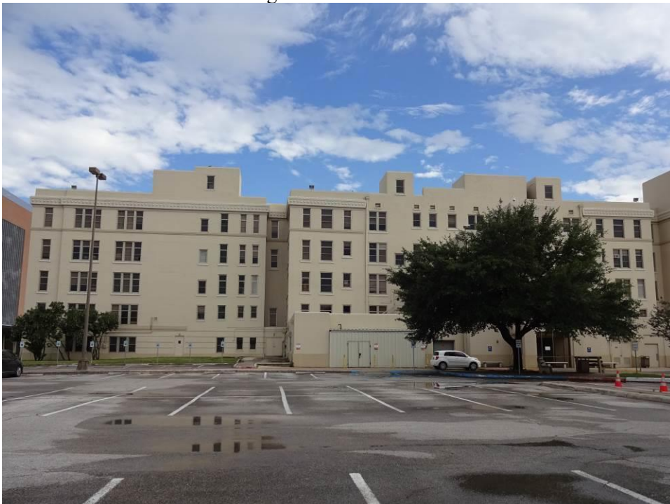
Photo 12 North elevation full view looking south
