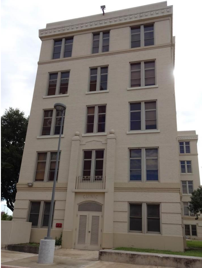
Photo 9 East elevation looking west
