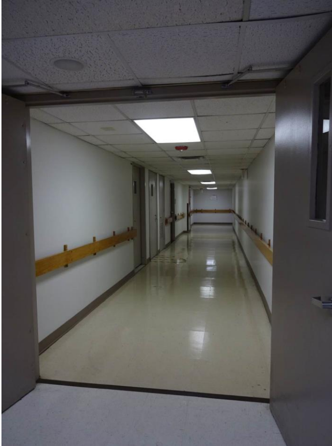
Photo 28 Interior, first floor hallway looking east
