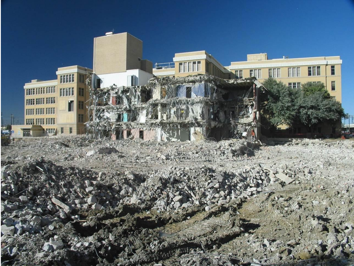
Figure 16 Demolition of Brady-Green Clinic, 2013
