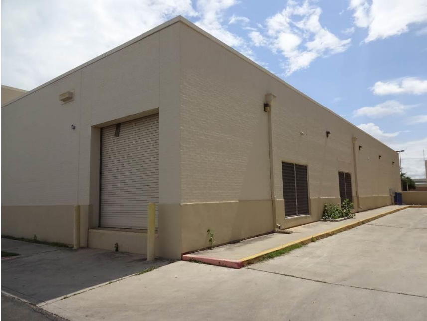
Power plant, south elevation looking east
