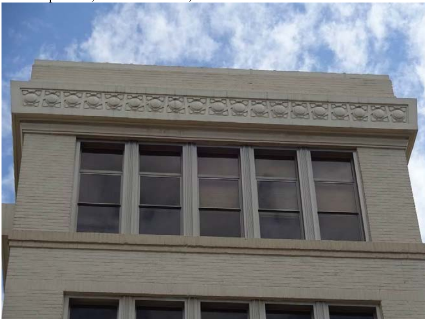
Photo 6 Central portion, south elevation, cornice detail
