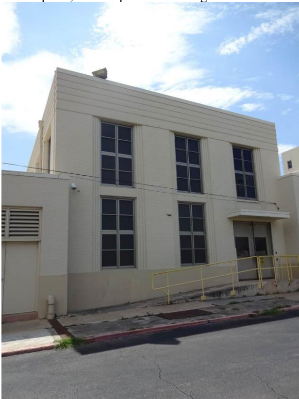
Power plant, central portion looking east
