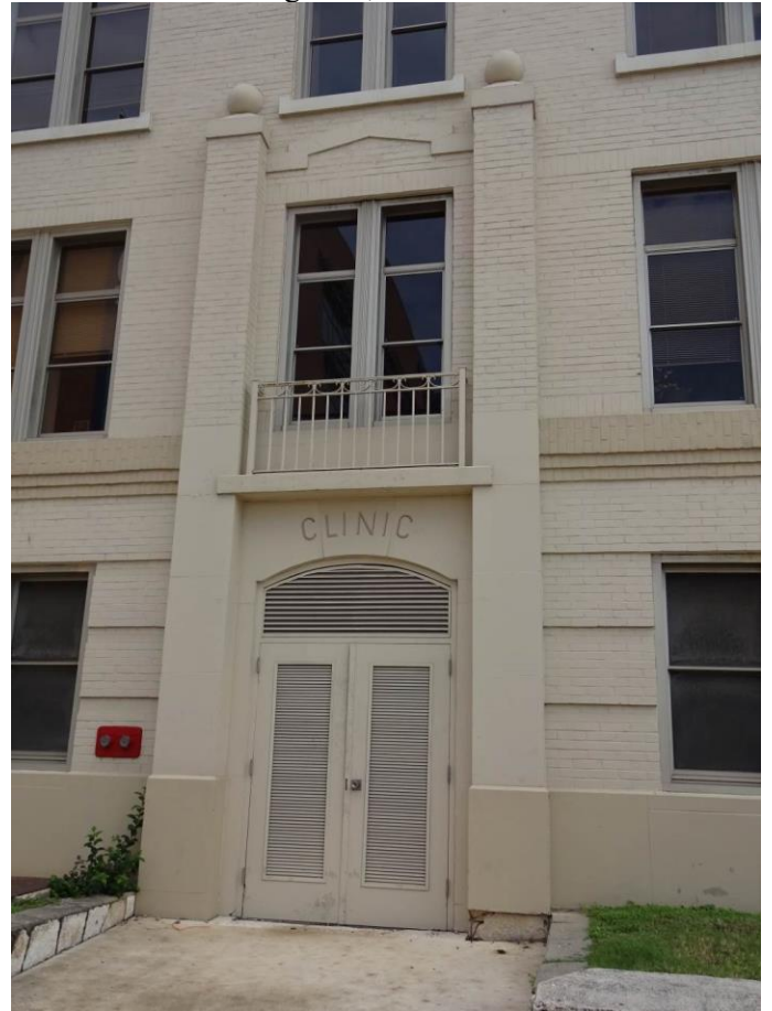
Photo 10 East elevation looking west, entrance detail
