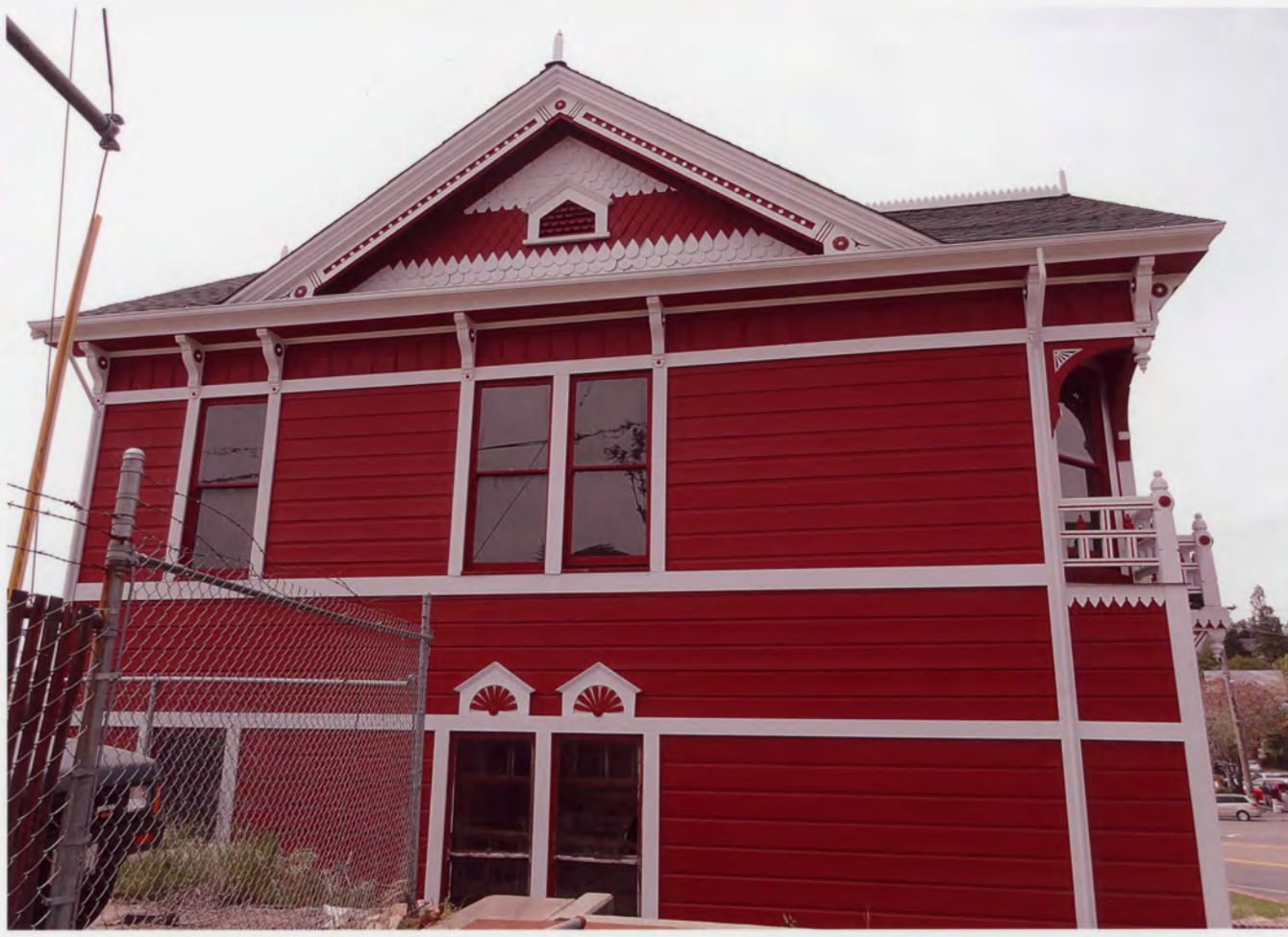
3. AUBURN FIREHOUSE NO. 1 PLACER COUNTY, CA
