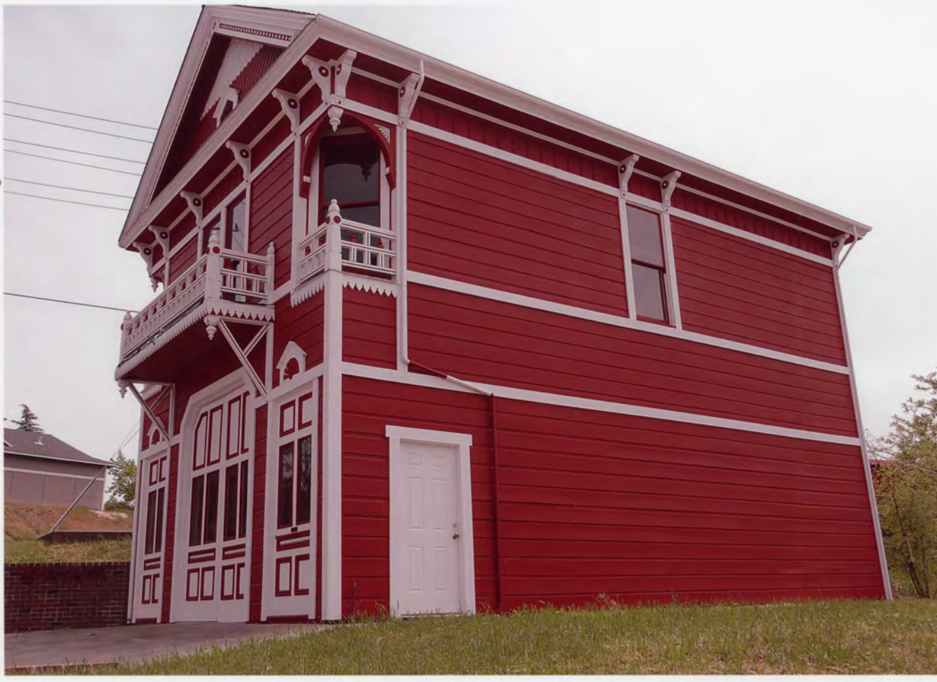
2. AUBURN FIREHOUSE NO. 1 PLACER COUNTY, CA
