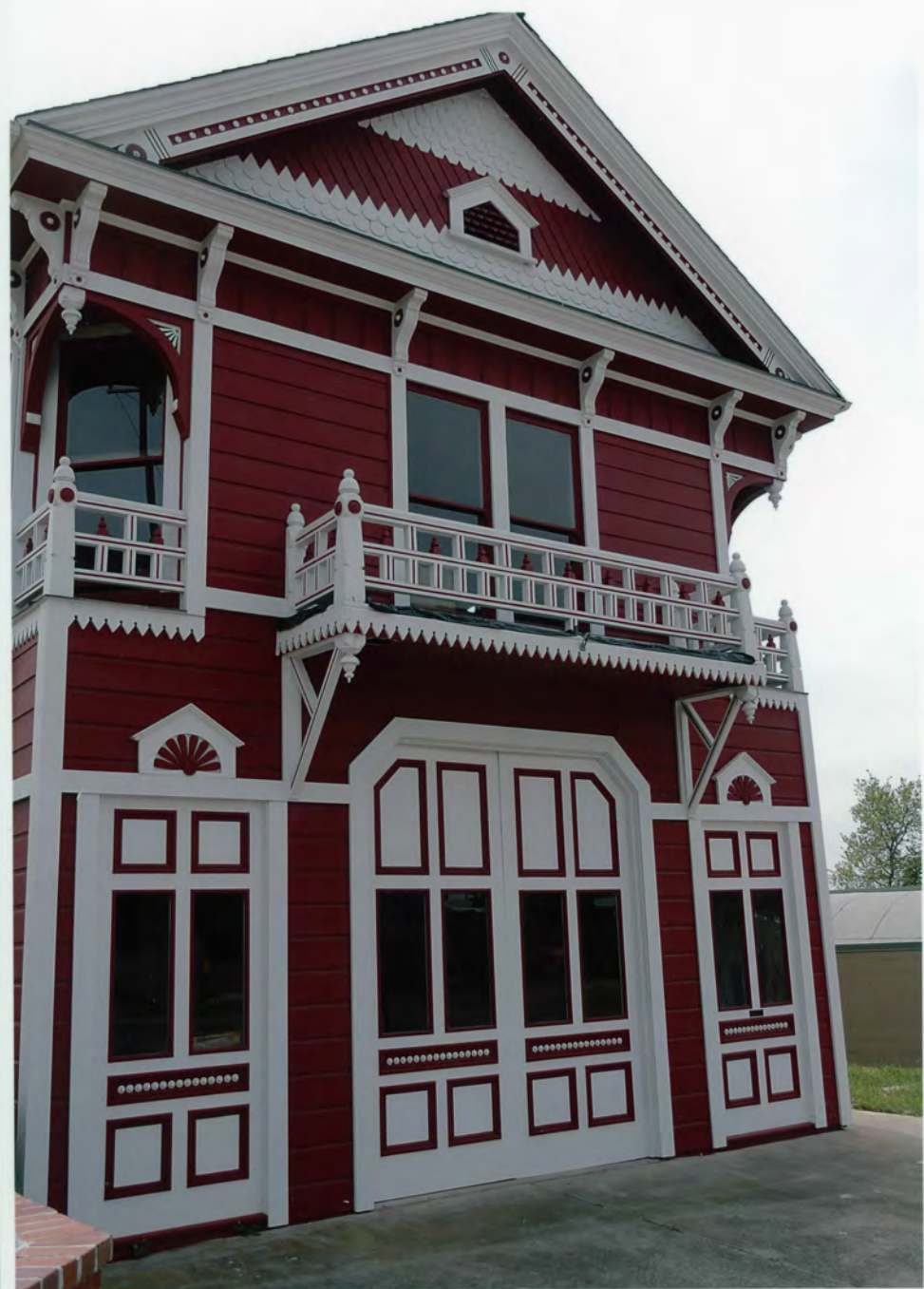
1. AUBURN FIREHOUSE NO. 1 PLACER COUNTY, CA
