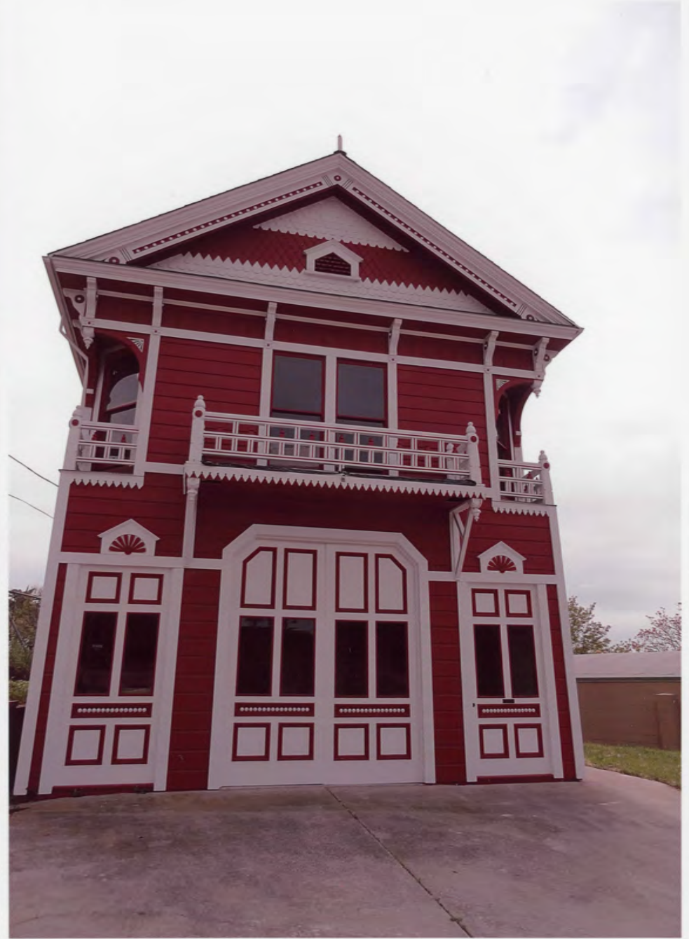
5. AUBURN FIREHOUSE NO. 1 PLACER COUNTY, CA
