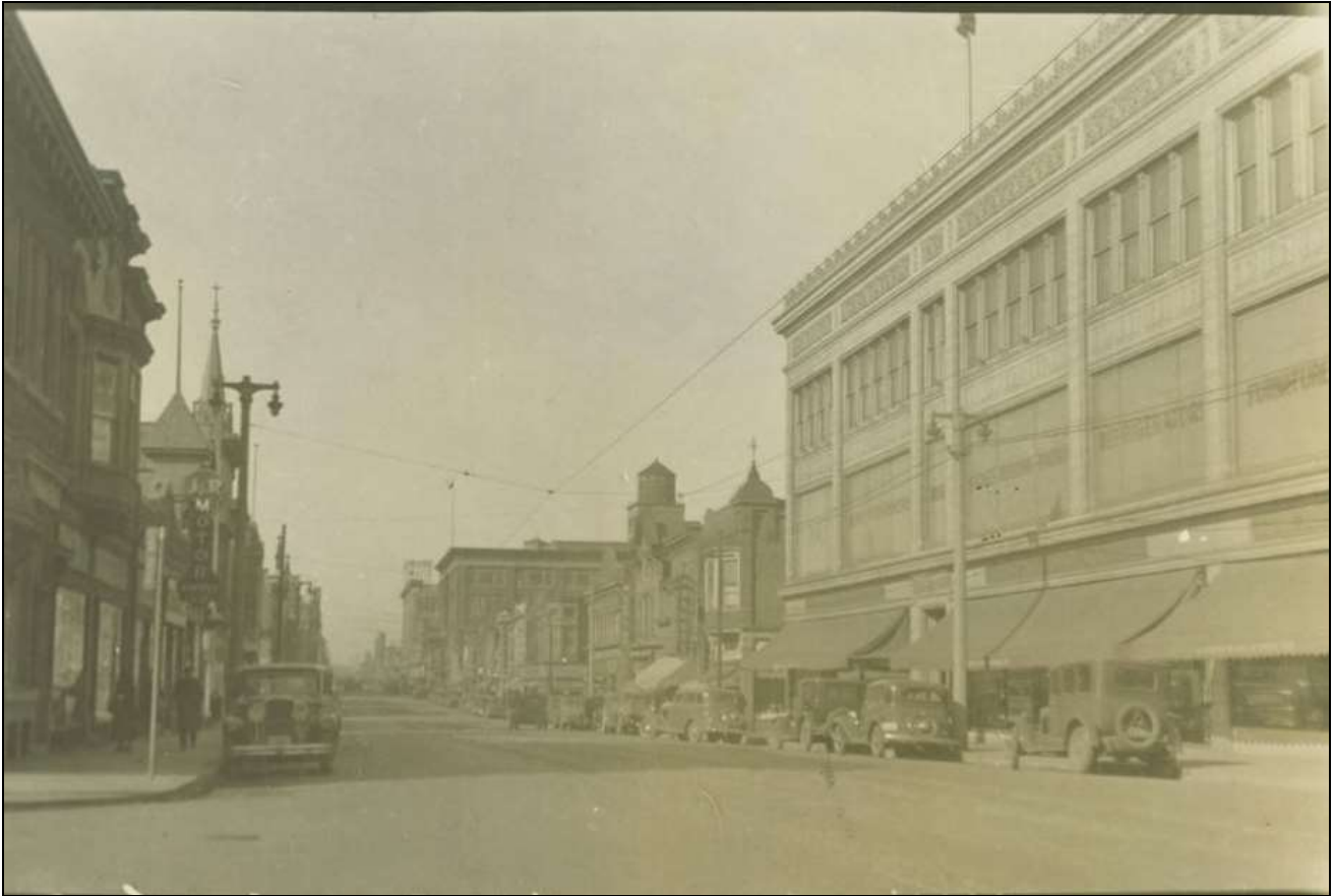
Figure 1: W. Mitchell Street looking west from S. 7 th Street (1934); Kunzelmann-Esser Furniture, 710 W. Mitchell Street, at right.
