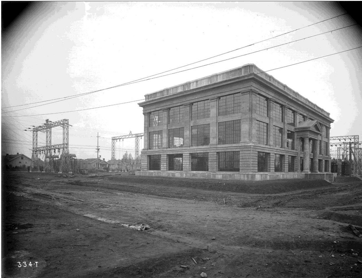
Figure 2. Cushman Substation, 1925, southwest oblique (viewing northeast) with view to switchyard. Image courtesy of Tacoma Power.
