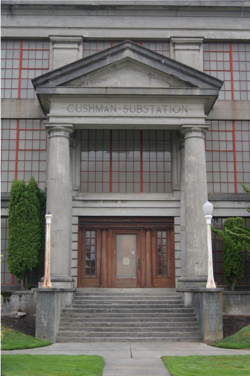
Photo 2 of 17. WA_PierceCounty_CushmanSubstation_0002. View of the temple front entrance on the façade (south face) of Cushman Substation.
