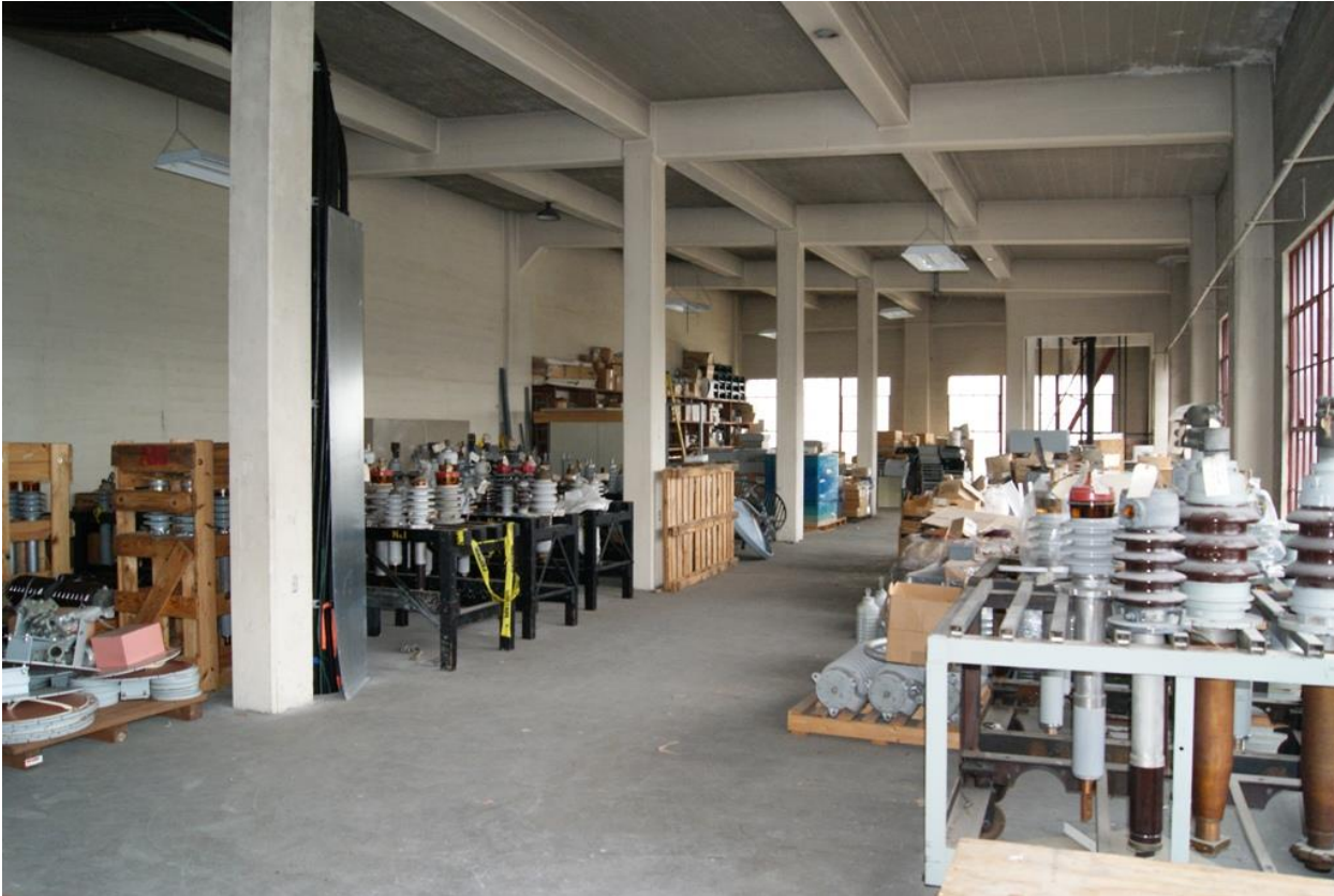
Photo 12 of 17. WA_PierceCounty_CushmanSubstation_0012. Second floor room at Cushman Substation, now used for storage.
