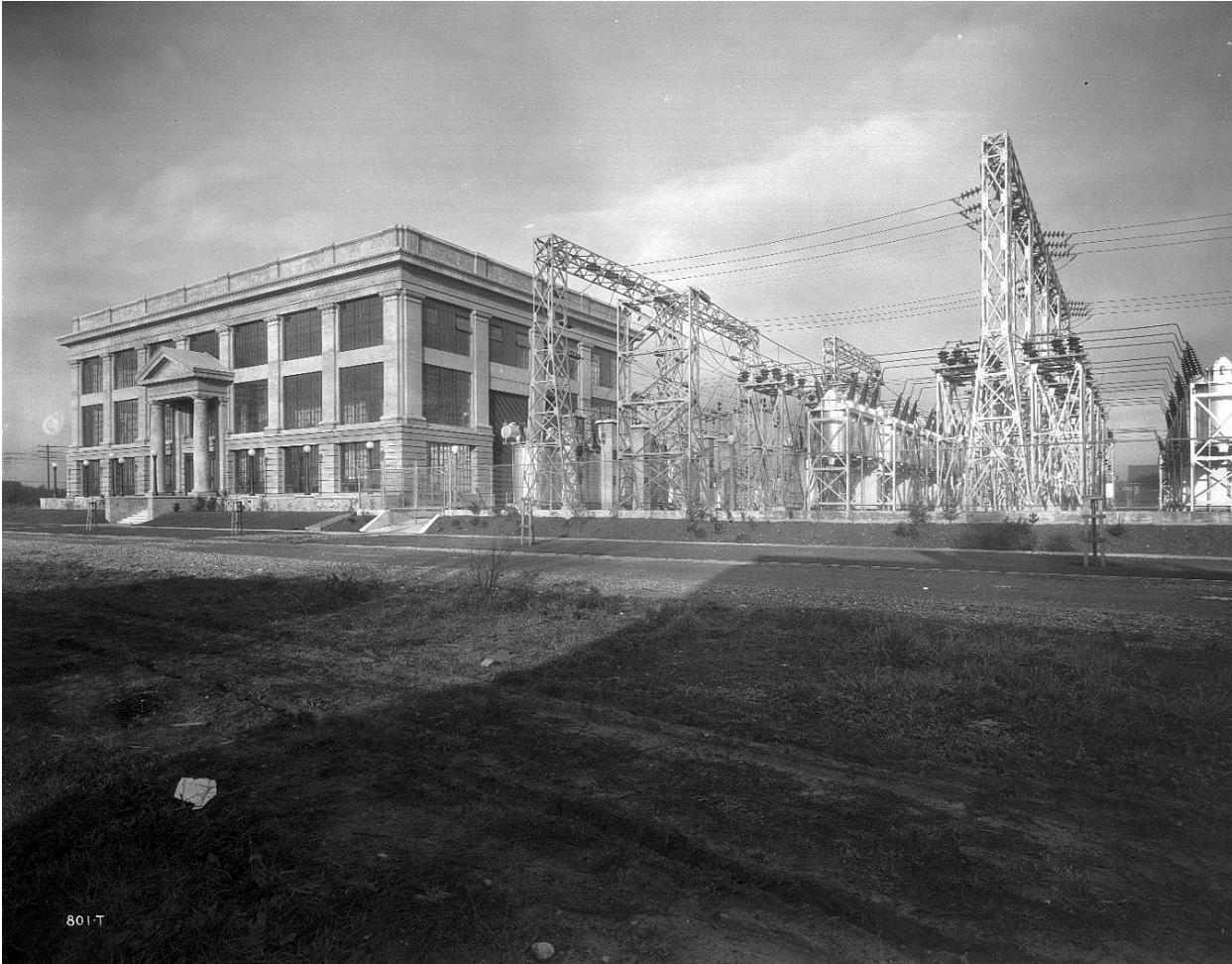
Figure 3. Cushman Substation, 1925, southeast oblique (viewing northwest) with view of switchyard (no longer extant). Image courtesy of Tacoma Power.
