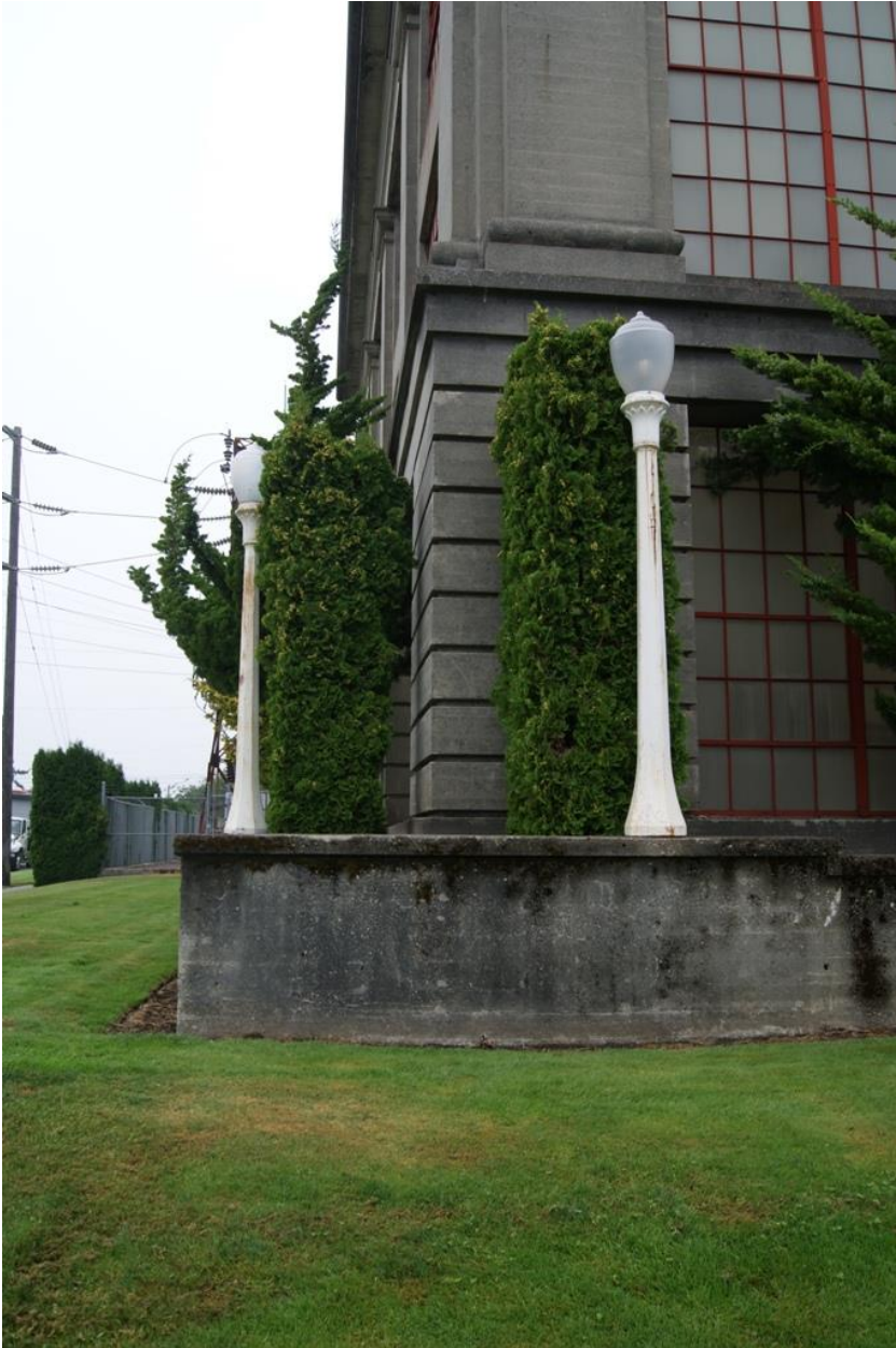
Photo 8 of 17. WA_PierceCounty_CushmanSubstation_0008. Detail of the original cast concrete lamp posts located on the northwest corner of Cushman Substation. The globes are modern plastic.
