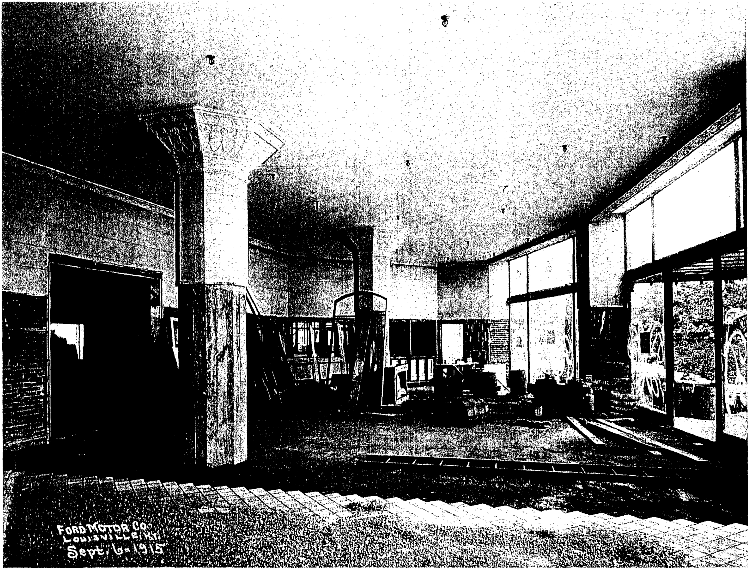
Figure 3: Photo of showroom during construction. Note: capitals and tile floors are extant but currently covered. Ford Motor Company Archives.
