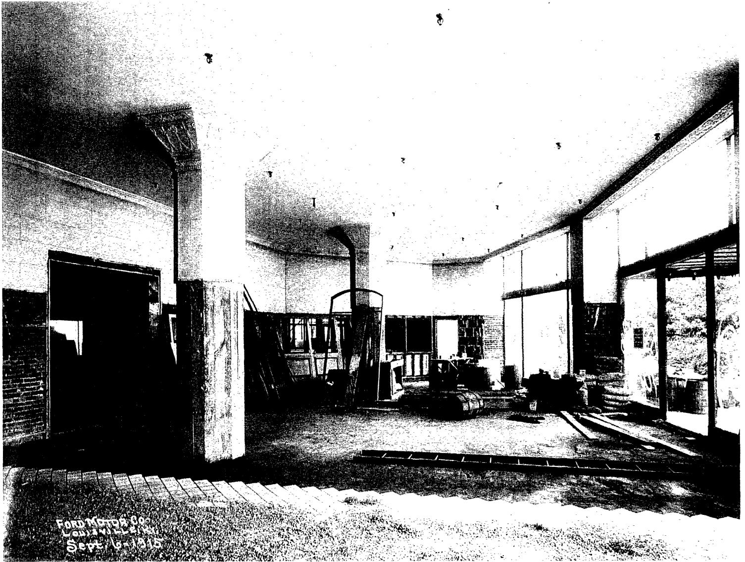
Figure 3: Photo of showroom during construction. Note: capitals and tile floors are extant but currently covered. Ford Motor Company Archives.
