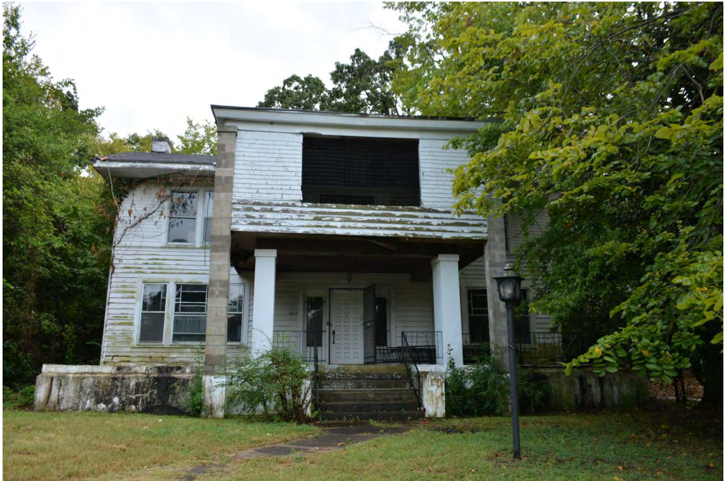
Property at 2623 West Markham – 2016. From the files of the Arkansas Historic Preservation Program.
