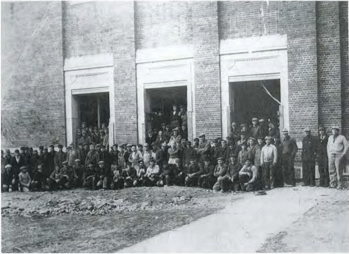
Figure 5: WPA workers in front of auditorium addition, taken in 1938 Brown County Historical Society
