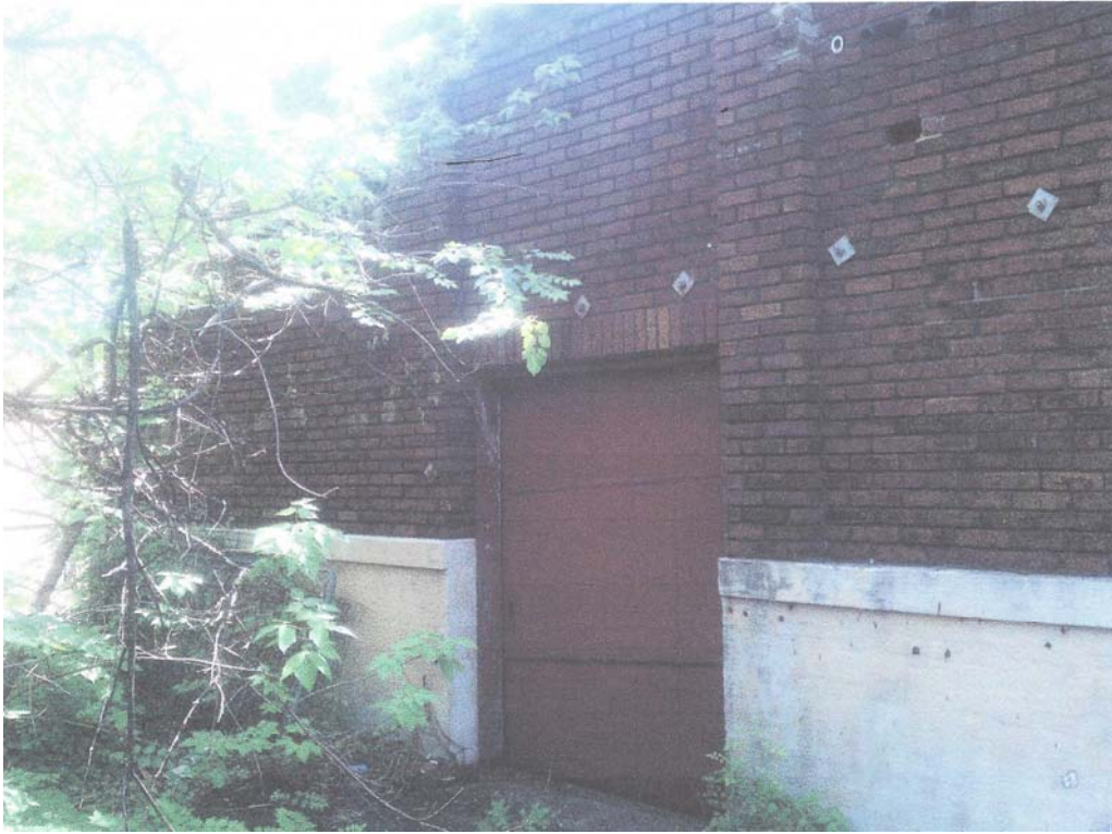
East (Back) Elevation: June 2014 Source: Owner
