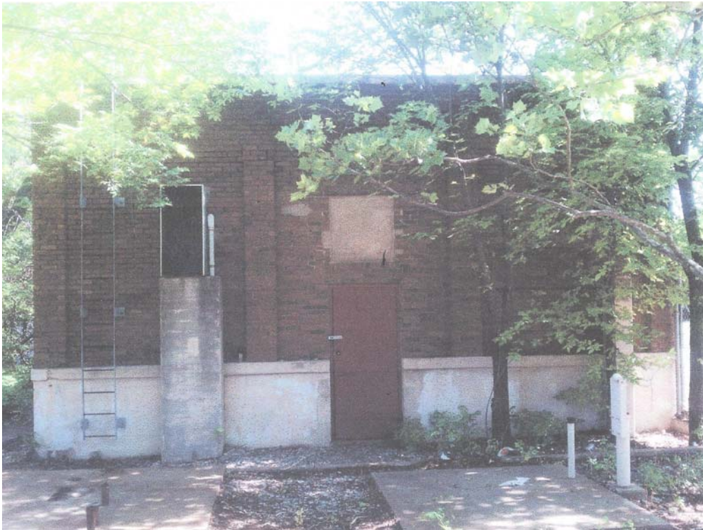
North Side Elevation: June 2014 Source: Owner
