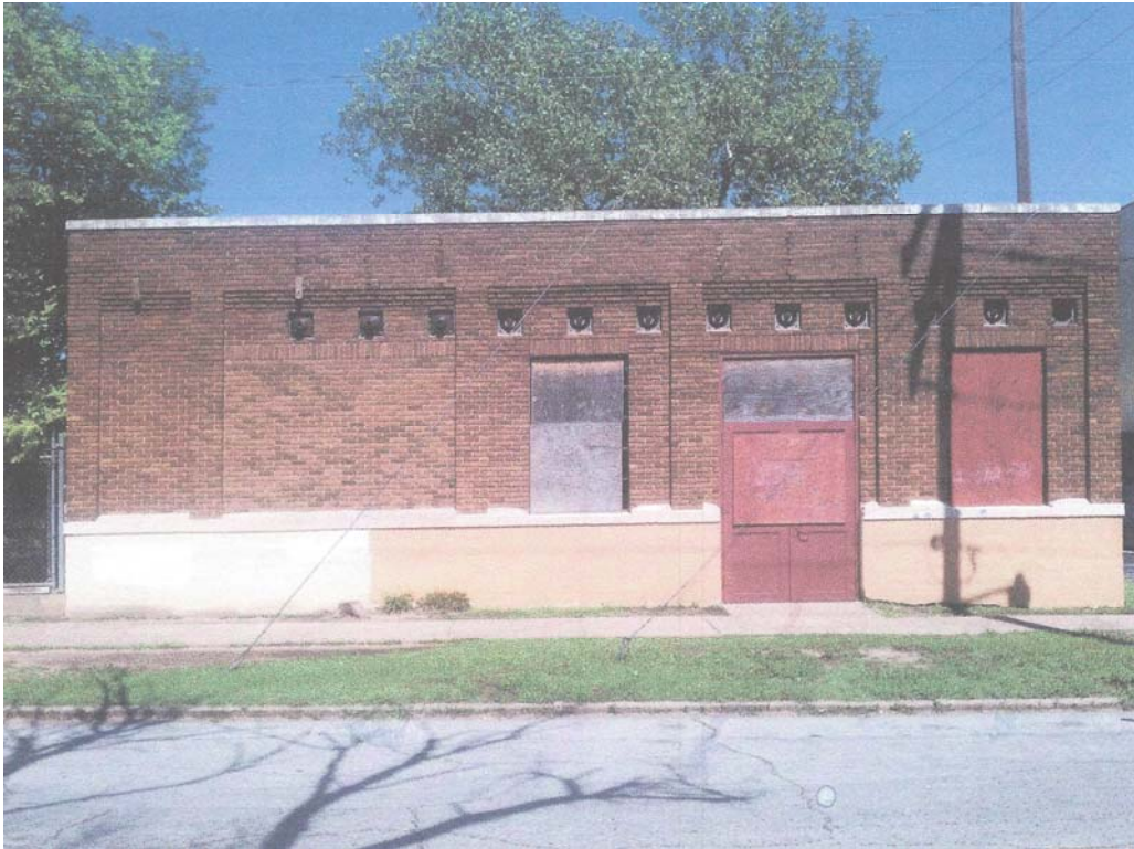
West Facing Façade: June 2014 Source: Owner
